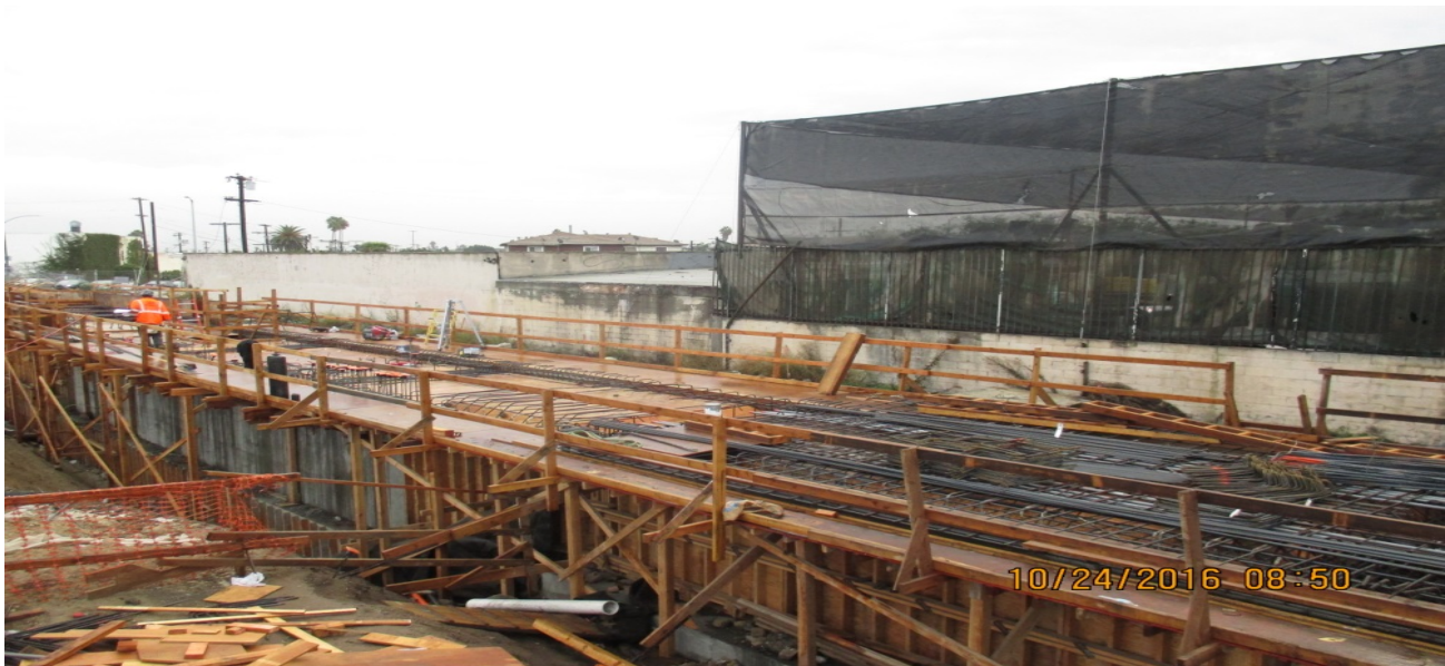
FAIRVIEW HEIGHTS STATION – Crews continued with rebar and formwork installations for the platform deck and through-girders as well as deck MEP embeds.
