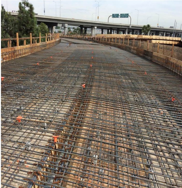
GREENLINE UNDERPASS – Deck rebar installation ongoing/girder-stem formwork installation ongoing.
