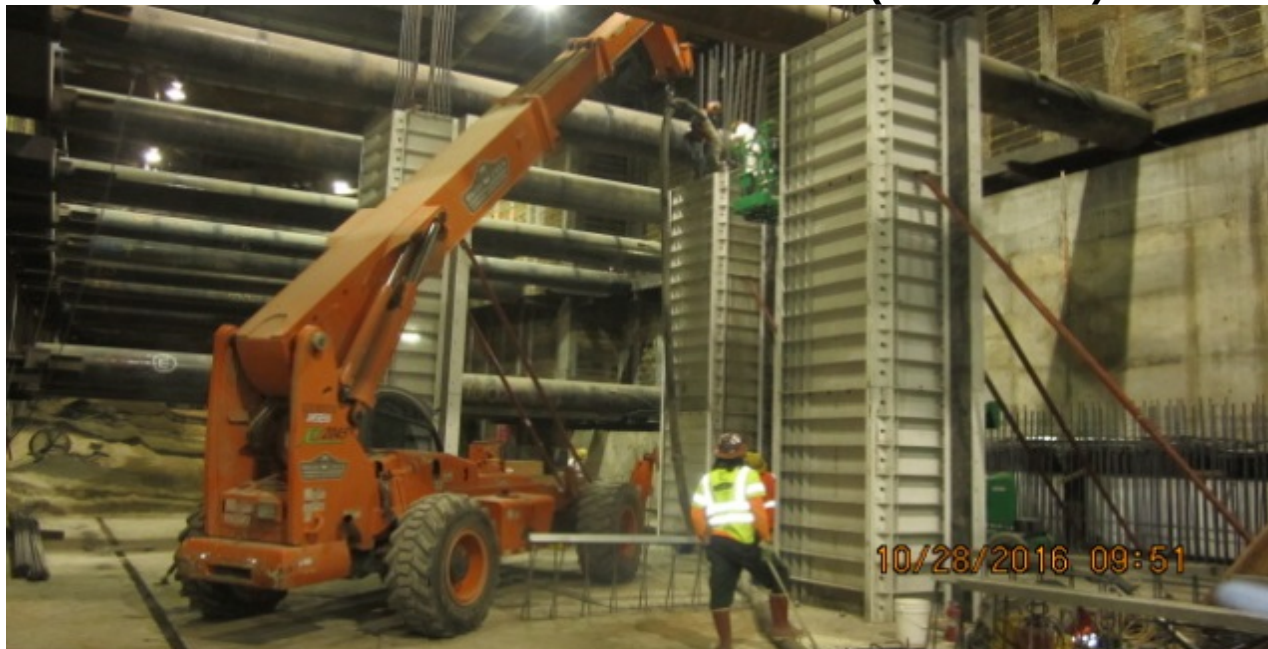
LEIMERT PARK STATION – Installation of invert column shear cap.
