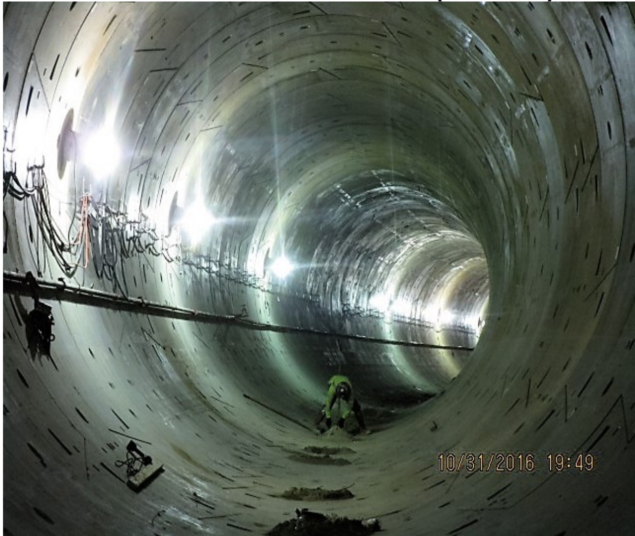
TUNNELING – Removed temporary rail and vent lines to prepare for invert pour of completed tunnel.
