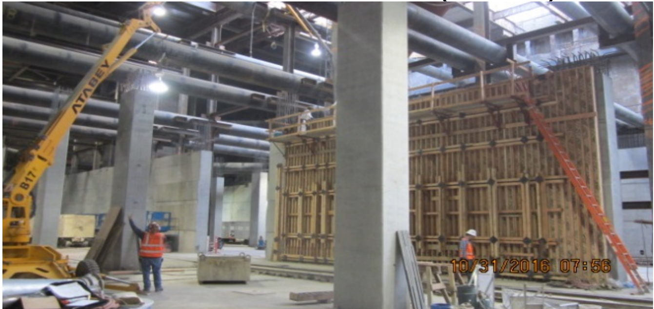
EXPOSITION/CRENSHAW STATION – Placing concrete for interior wall.
