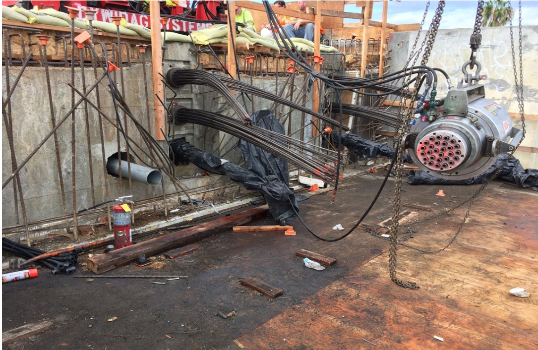
MANCHESTER BRIDGE – Bridge deck concrete placement complete. Subcontractor completed post tensioning stressing operations.
