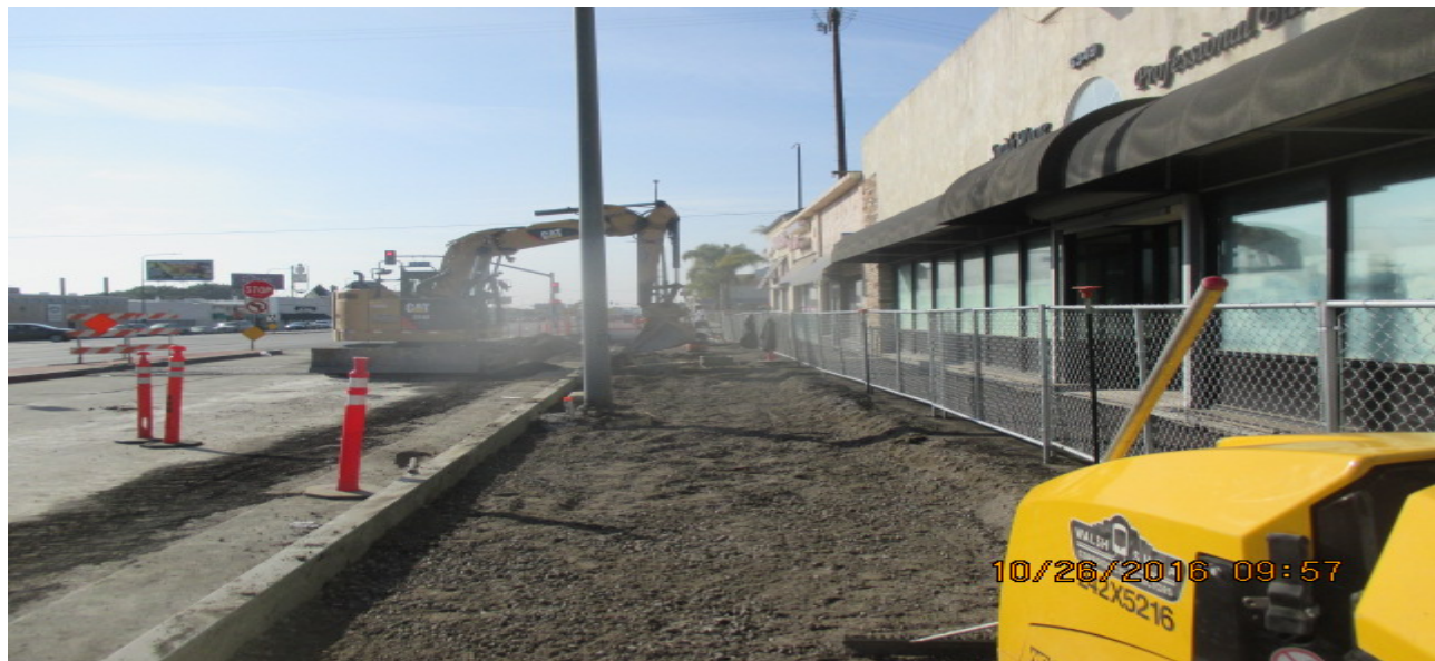
PARK MESA – Placing CMB base section north of 54 th .
