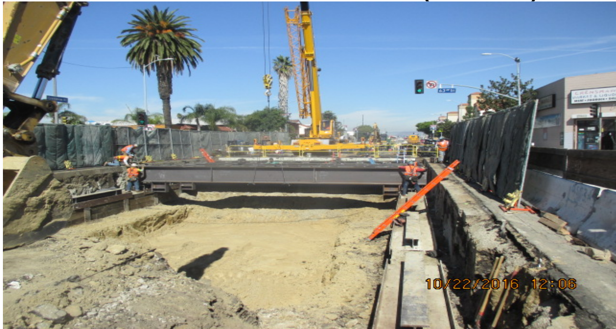
UG#3 – Completed placing deck beams and deck panels south of 63rd Street.
