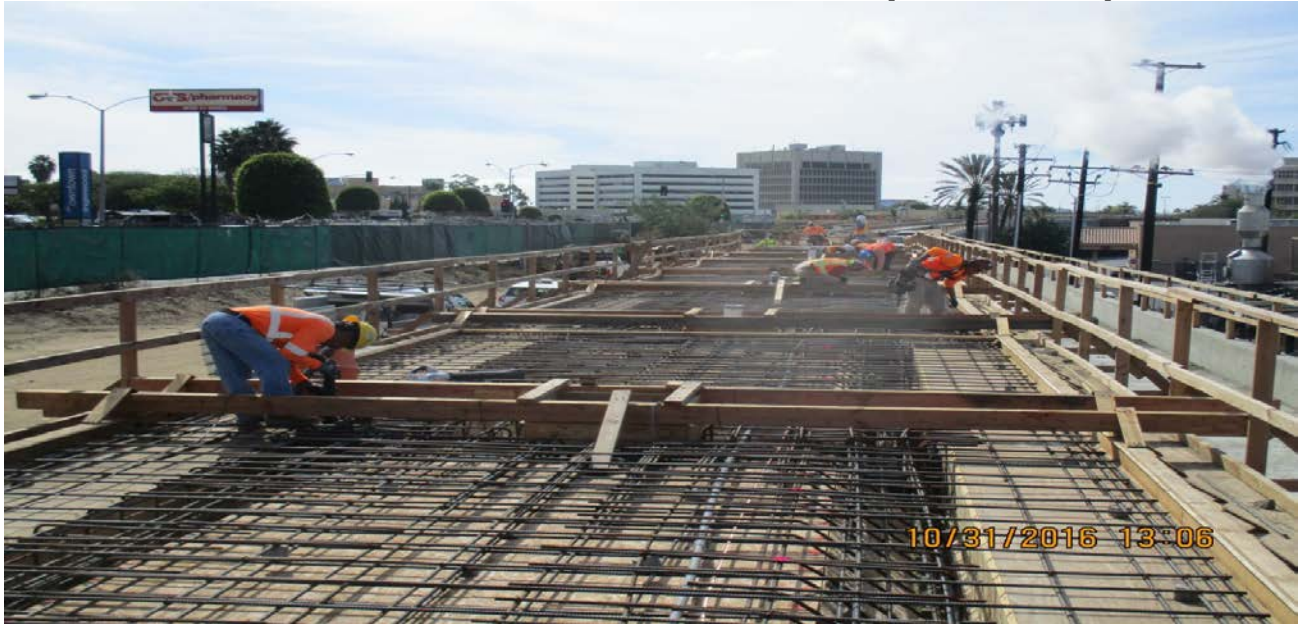
LA BREA BRIDGE -Crews prepped the platform deck and formed bulkheads for the upcoming concrete placements.
