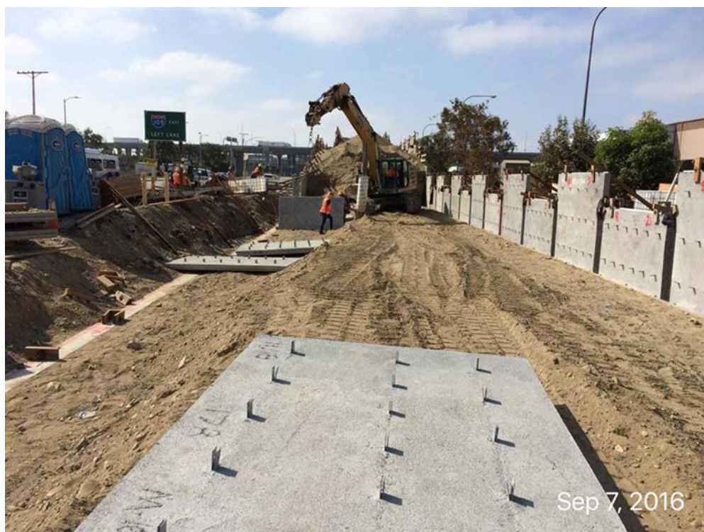
MSE WALL 17L & R (North of Imperial Hwy/I-105) – Continued with precast panel, erection, strap placement, backfill and compaction testing.
