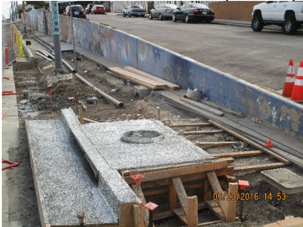
PARK MESA HEIGHTS – Placement of catch basin #25.
