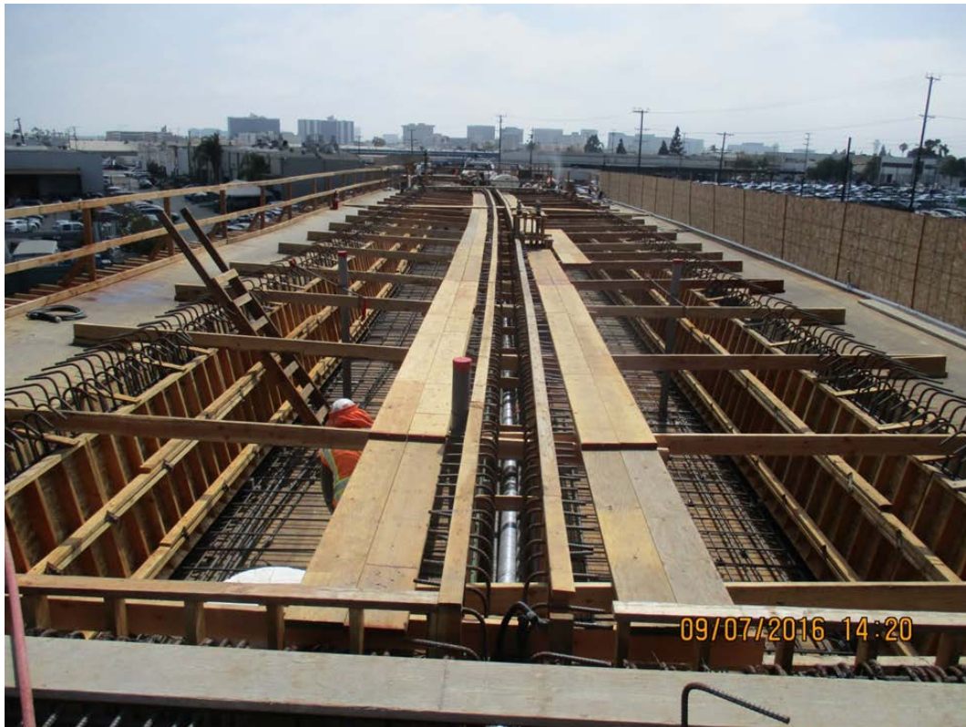
MANCHESTER BRIDGE – Finished formwork, placed and cured concrete for the stems and soffit.
