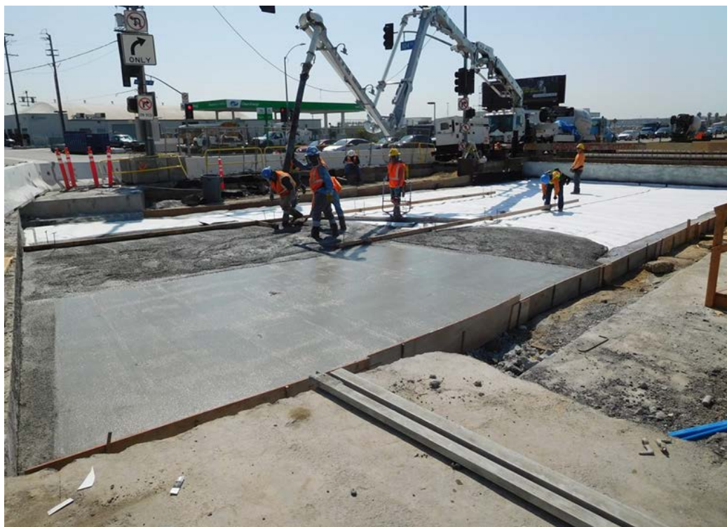
104 th STREET – Finished cut and cover tunnel including waterproofing protection slab and street restoration.
