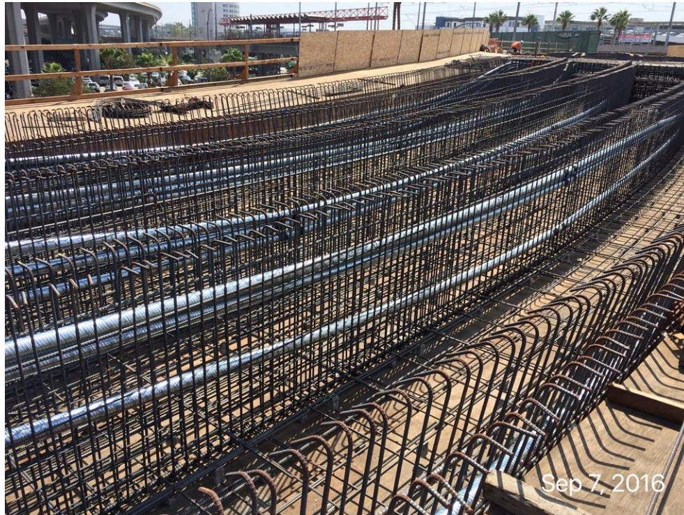
GREENLINE UNDERPASS – Post tensioning duct and girder stem/bent cap rebar installation Frame 1.
