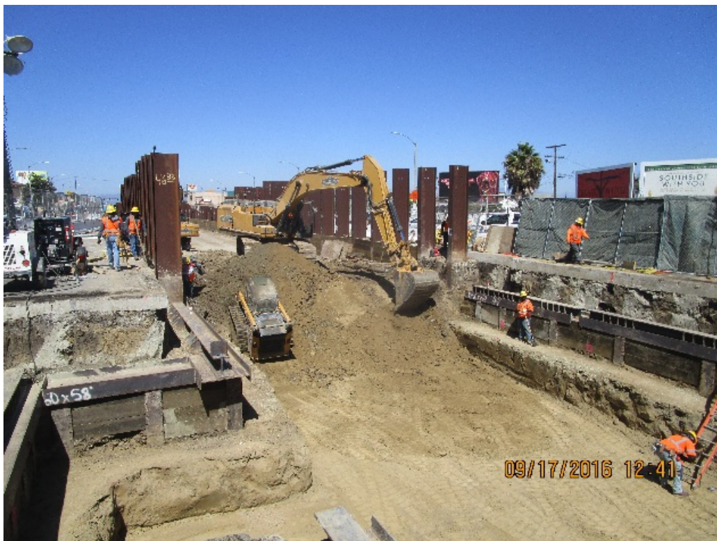
UG#3 – Excavation activities at north portal.
