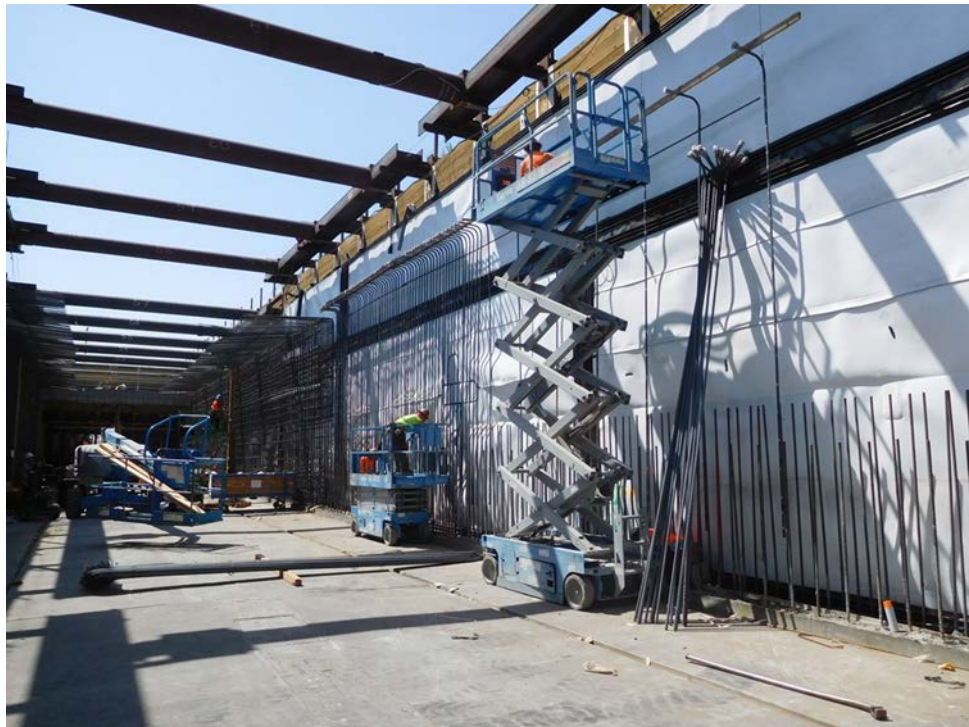
UG#1 – Type 2 strutted U-wall rebar installation.
