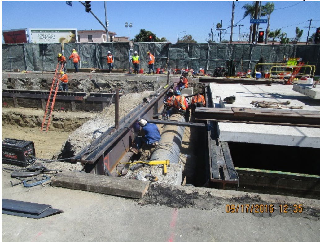
UG#3 – Setting deck beam and deck panels.
