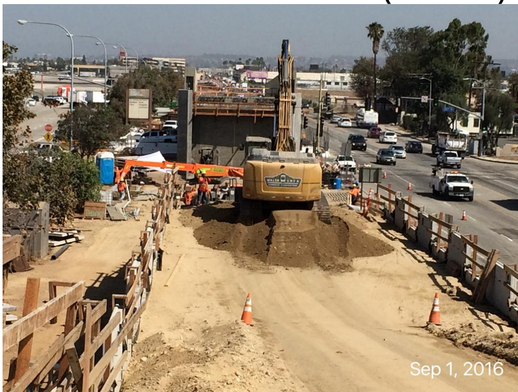
MSE WALL 17L & R (North of Imperial Hwy/I-105) – Continued with precast panel, erection, strap placement, backfill and compaction testing.
