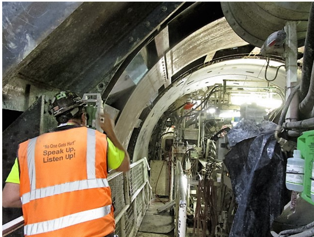
TUNNELING – Installation of ring #693.
