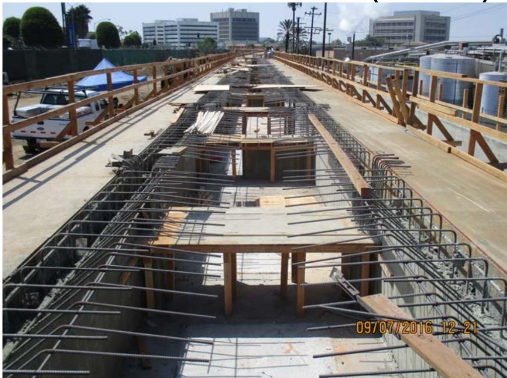
DOWNTOWN INGLEWOOD STATION – Deck formwork starts for the Downtown Inglewood Station platform.
