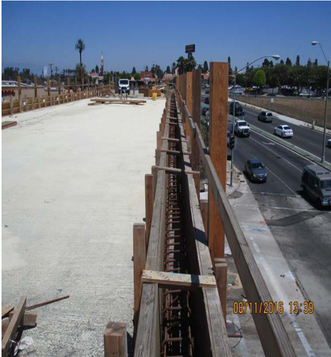
LA BREA BRIDGE – Worked on forming and concrete placement for the bridge deck parapet walls.
