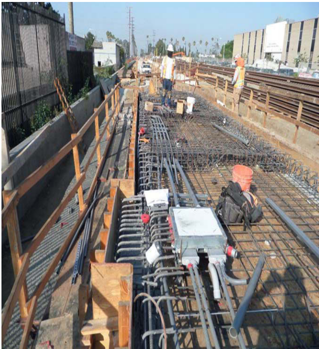
FAIRVIEW HEIGHTS STATION - Formwork installation and concrete placement for the subterranean TC&C room retaining walls.
