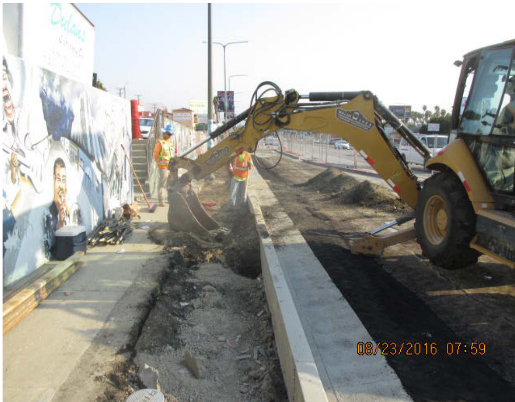
PARK MESA – Back fill activities behind installed curb and gutter at mural walls.
