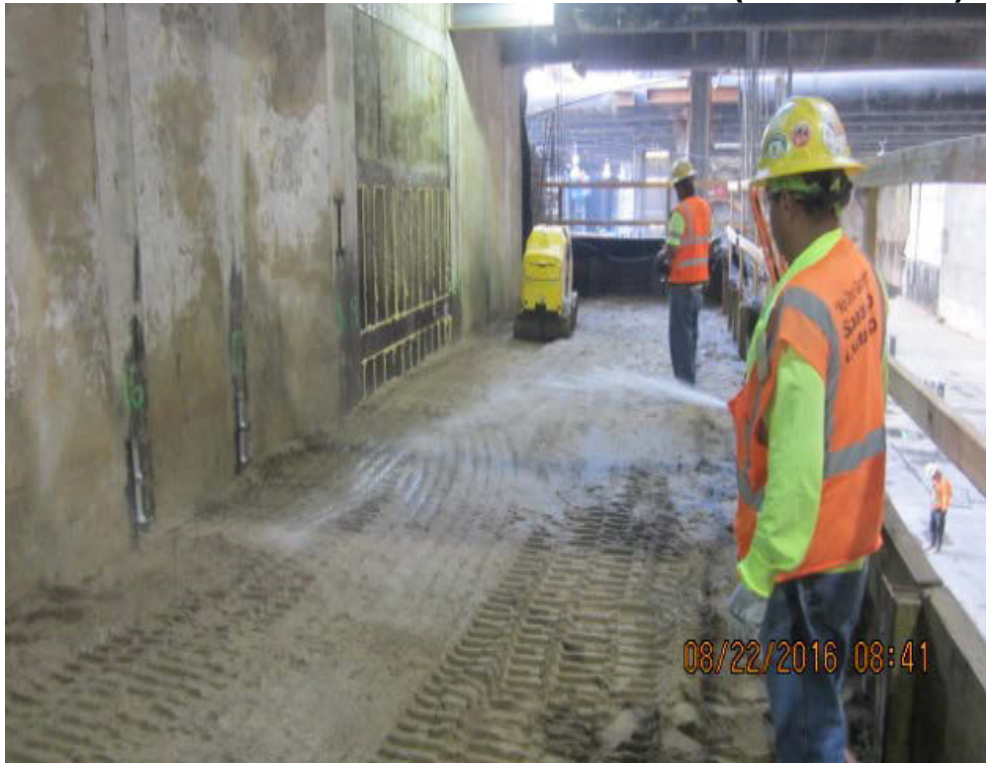
MARTIN LUTHER KING JR. STATION – Backfill and compaction activities at the south west bump out wall.
