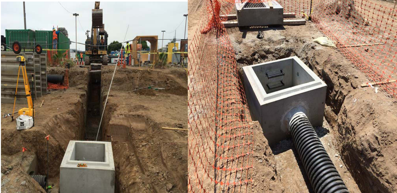
96 th STREET STATION ACCOMMODATIONS - Continued work on HDPE storm drain installations.
