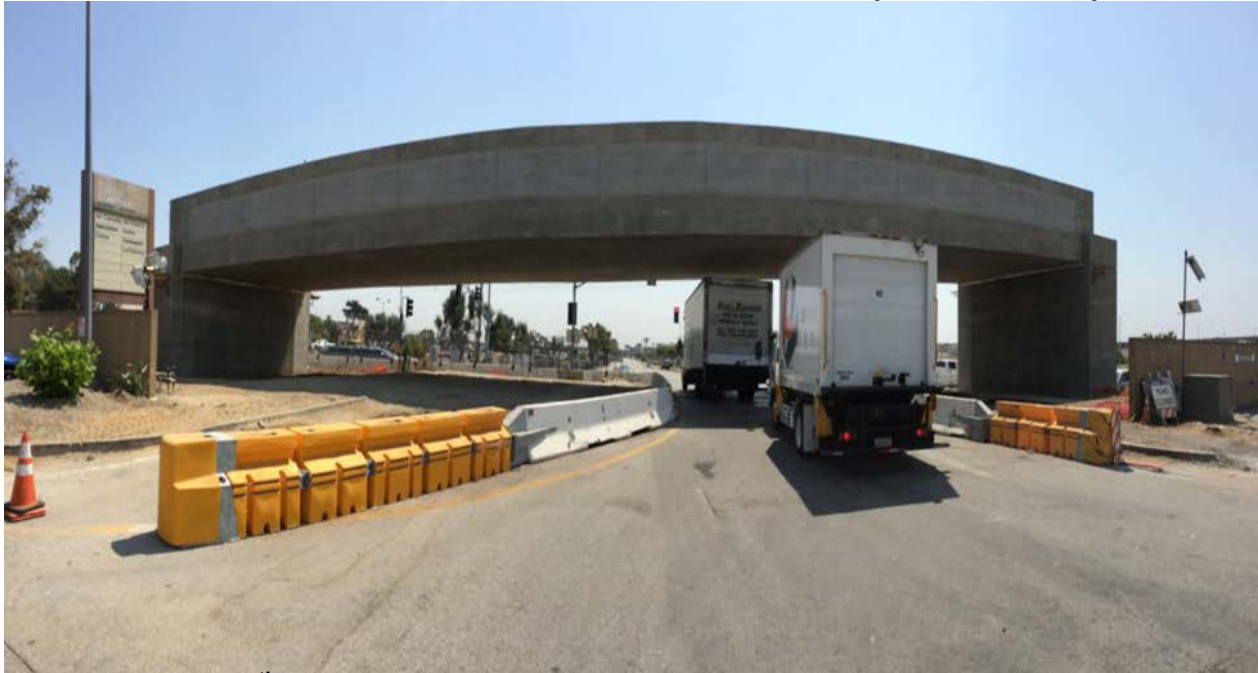
111 th STREET UNDERPASS - Panoramic view looking east.
