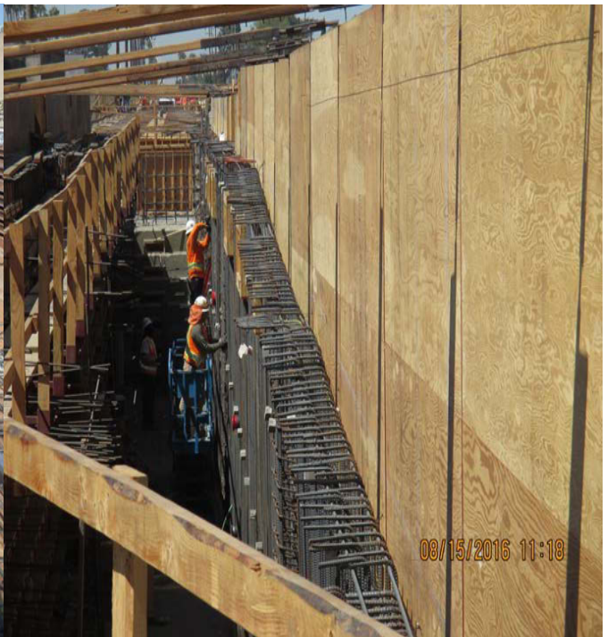
FAIRVIEW HEIGHTS STATION - Formwork installation and concrete placement for the subterranean TC&C room retaining walls.
