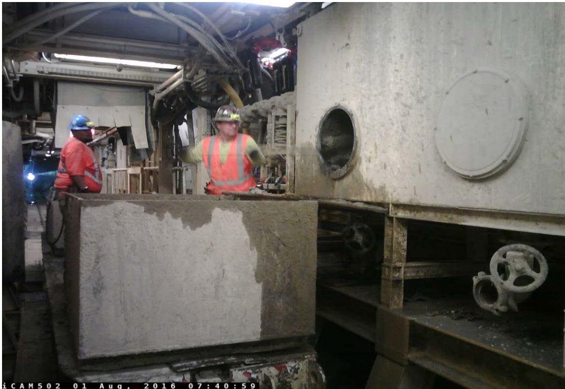
TUNNELING – Mucking out discharge tank.
