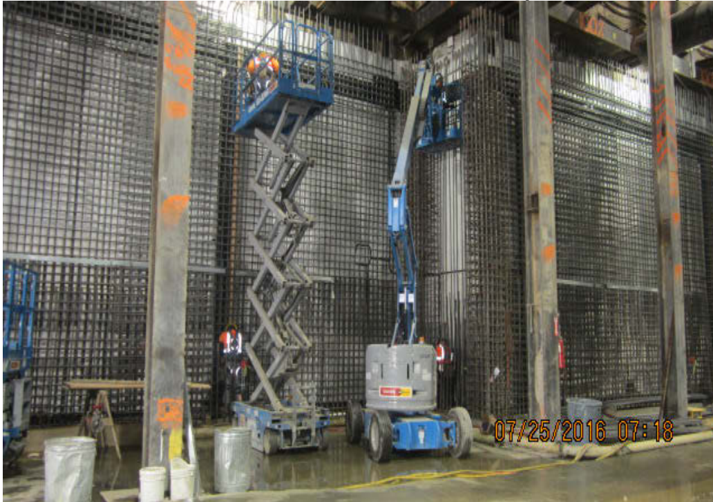
EXPOSITION/CRENSHAW STATION - Installation of rebar for east lower wall D-29 thru D-31.
