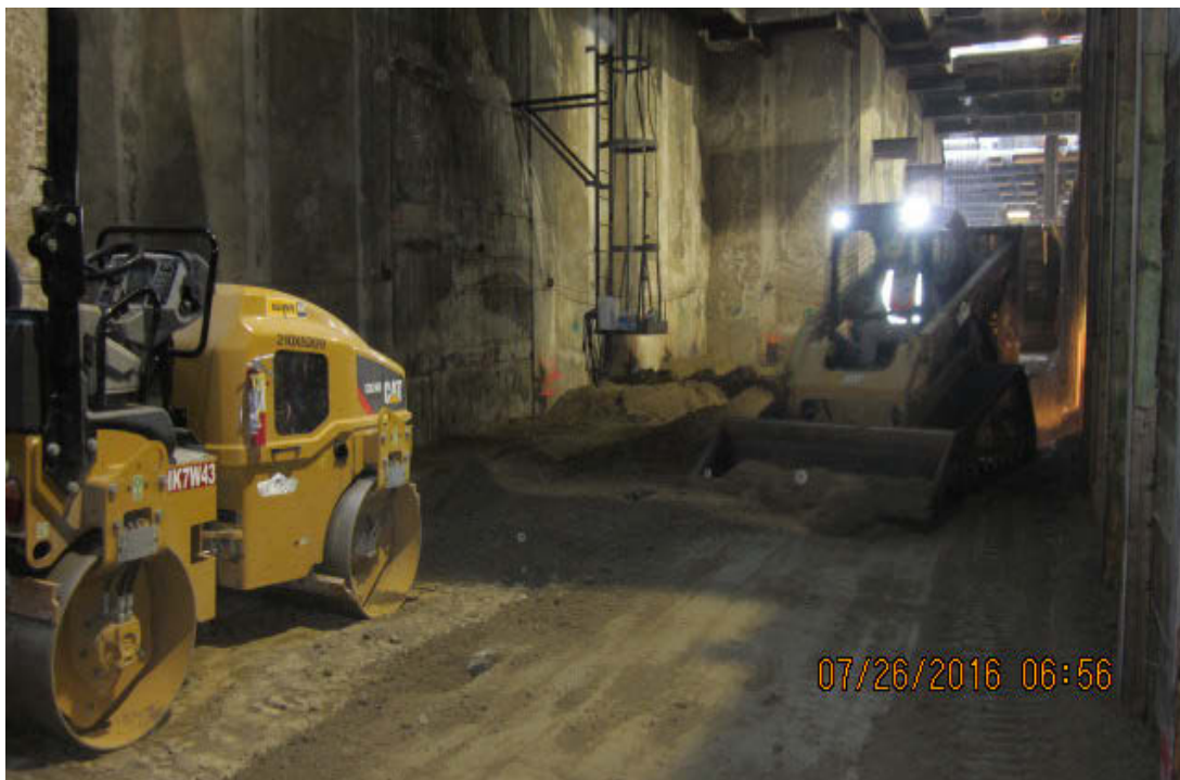
MARTIN LUTHER KING JR. STATION - Backfill and compaction of west bump out wall.
