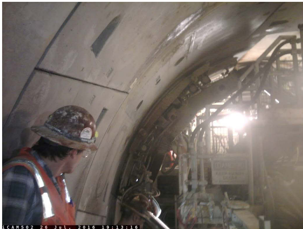
TUNNELING – Setting ring #519.
