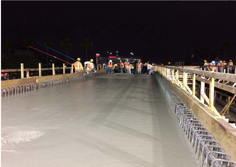
AVIATION/CENTURY BRIDGE – Frame 1A deck concrete placement.
