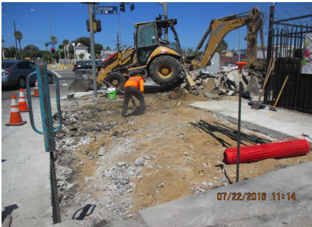
PARK MESA HEIGHTS - Demolition activities at sidewalk at 52 nd Street.
