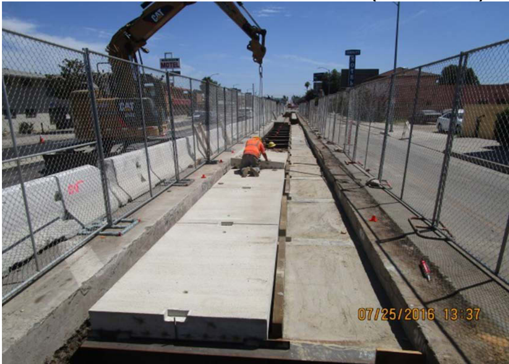
UG#3 – Installation of west side deck panels.
