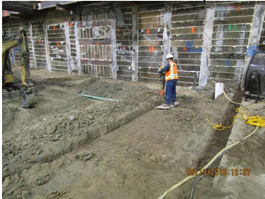
LEIMERT PARK STATION – Installation of grounding grid in preparation for mudslab placement.
