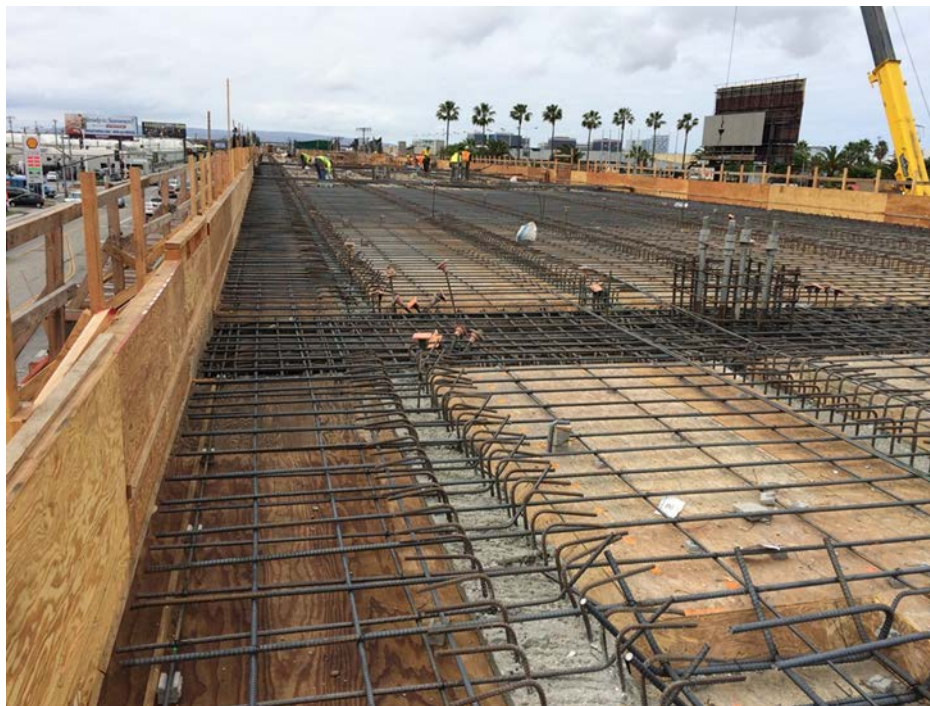
AVIATION/CENTURY BRIDGE – Frame 1 deck rebar installation.
