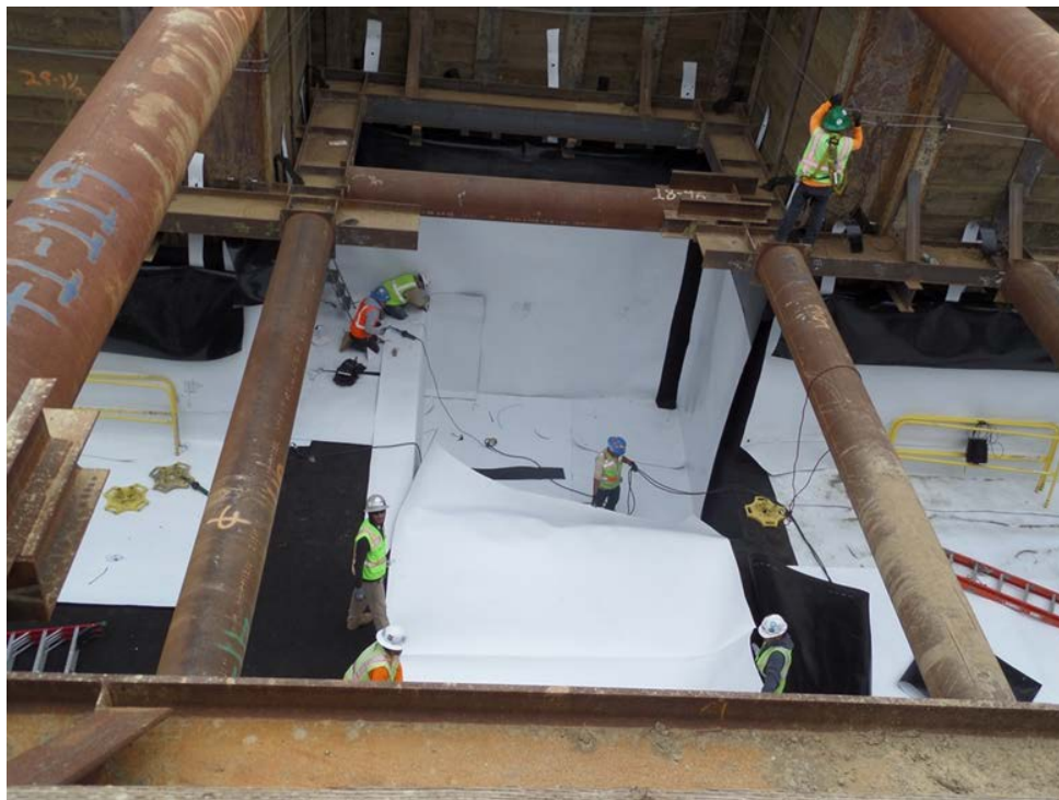
UG#1 – Waterproofing (HDPE) installation at Sump Pump #2.
