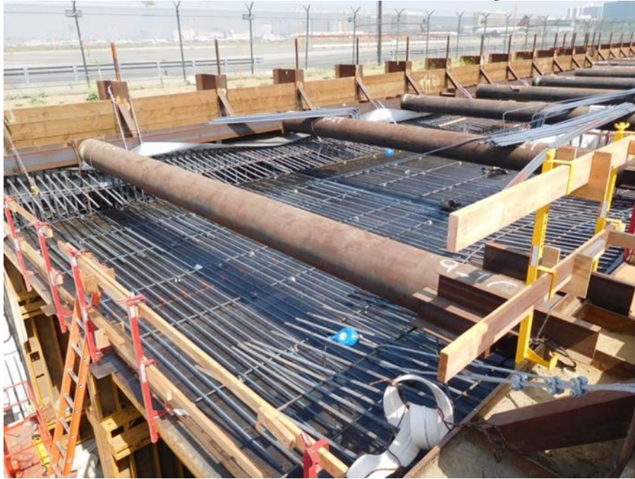
UG#1 – Roof slab rebar installation for the cut and cover tunnel section.
