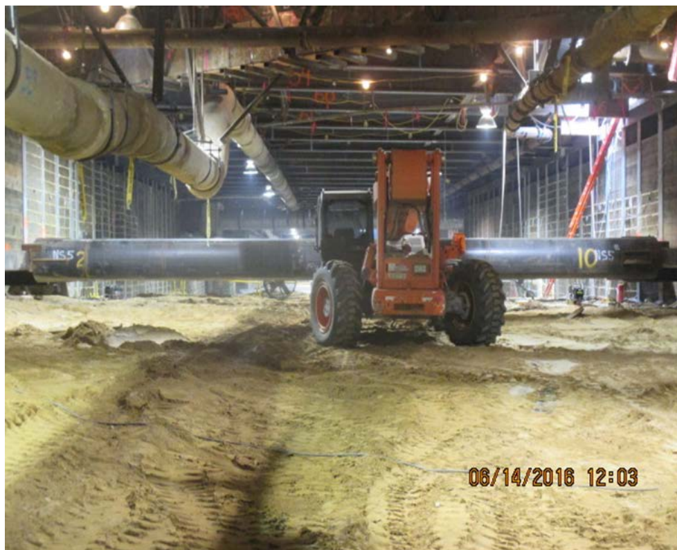
UG#4 – Staging struts.
