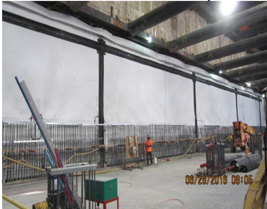
MARTIN LUTHER KING JR. STATION – Installation of geotextile membrane at the station.
