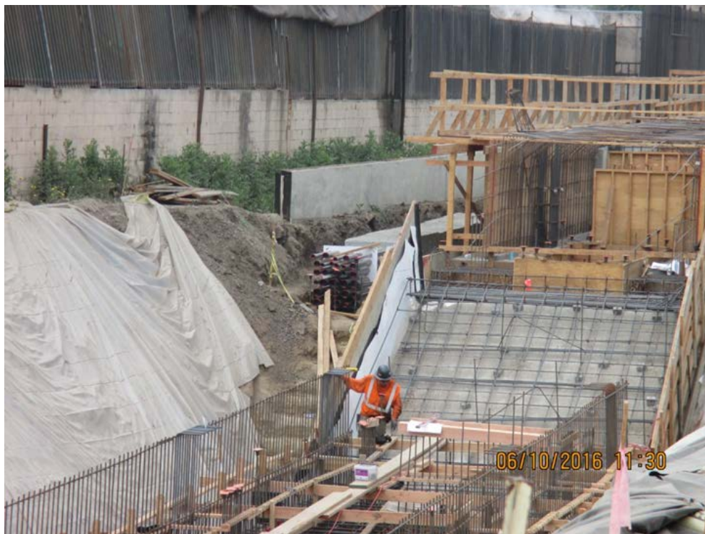
FAIRVIEW HEIGHTS STATION – Crews continue with MEP embed installation for the TC&C room invert. Poured the station platform footing and stem walls.
