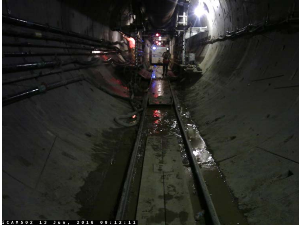
TUNNELING – Looking south into the southbound tunnel.
