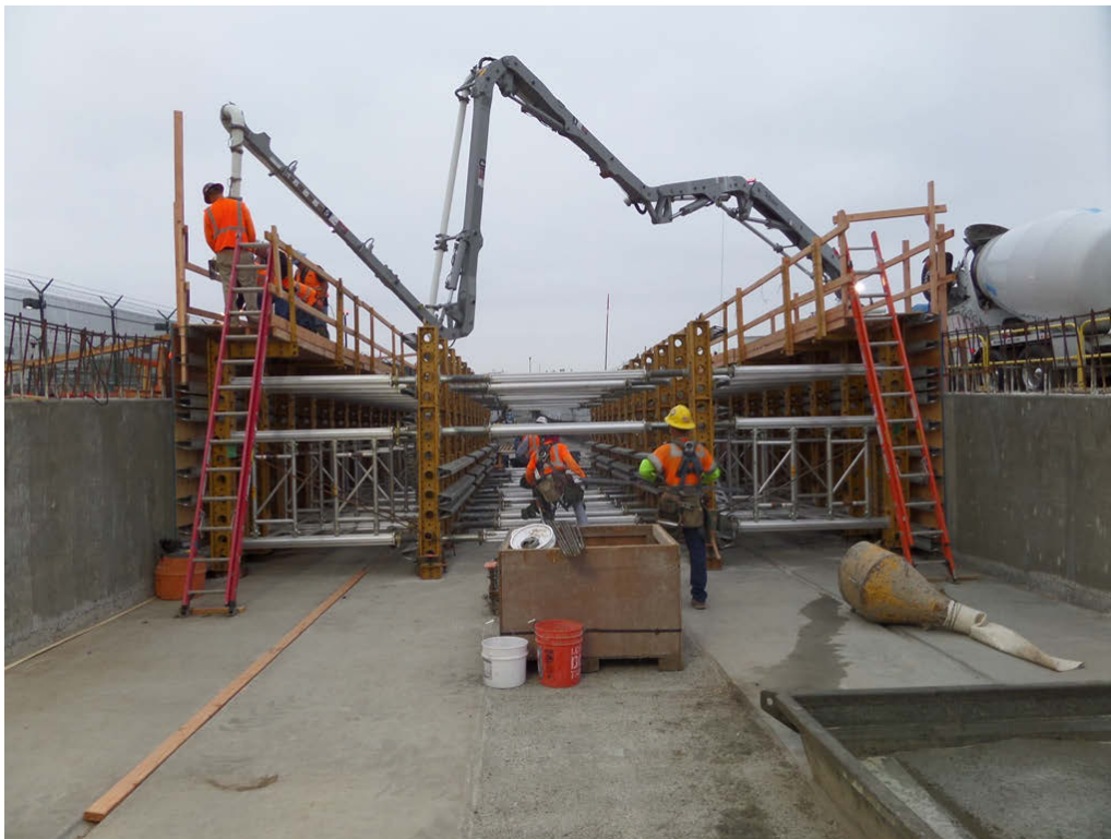
UNDERGROUND GUIDEWAY 1 - Crews continue with sequential construction at Underground Guideway 1, progressing from south to north.
