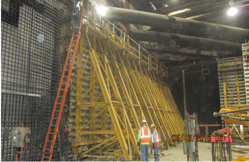
EXPOSITION STATION – Stripping forms for the previous lower wall placement.
