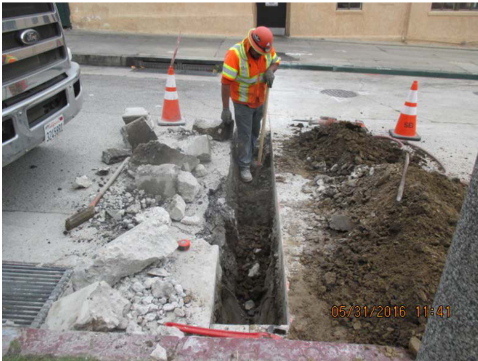
PARK MESA HEIGHTS – New electrical utility placement.
