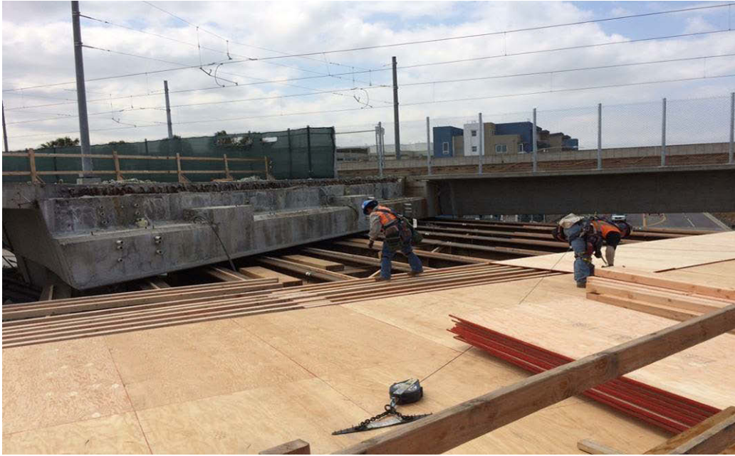
GREENLINE UNDERPASS – Falsework erection complete; formwork placement, soffit exterior girder and overhang formwork placement continues.
