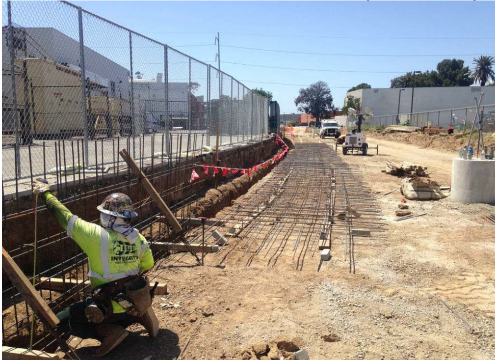
SEGMENT A – Ballast retainer wall construction ongoing.
