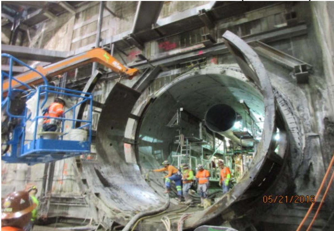
TUNNELING – Removal of thrust ring used to launch the TBM.
