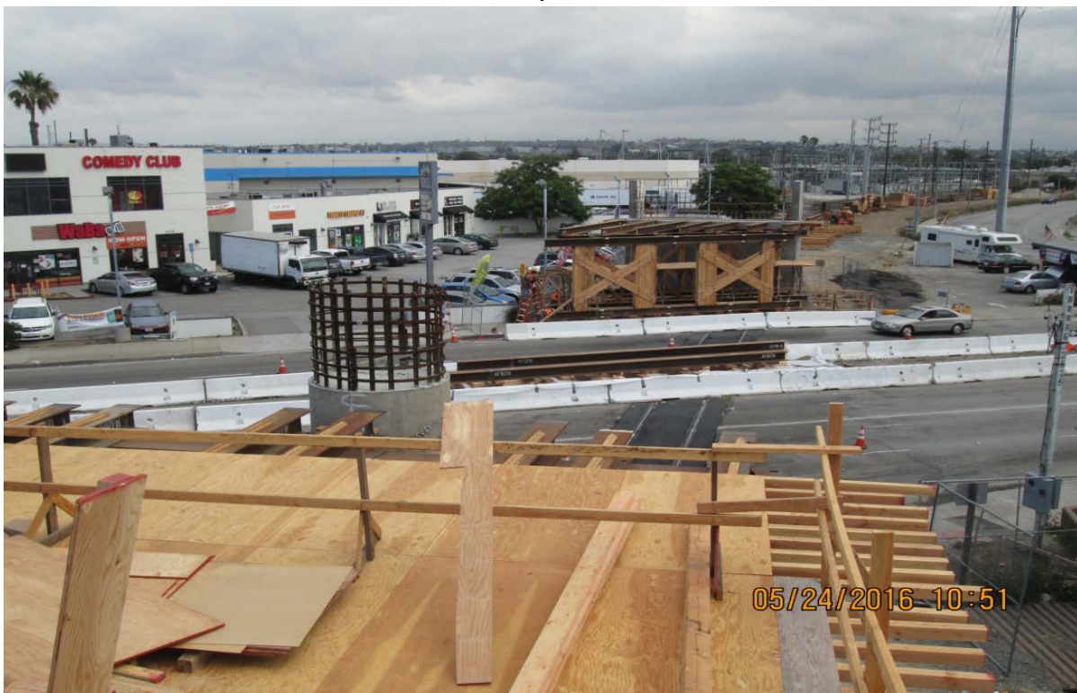
MANCHESTER BRIDGE UNDERPASS – Looking up the station.
