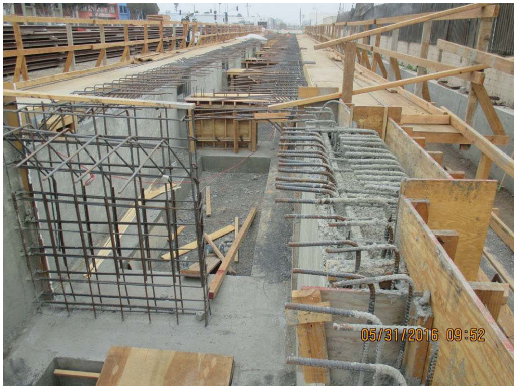
FAIRVIEW HEIGHTS STATION - Crews installed MEP embeds for the TC&C room invert. Crews poured the station platform footing and stem walls.
