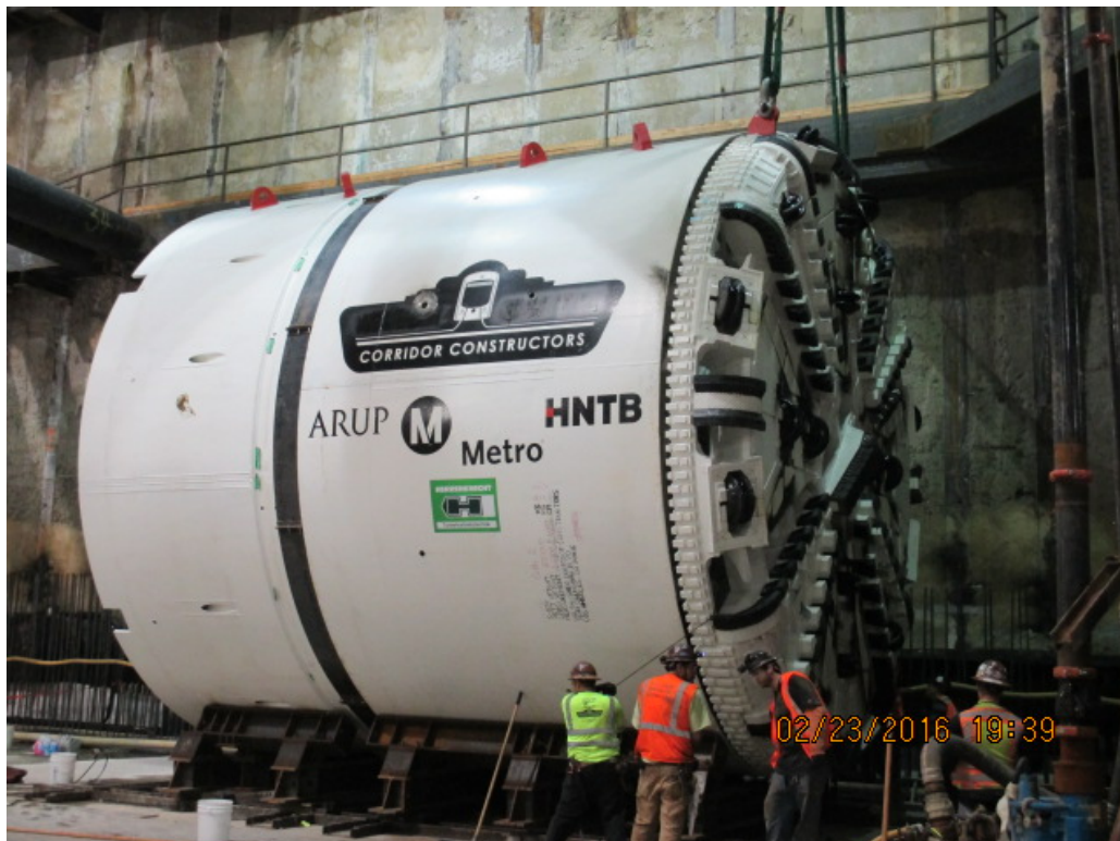
EXPOSITION/CRENSHAW STATION – Attaching Tunnel Boring Machine (TBM) cutter head to the front shield.
