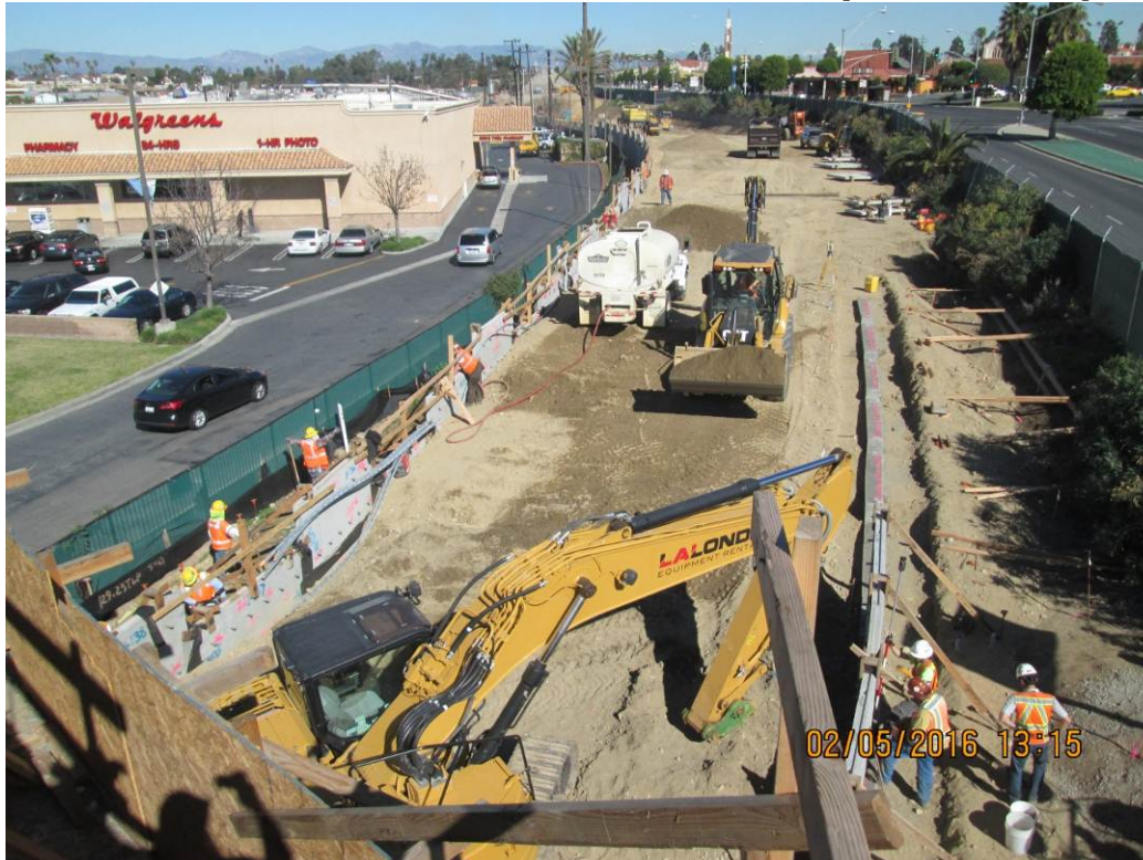
MSE WALL 202L&R - Crews continue to work on subgrade preparation, leveling pads, precast panel erection, strap placement and embankment backfill.
