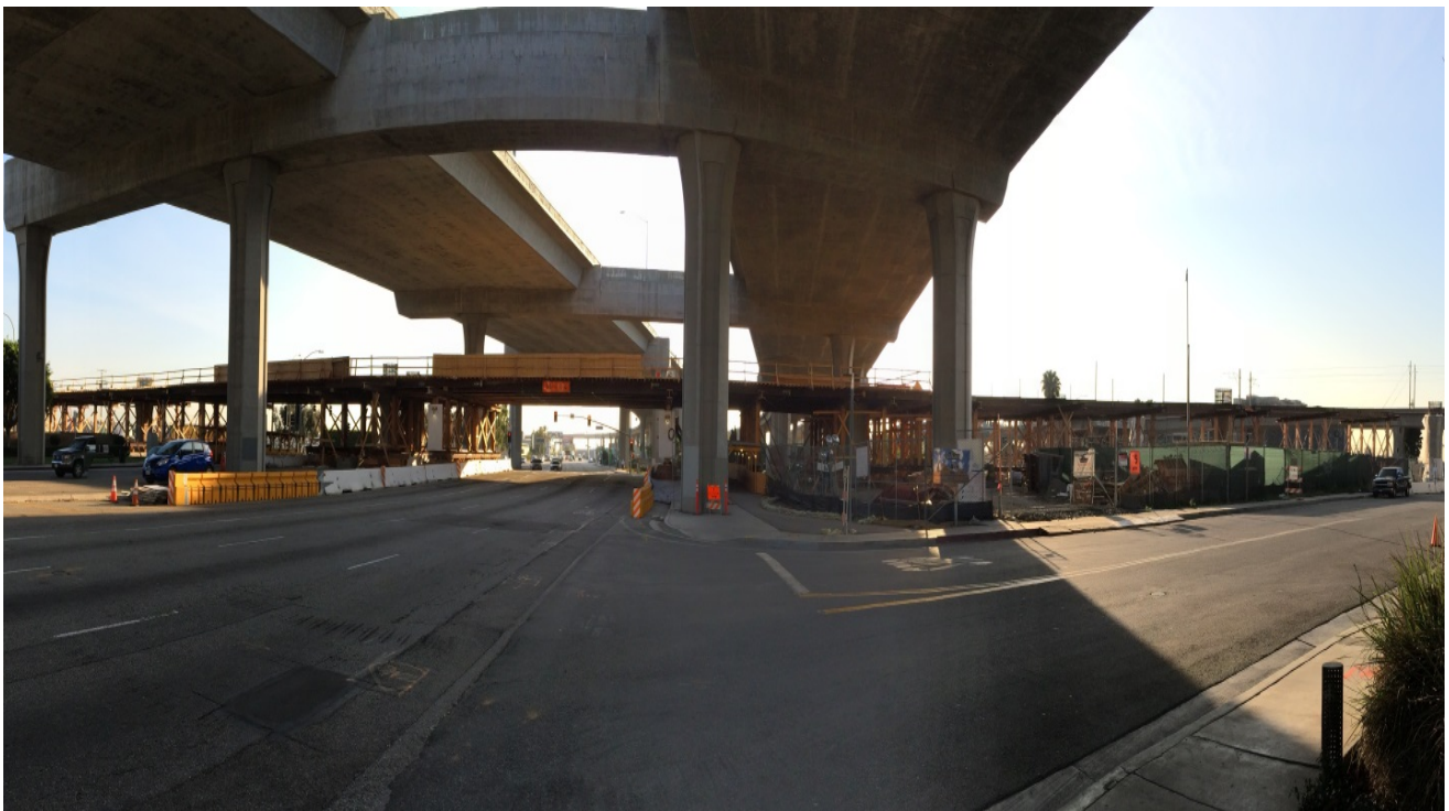
GREENLINE UNDERPASS – Falsework and rolling soffit continue
