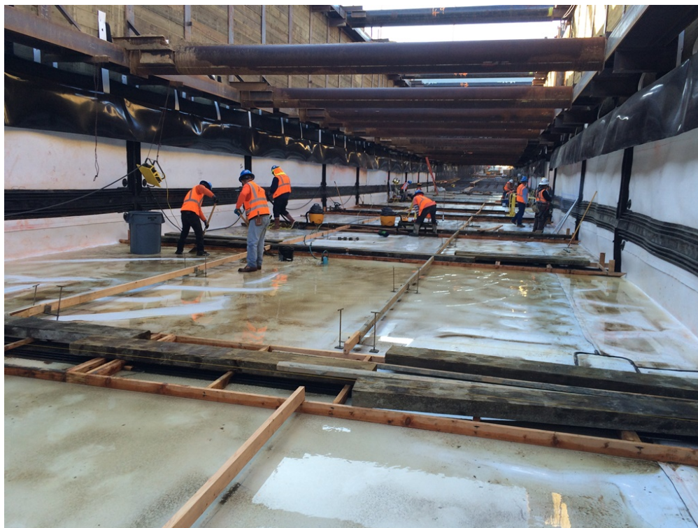
UG1 – Installing waterproof membrane
