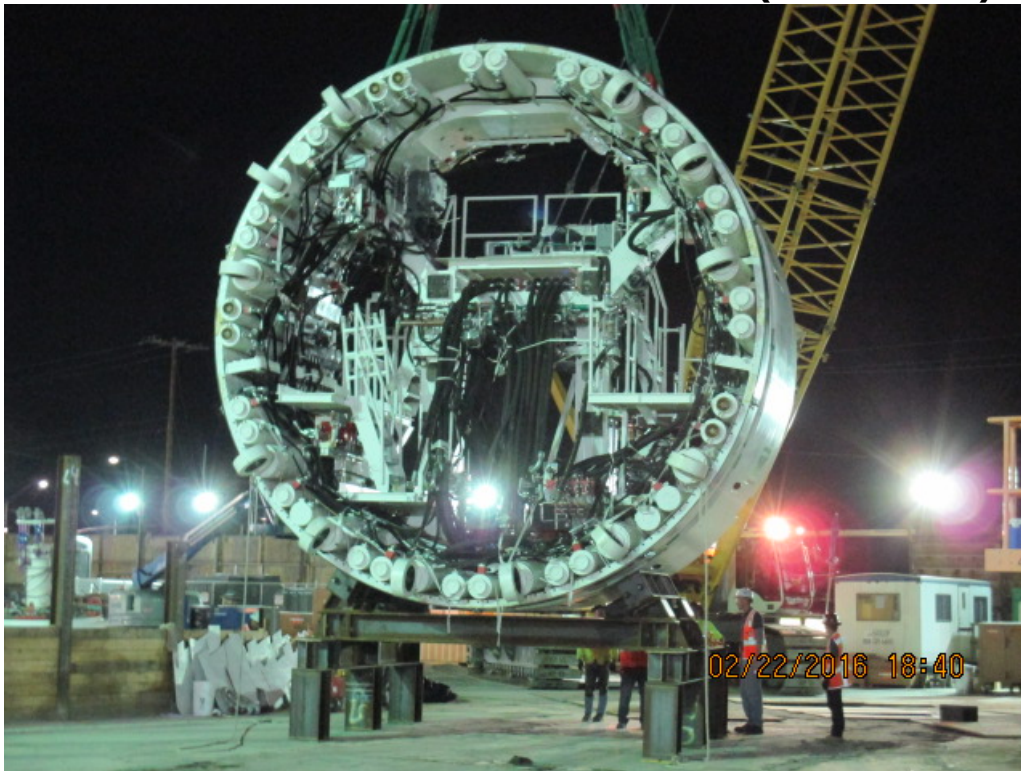
EXPOSITION/CRENSHAW STATION – Lowering of mid-shield of Tunnel Boring Machine (TBM) into Expo station
