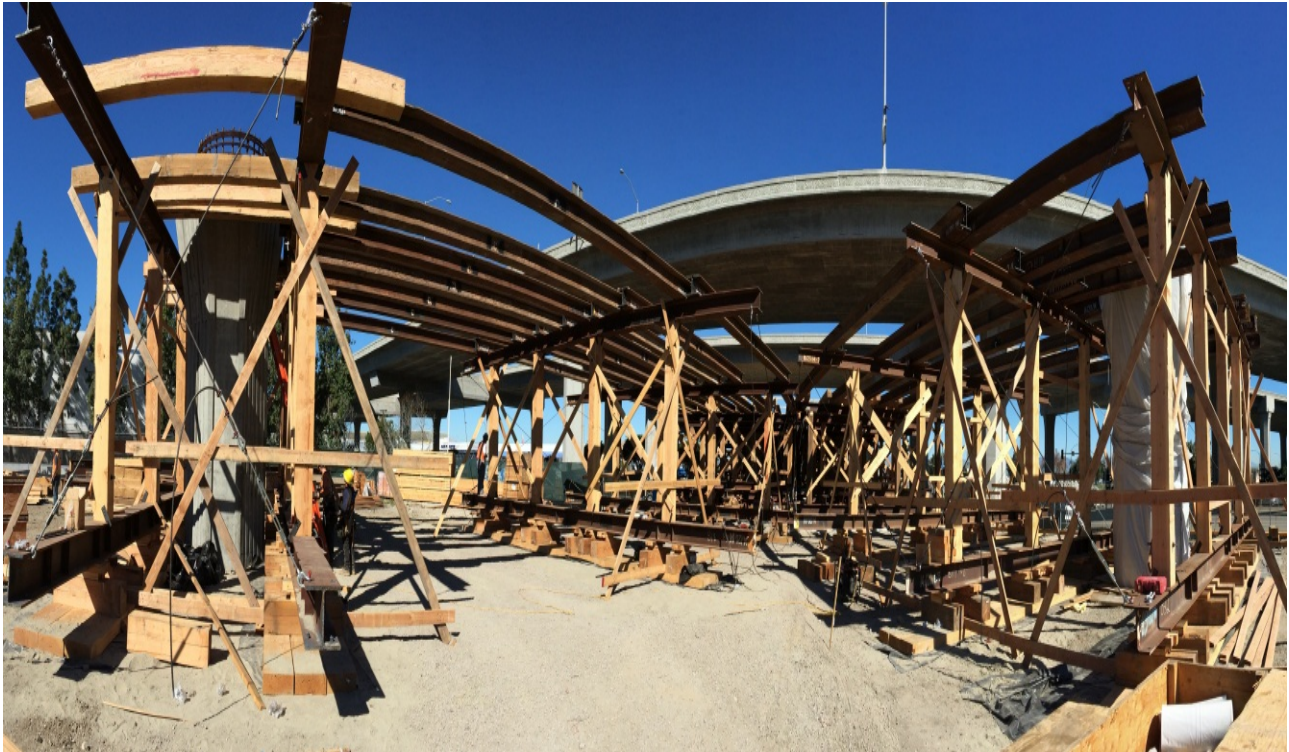
GREENLINE UNDERPASS – Falsework and rolling soffit continue
