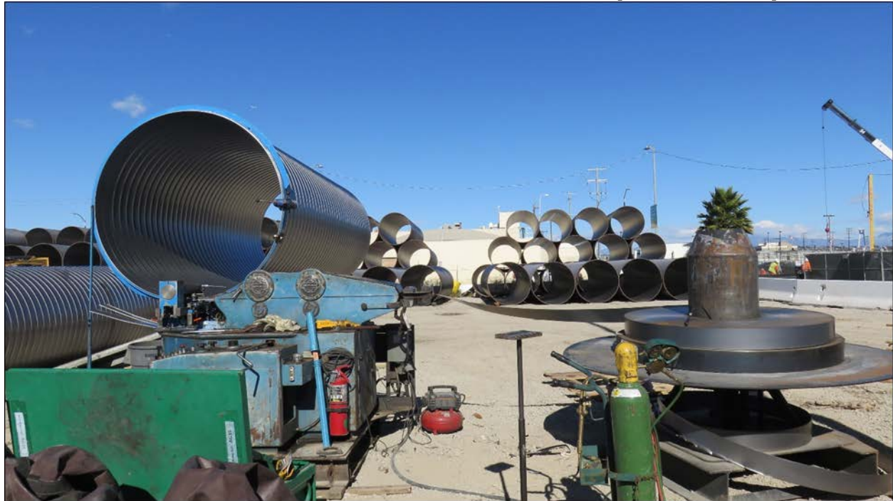
Tunnel ventilation fabrication at Bellanca Yard.
