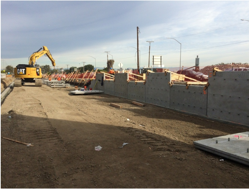
MSE Wall 17L&R (Mechanically Stabilized Embankment): Precast Panel placement begins. Leveling pads and subgrade preparation nearly complete.
