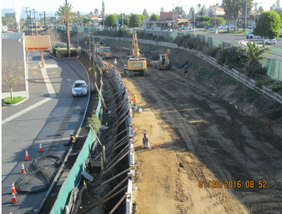
MSE WALL 202L&R: Crews continue to work on subgrade preparation and leveling pads for MSE 202L&R. Crews have begun to work on precast panel erection and strap placement/backfill for 202L.
