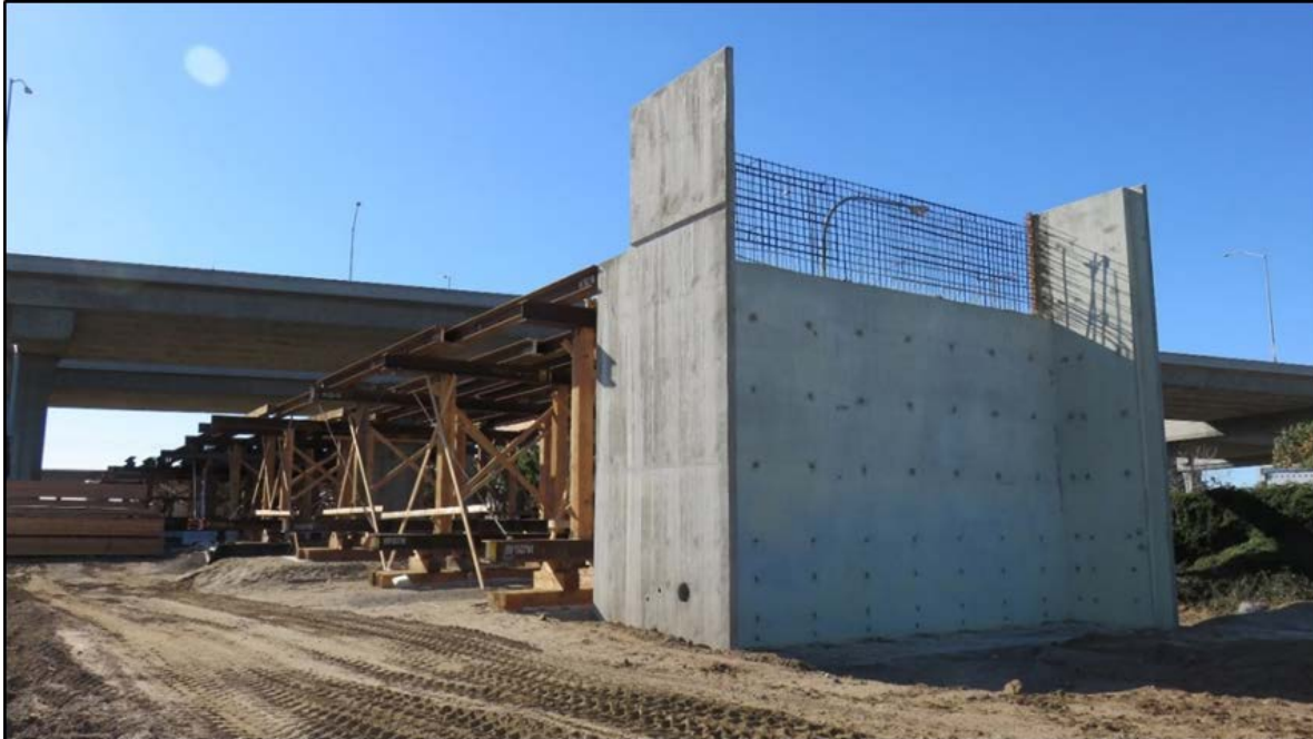
Completed (North) Abutment and Falsework.
