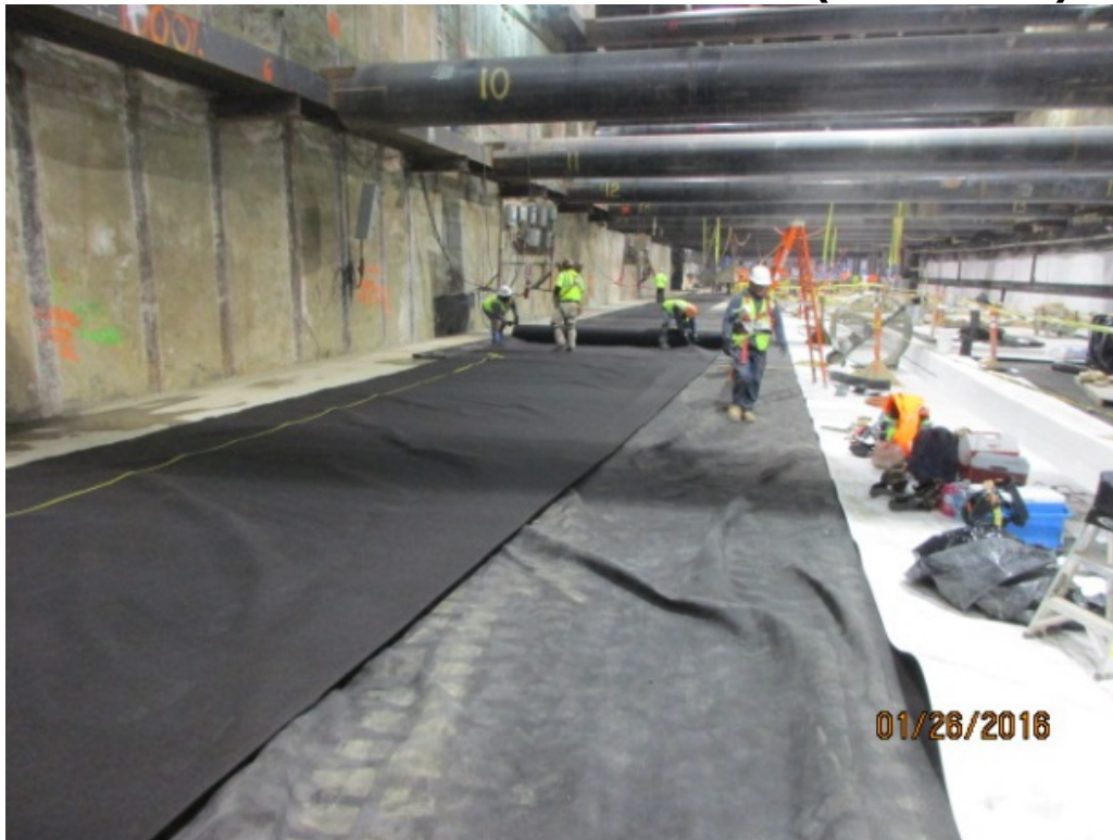
EXPOSITION/CRENSHAW STATION – Installation of waterproofing components
