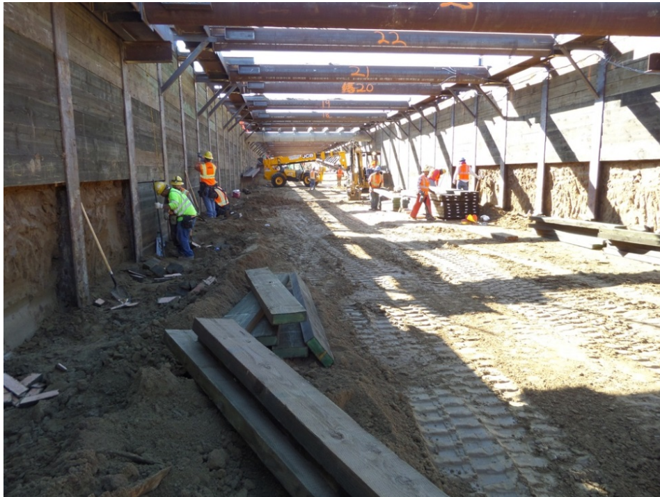
UG#1 - Struts and wales being installed per plan. Tier 2 lifts and kickers being installed in preparation for tier 2 walers and struts. Treated lagging installation ongoing as excavation continues.
