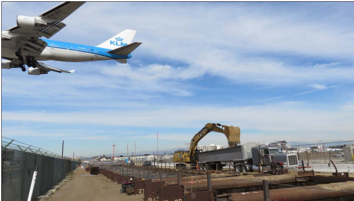
UG1 – On-going excavation.
