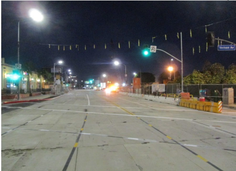
UG4 – Decking complete; looking north from Vernon.
