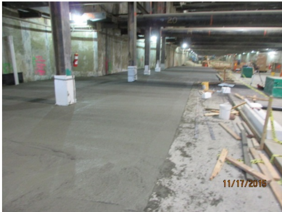
EXPO/CRENSHAW STATION – Phase 2 mud slab installed at the central portion of Expo station box.
