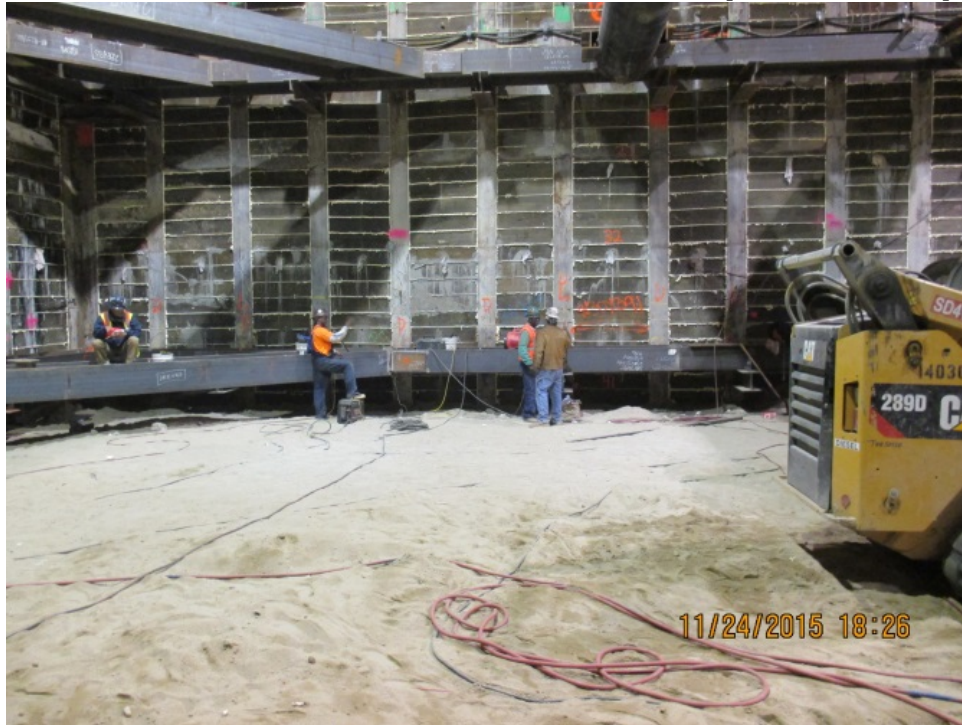
LEIMERT PARK STATION – Tier 2 wale welding operation.
