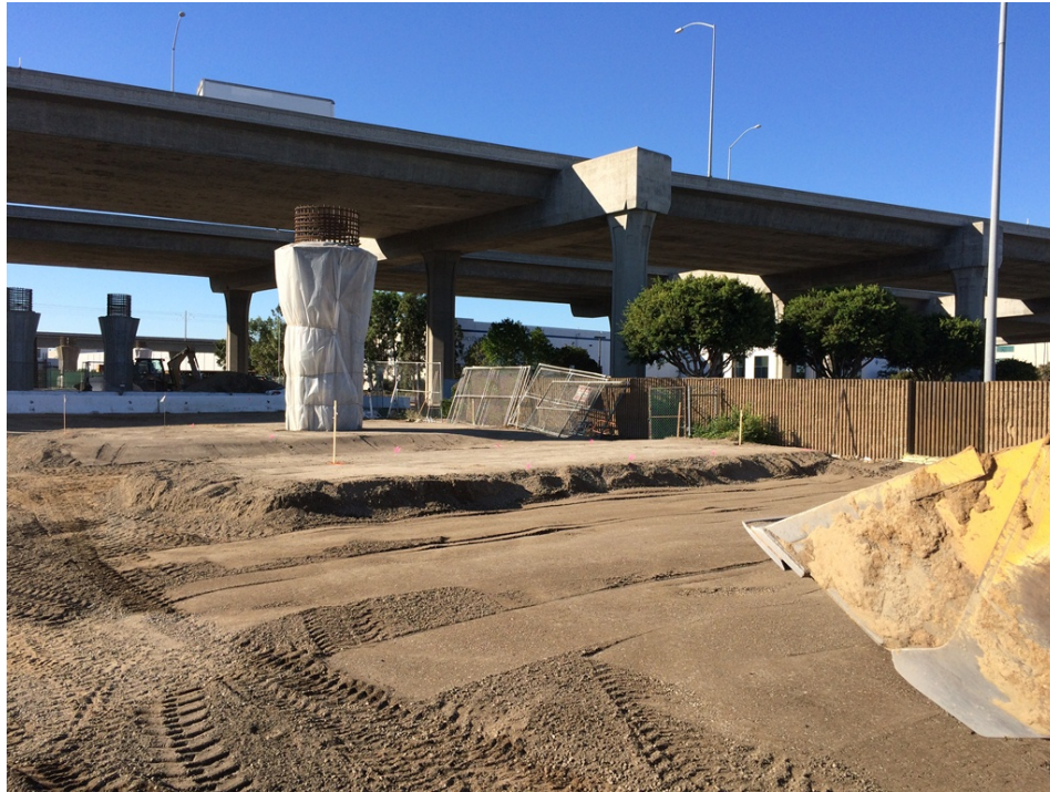
GREENLINE UNDERPASS - Subgrade compaction for falsework erection.
