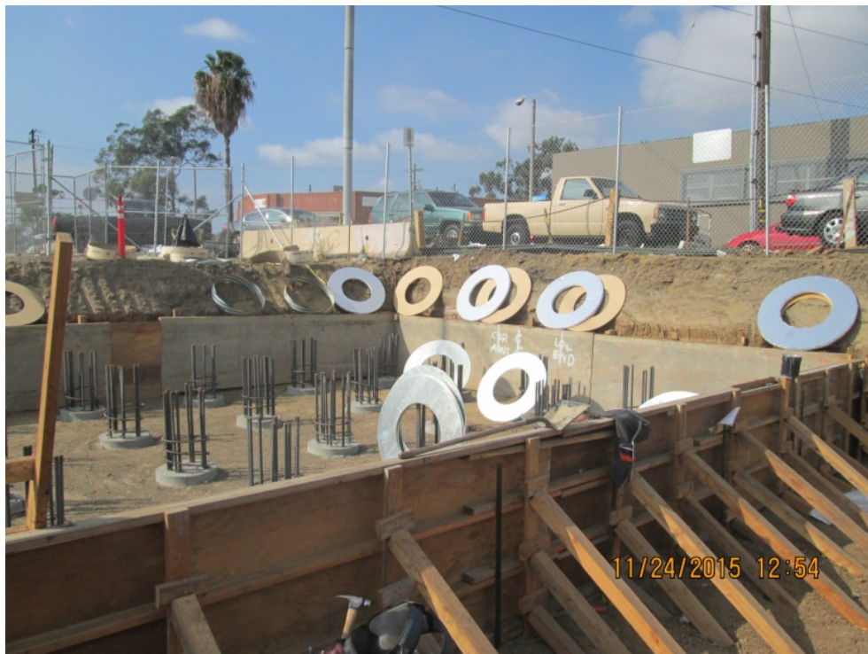
I-405 BRIDGE - Abutment 5 footing construction ongoing.
