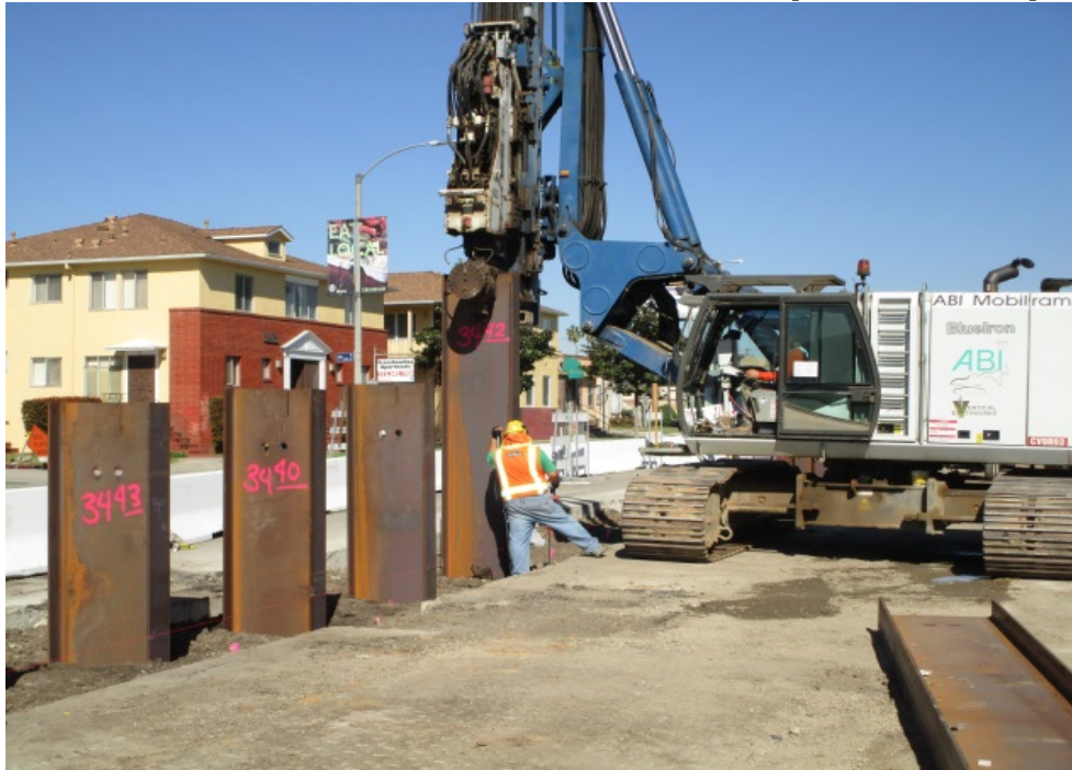
UG3 – Vibrating piles at UG3 looking north (Near Crenshaw and 58 th Pl.).
