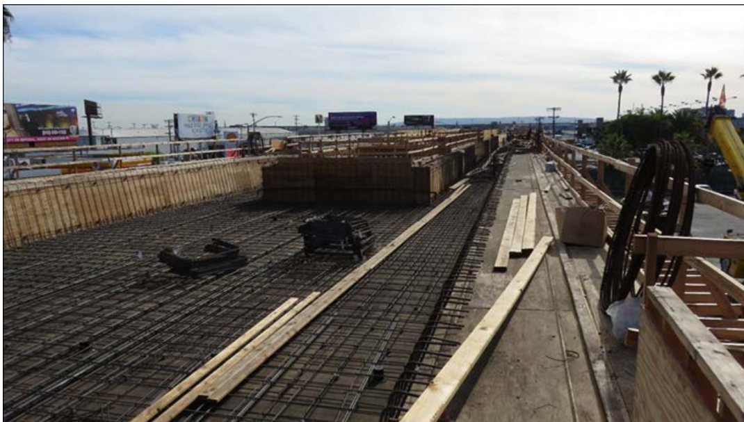
CENTURY BRIDGE – Super Structure Rebar.
