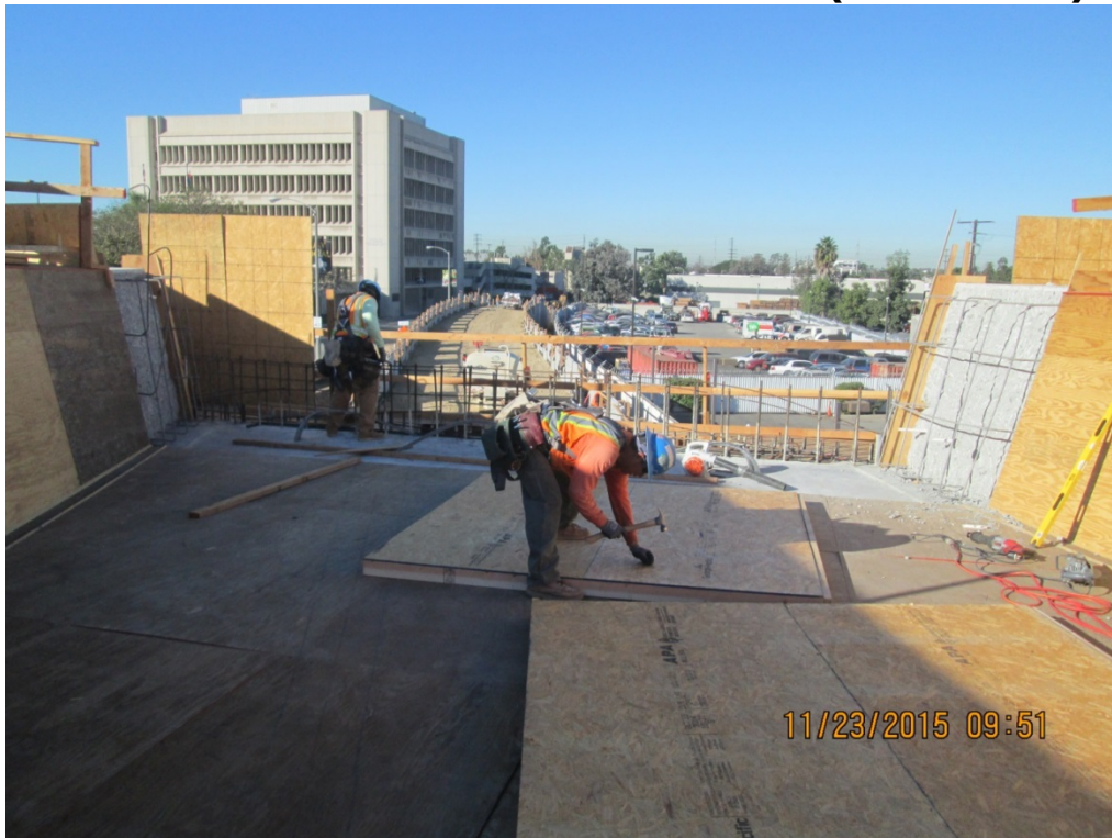
LA BREA BRIDGE - Back wall formwork.
