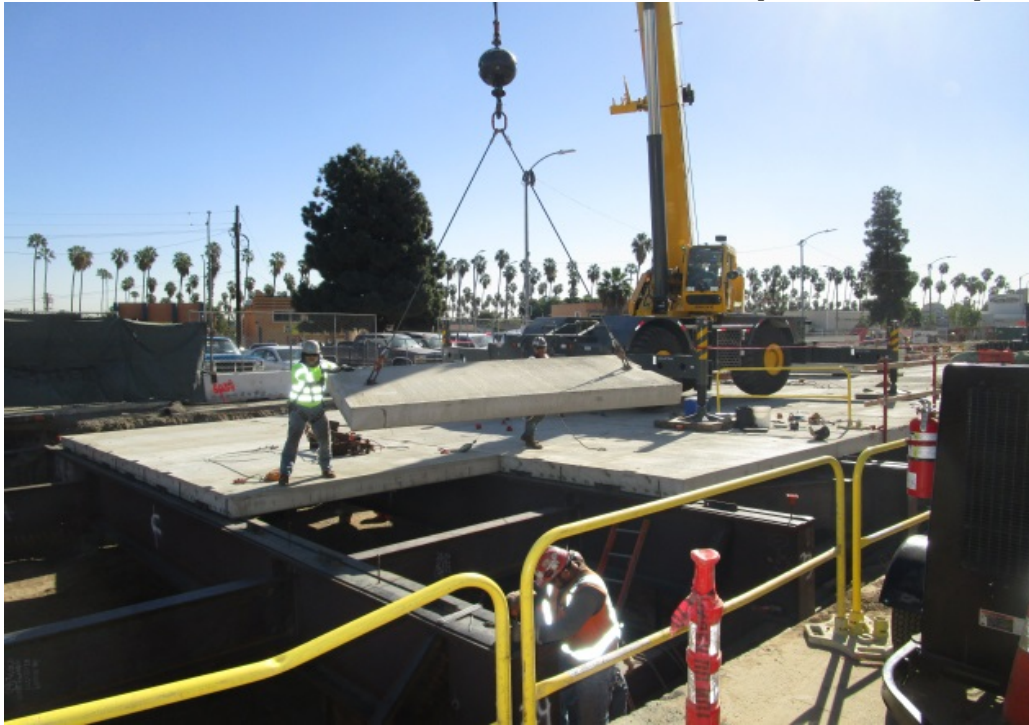
UG4 – Setting precast deck panels looking south.
