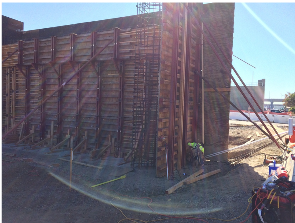
111 TH STREET BRIDGE - Abutment 2 formwork installation.
