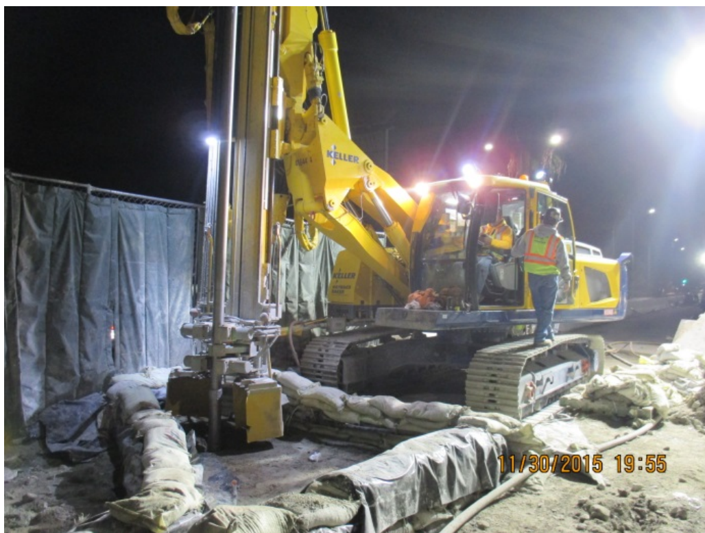
CROSS PASSAGE 2 – Jet grouting operation.
