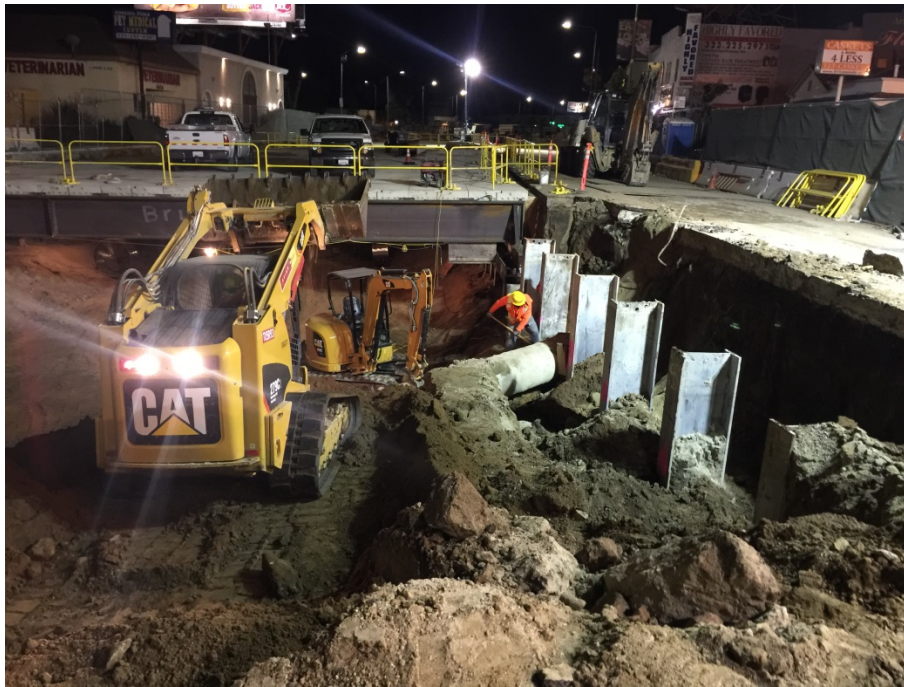
UG4 – Excavation operation around utilities.
