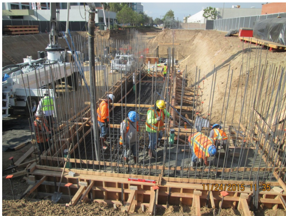
FAITHFUL CENTRAL BIBLE CHURCH - Pedestrian Underpass: Wall steel placed for tunnel/walkway structure.
