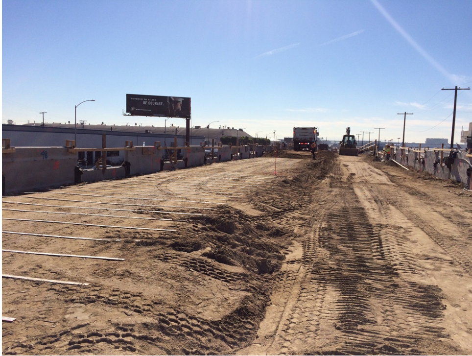
MSE (Wall 3, 60L&R): Precast Panel erection, placement of soil reinforcement, backfilling and compaction testing ongoing.
