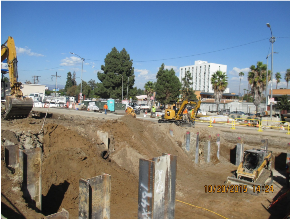
UG#4 – Asphalt demo and excavation for decking operations
