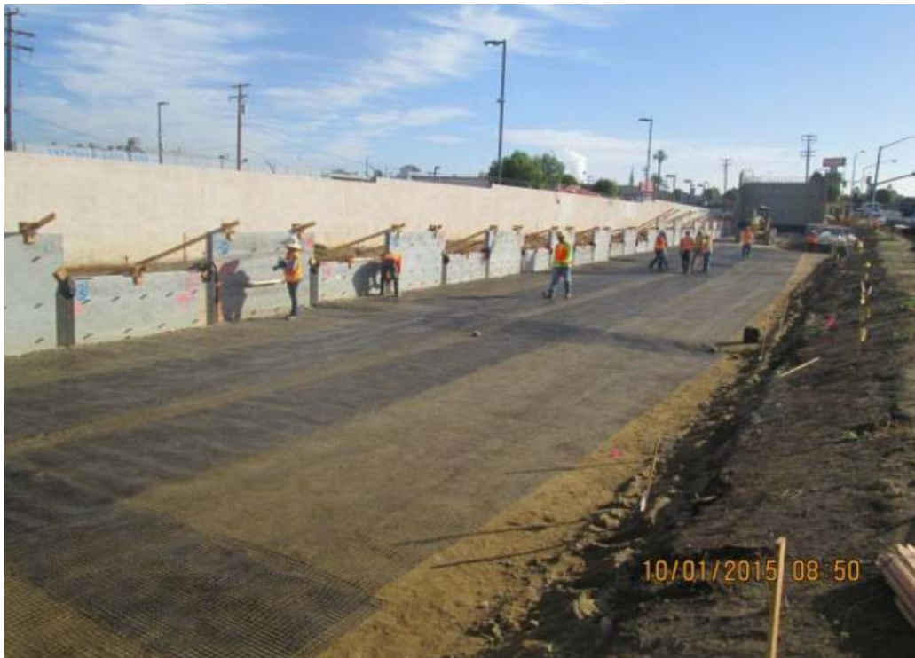
B1 GUIDEWAY – MSE Wall Panel erection and galvanized strap placement
