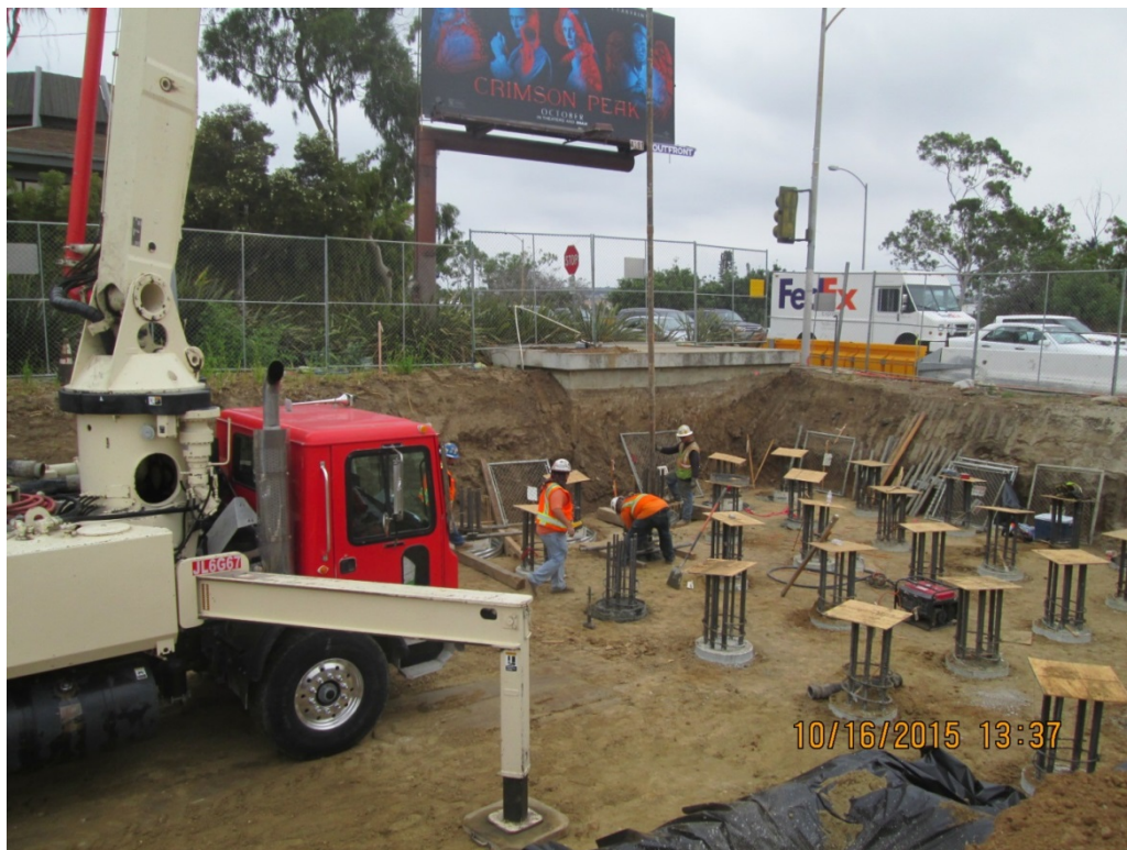
I-405 - Abutment 1 CIDH placement
