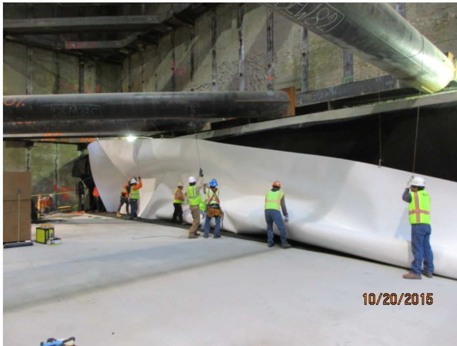
CRENSHAW/EXPOSITION STATION – Installation of HCR membrane over Geotextile
