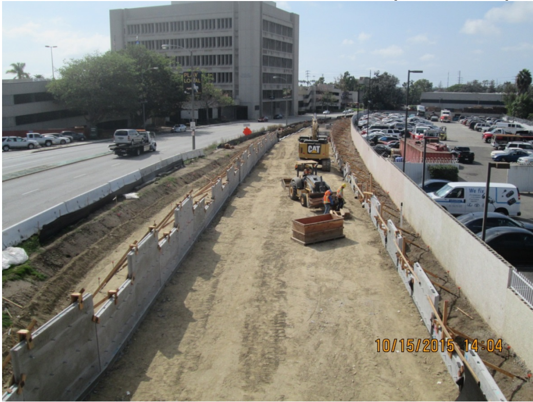
LA BREA BRIDGE - MSE panel erection
