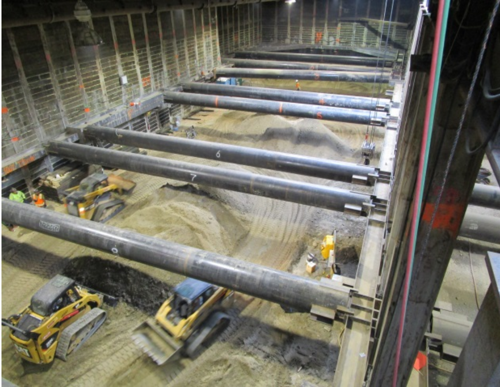
LEIMERT PARK STATION – Excavation operation looking north
