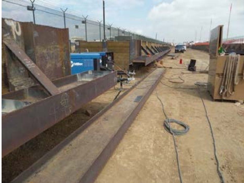
UG1: Welding walers along West pile line.
