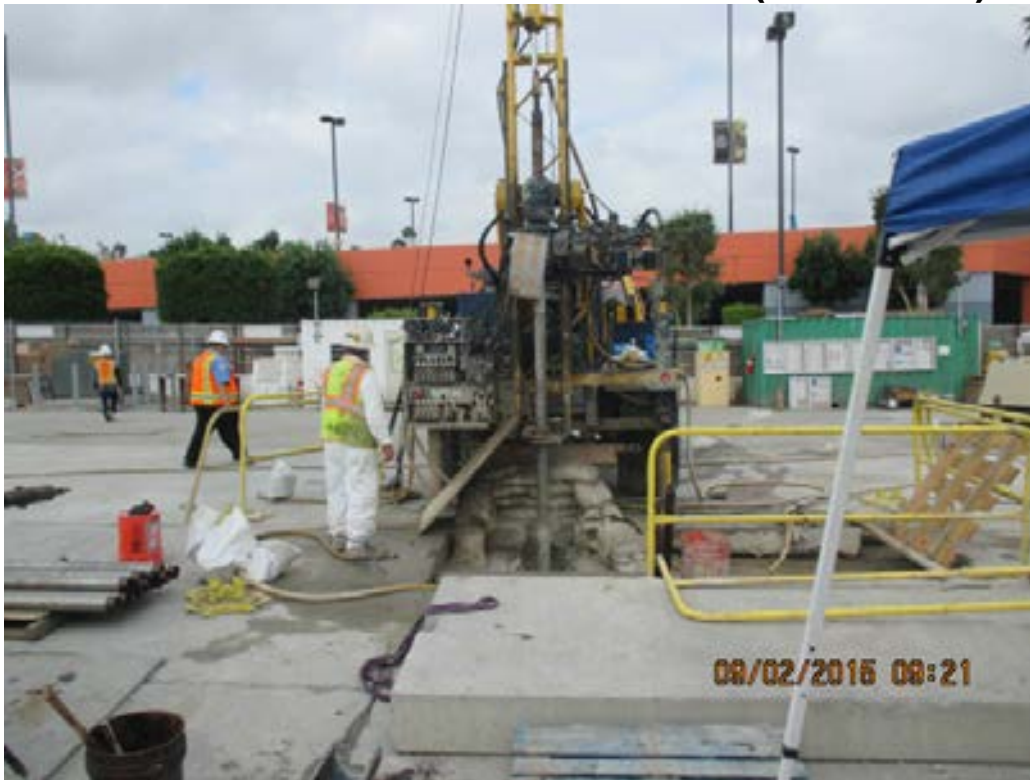
MLK STATION – Coring jet grout panels at MLK for QC testing.
