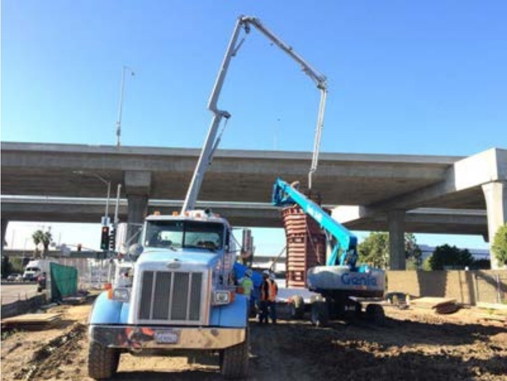
GREEN LINE: Poured Bent 5 column and finished installing abutment 6 formwork.
