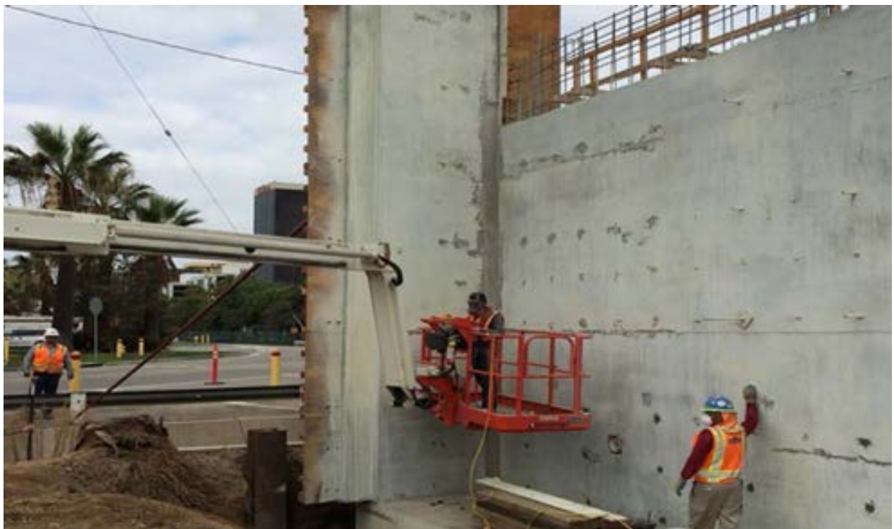
AVIATION/CENTURY : Bent 6 & 7; bent cap formwork construction. Abutment 1 footing; debris on subgrade, formwork and lagging removed.
