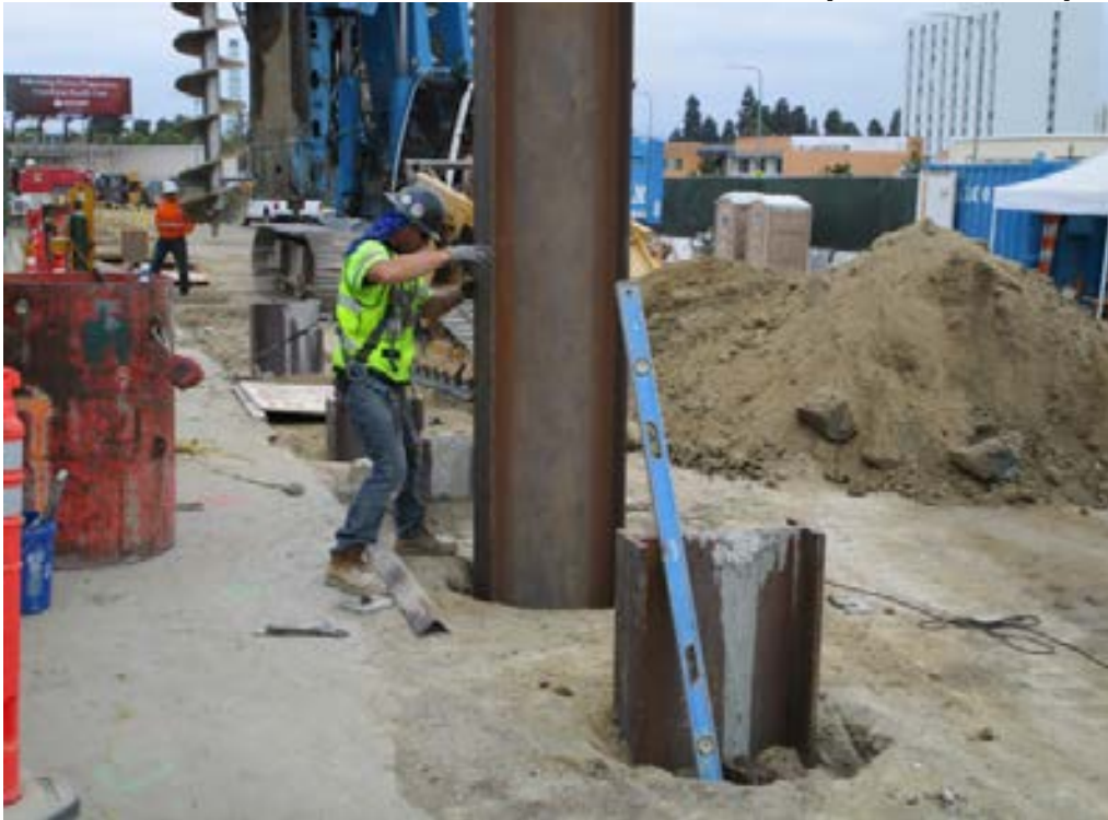
UG4 – Setting pile on the south side of UG4.
