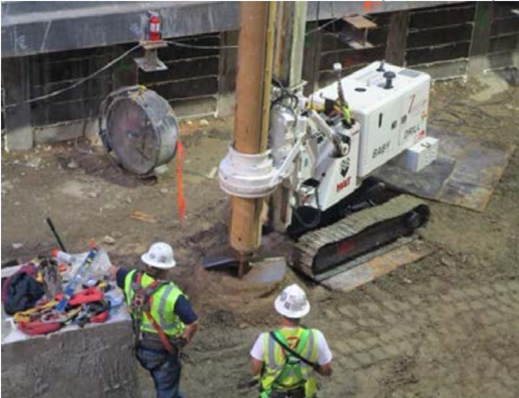
LEIMERT PARK Drilling for elevator Shaft #2.
