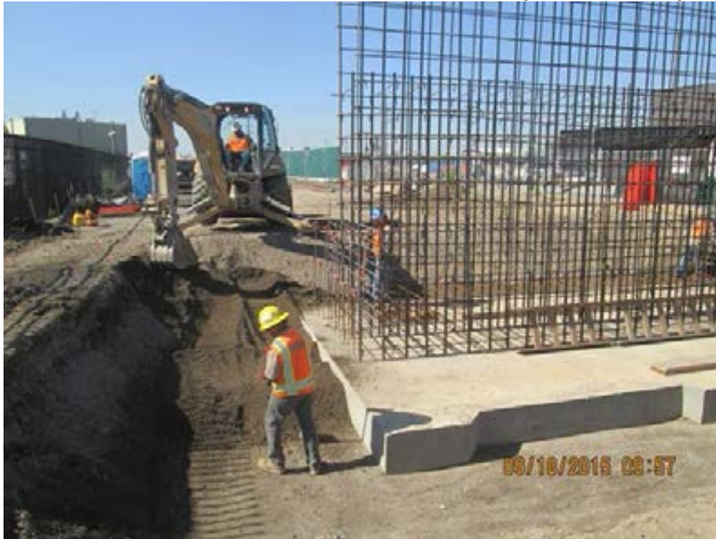
MANCHESTER – Abutment 1, structural backfill.
