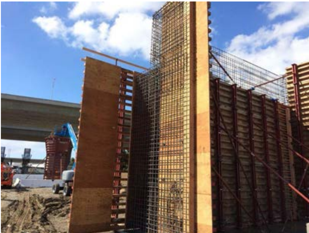
GREEN LINE: Poured Bent 5 column and finished installing abutment 6 formwork.
