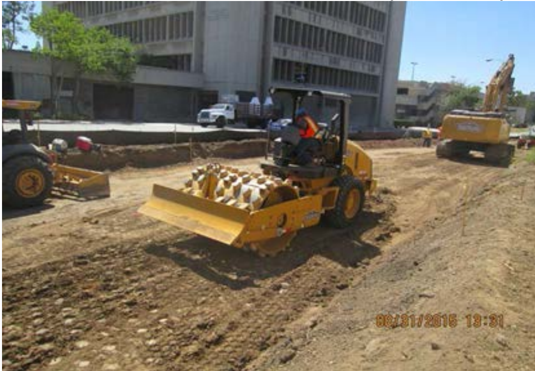
B1 Guideway: Excavation for MSE wall leveling pad (MSE 192L&R).
