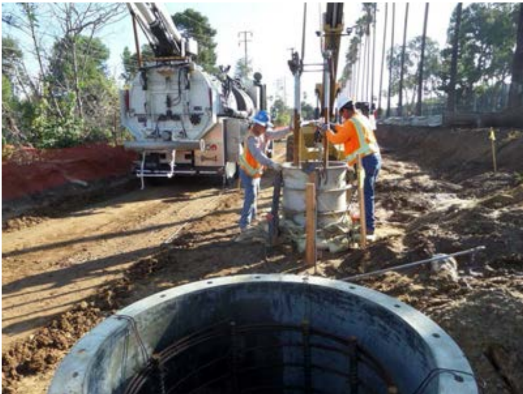
B1 GUIDEWAY – Continued OCS foundation work.
