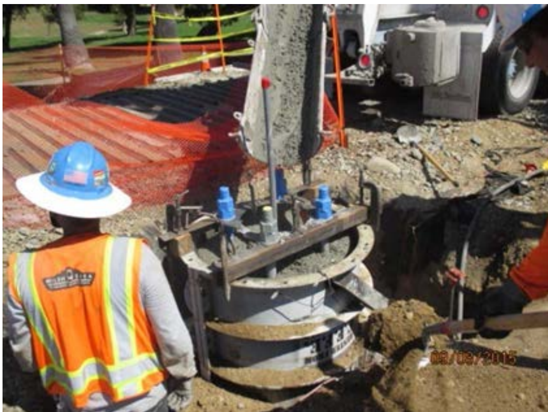
B1 Guideway: Pouring OCS foundations between Cedar and Centinela (12 complete).
