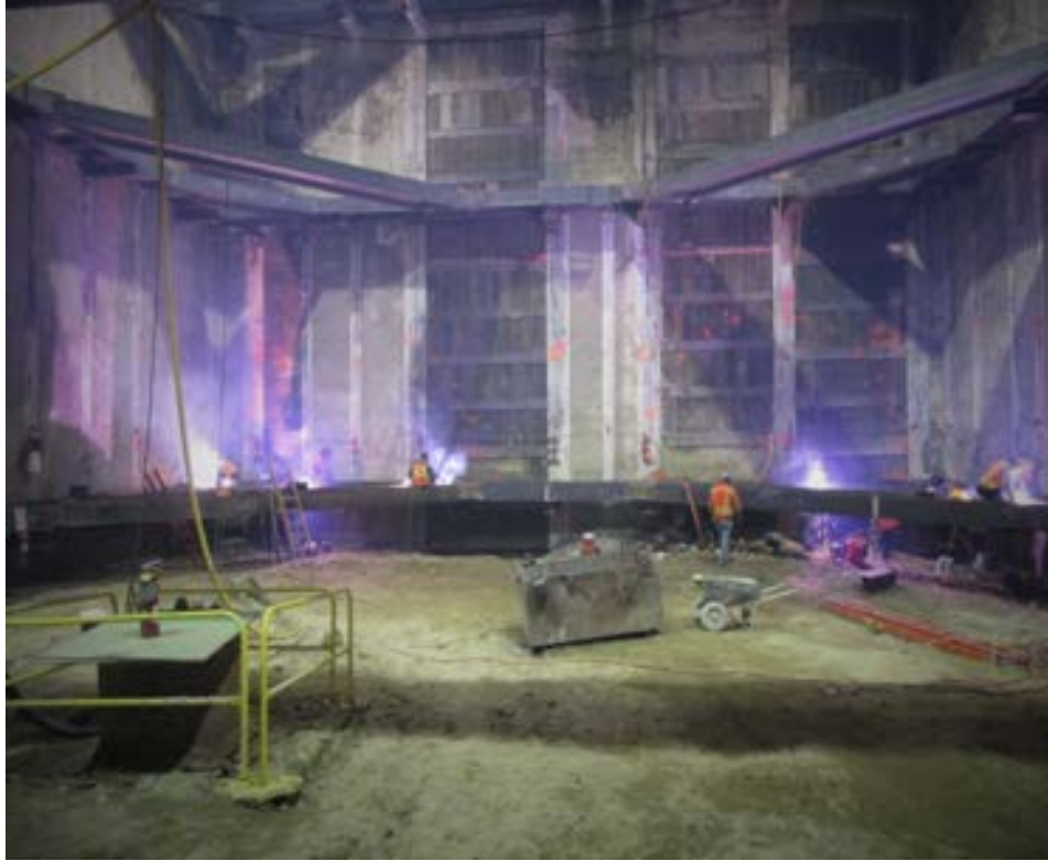
EXPOSITION/CRENSHAW – Tier-3 welding operation on south headwall.
