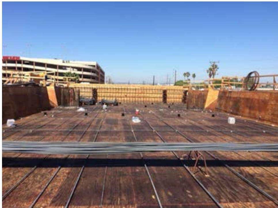
AVIATION/CENTURY Span 6 soffit rebar placement.
