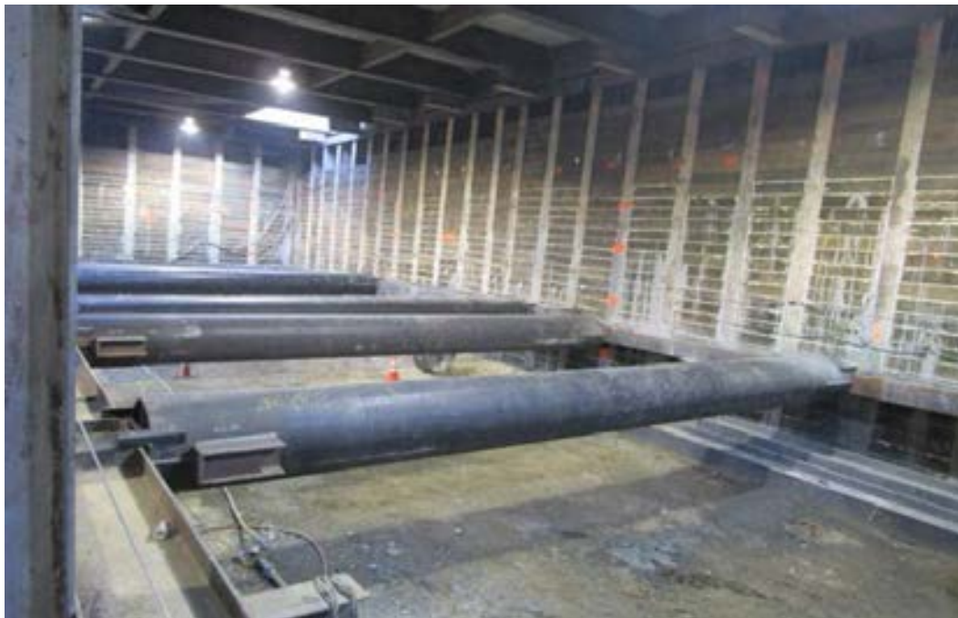
LEIMERT PARK Staged Tier 1 struts east of pin piles.
