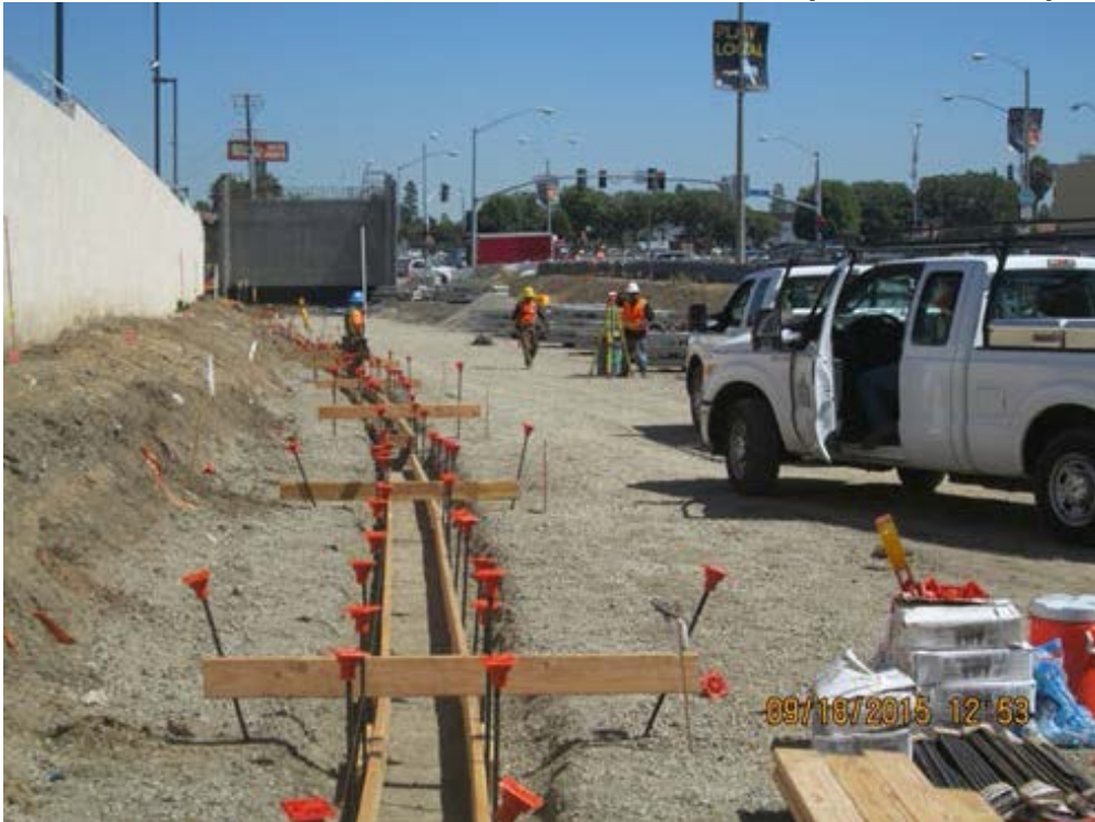
B1 GUIDEWAY - Cutting grade and leveling pad.
