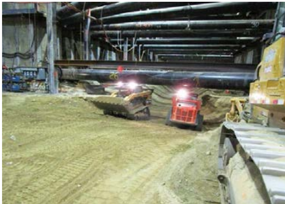
EXPOSITION/CRENSHAW – Excavating trough beneath Tier 3 pipe struts.
