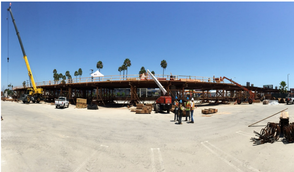
AVIATION/CENTURY STATION – Underpass Falsework Span 4 to 7.
