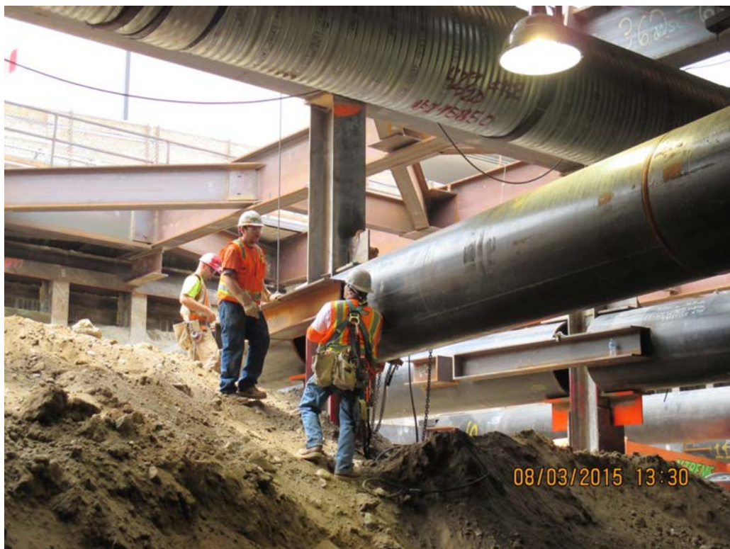
MARTIN LUTHER KING JR. STATION – Strut Installation at the station.
