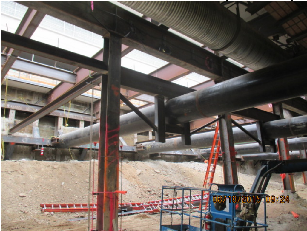
MARTIN LUTHER KING JR. STATION – Mid span strut support.
