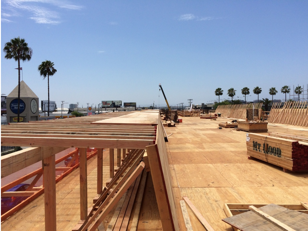
AVIATION/CENTURY STATION – Underpass Girder Stem and Overhang Formwork Placement.
