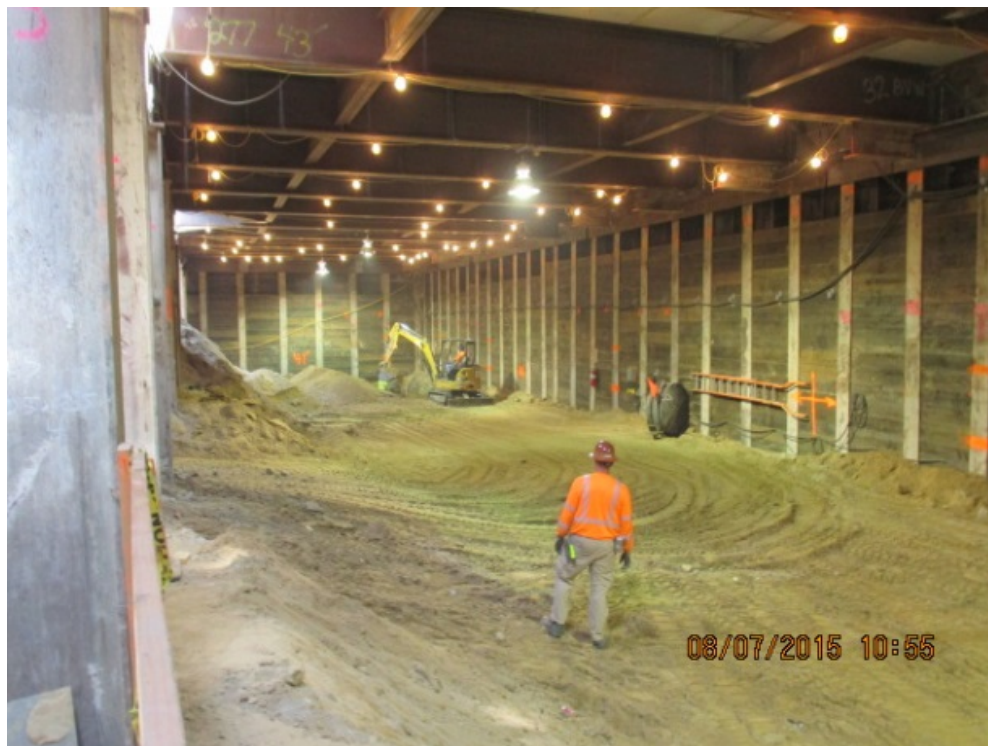
LEIMERT PARK STATION – Lagging operation at the station.
