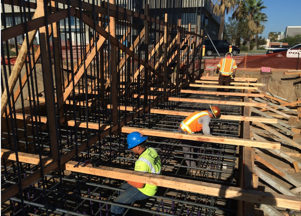
AVIATION/CENTURY – Underpass abutment 1 footing debris removal and epoxy U-bar tying.
