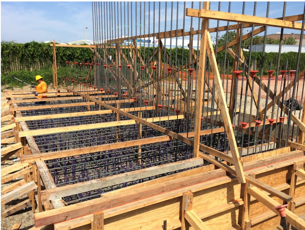
GREEN LINE – Underpass Abutment 6 Footing.
