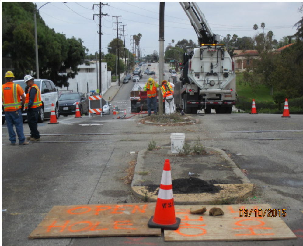
CENTINELA – Utility potholing on the north end.
