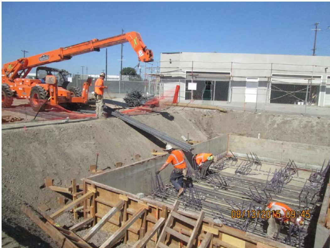
MANCHESTER AVENUE - Underpass abutment 1 footing steel placement.
