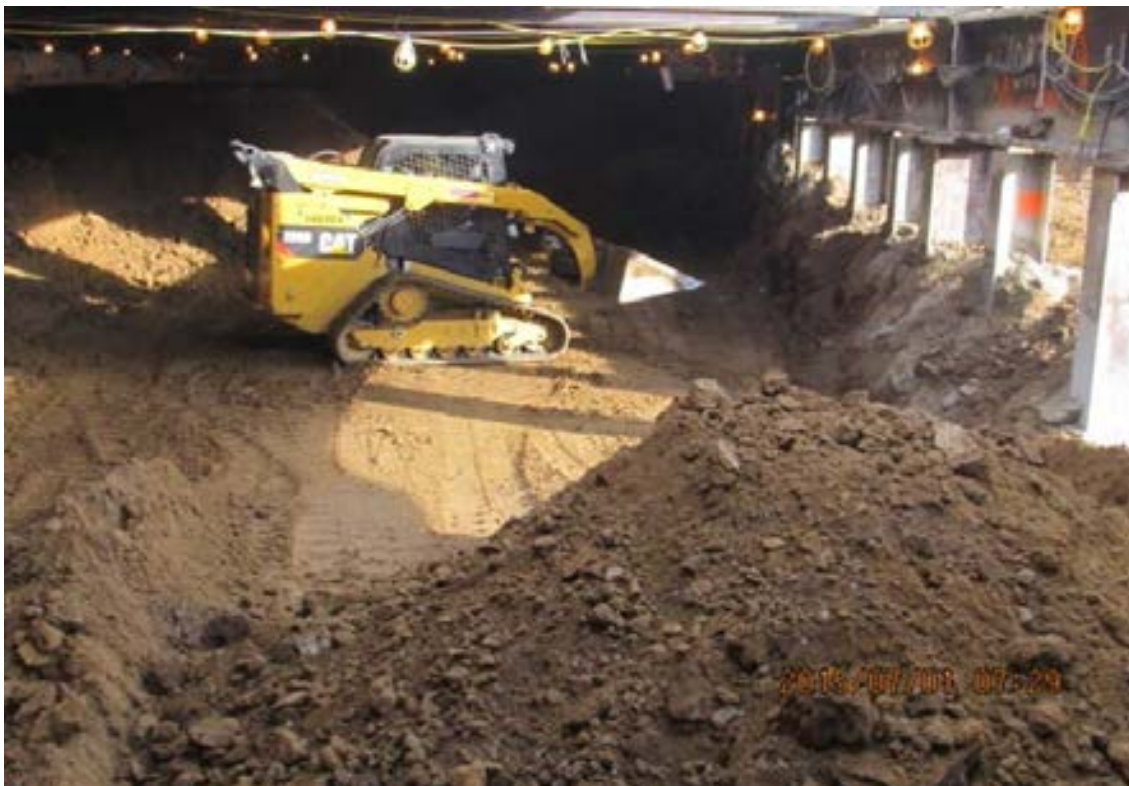
VERNON STATION - Excavation below Deck.
