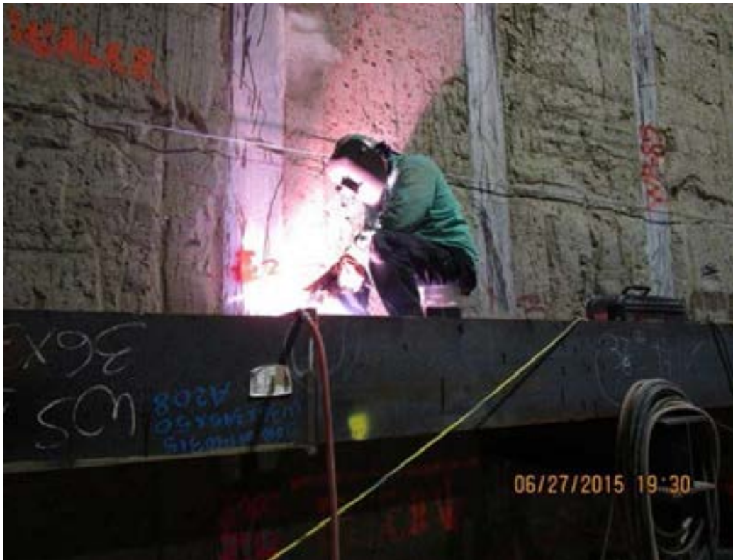
EXPOSITION STATION – Welding Tier 2 Bracing along the West Wall in the south Station.
