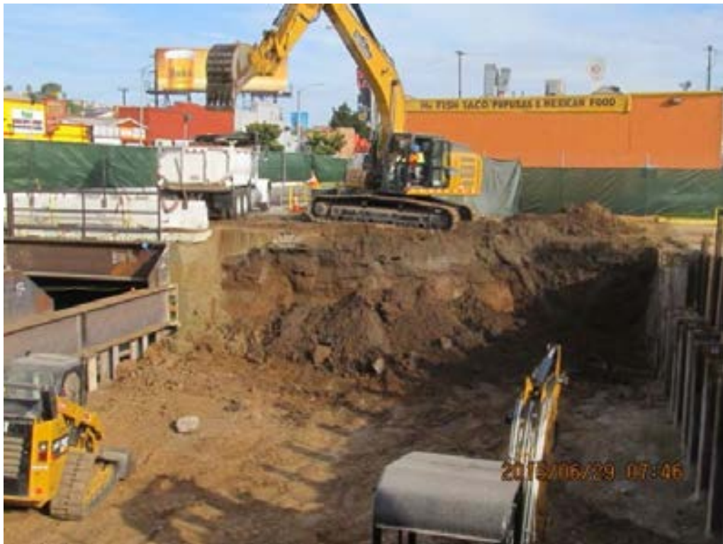
VERNON STATION - Looking north at the Excavation.
