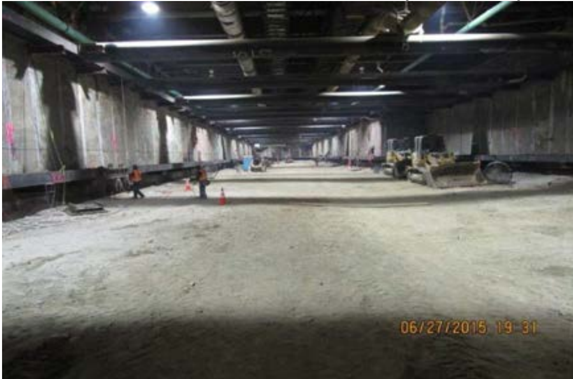
EXPOSITION STATION – Tier 2 bracing activities in the South Station.
