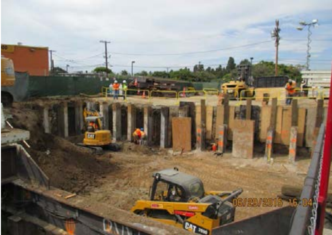
VERNON STATION – Excavation.
