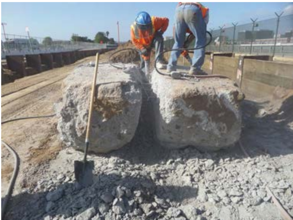
UG #1 - Ongoing demolition of the Navaid Lighting Foundation.
