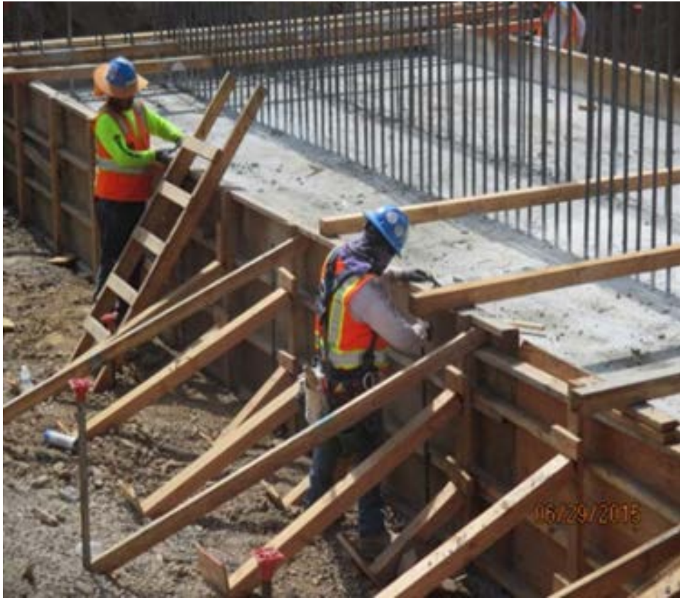
WSSC stripping forms from Imperial Abutment 10 Footing.
