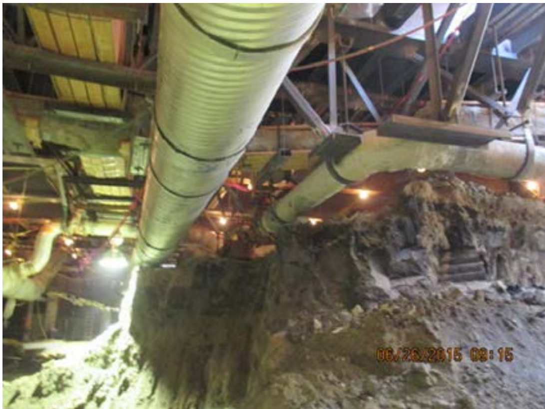
MLK STATION –Excavating under DWP fire line.
