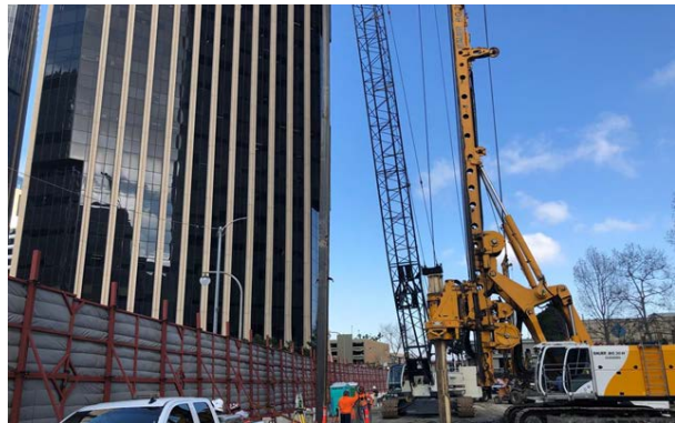
Soldier Pile Installation in Century City
