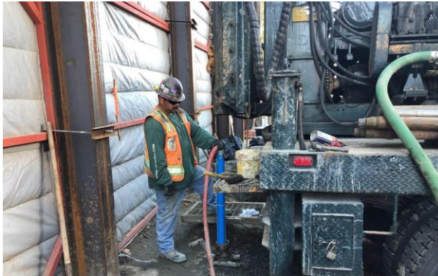
Grouting of Inclinator Casing
