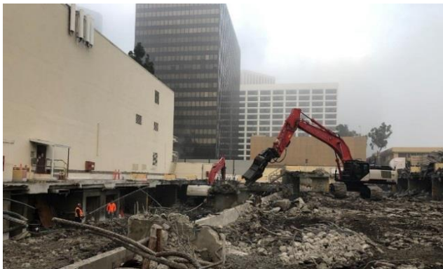
2010 Century Park East AT&T Parking Structure Demolition
