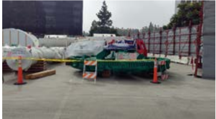
Tunnel Boring Machine (TBM) Delivery
