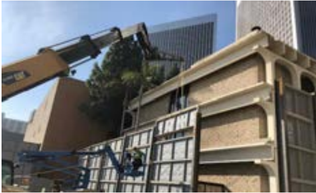
1940 Century Park East (CPE) Sound Wall Panel Installation
