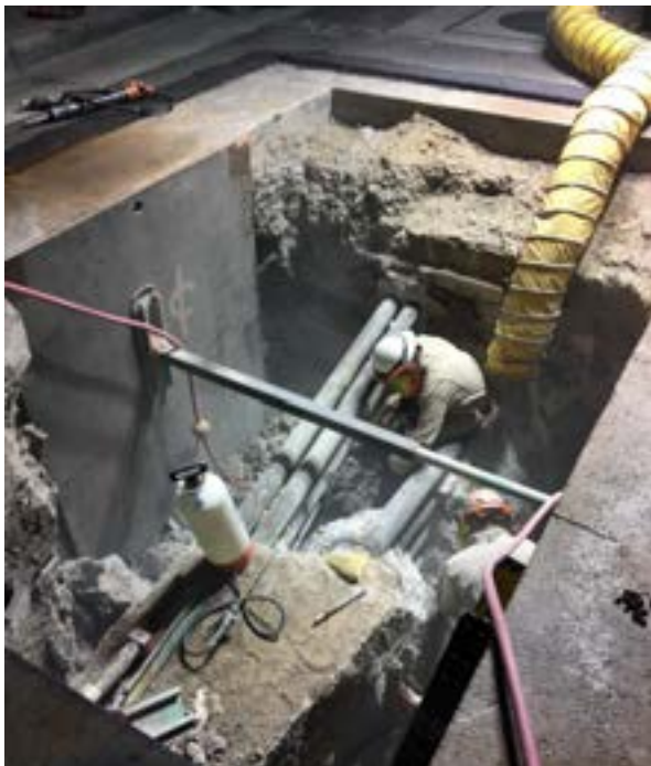
DWP Power Ductbank in Century City
