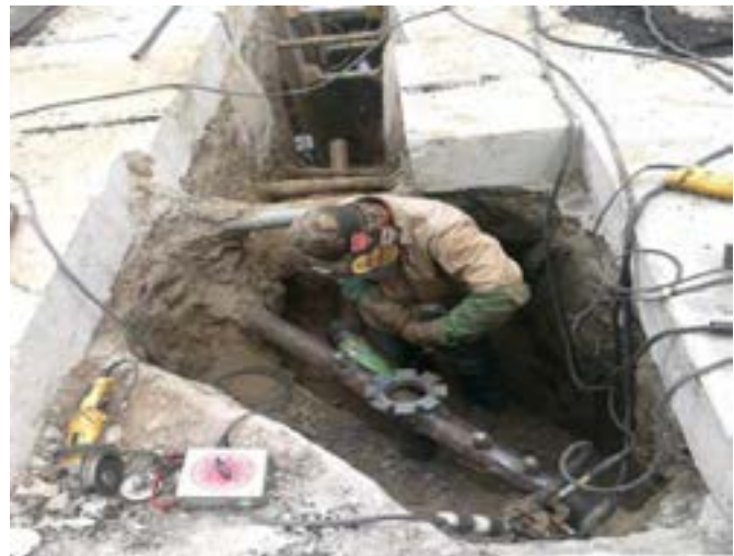
SCG Pipe Placement in Beverly Hills
