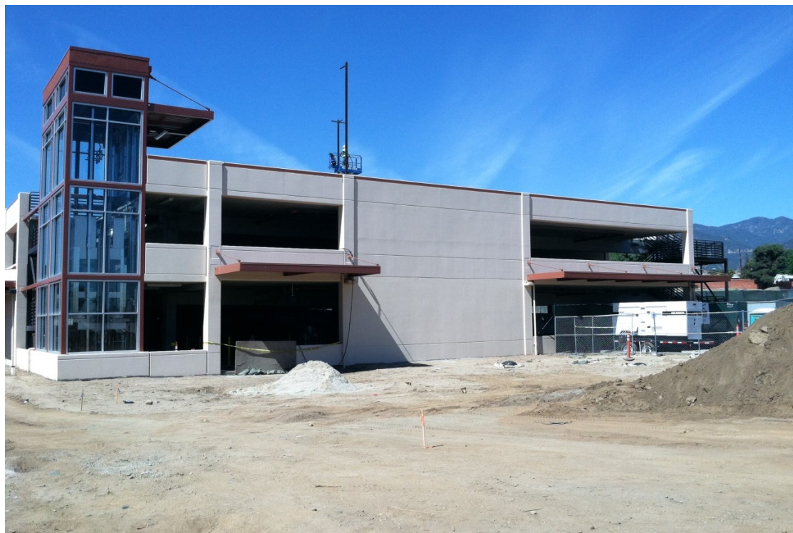
Monrovia Parking Structure Site Overview
