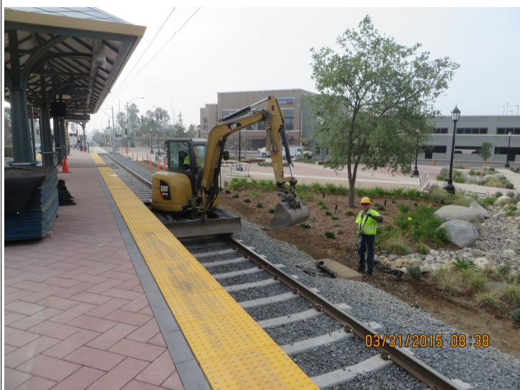
Segment 2: Arcadia Station - Grading Work
