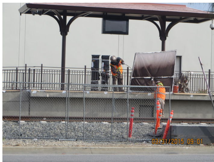
Segment 3: Duarte Station - Guardrail Painting
