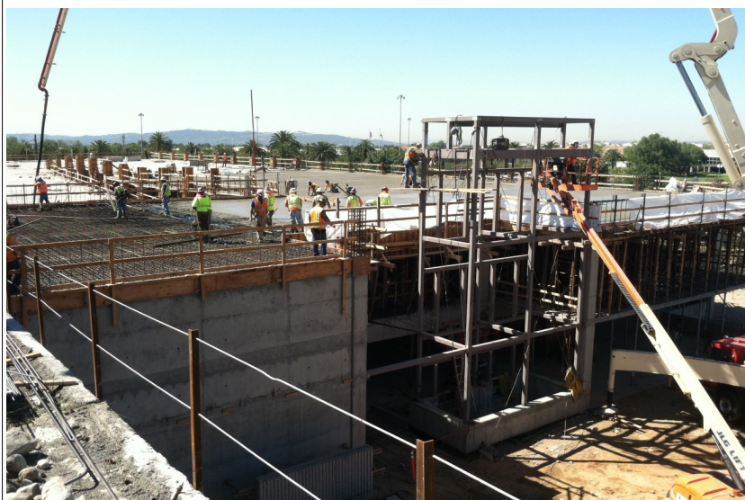
Irwindale Parking Structure Site Overview
