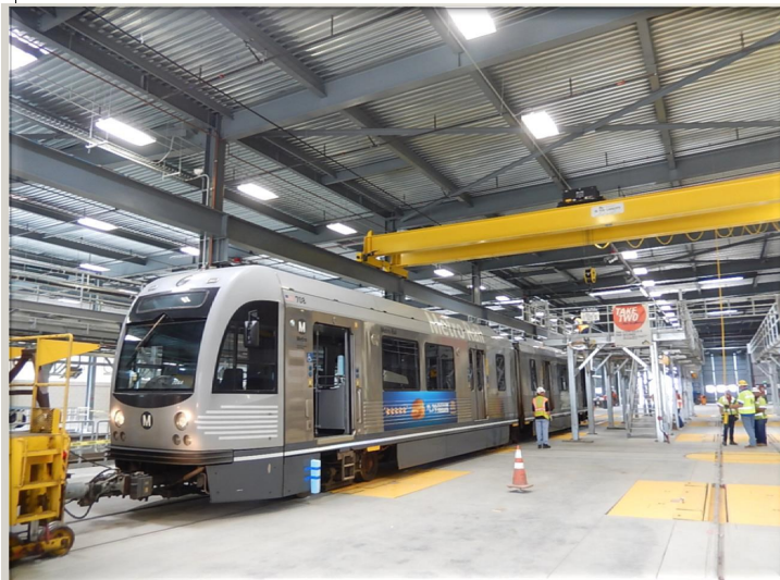
Operations Campus: First Vehicle in Building
