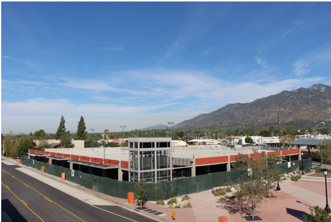
Arcadia Parking Structure Site Overview
