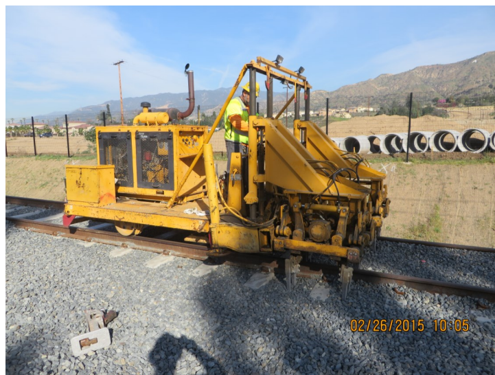
Segment 4: Citrus to Barranca - Track Surfacing
