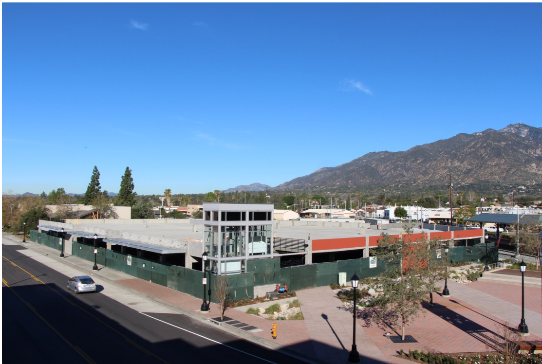
Arcadia Parking Structure Site Overview
