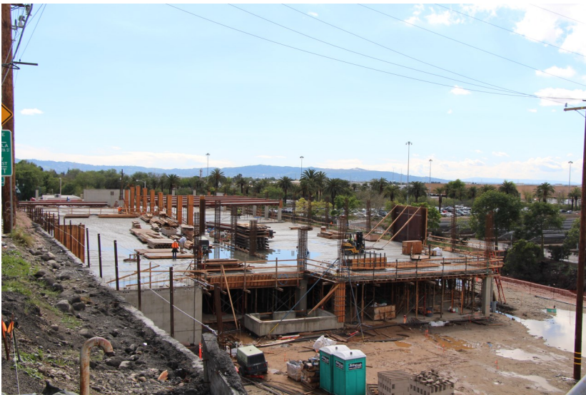
Irwindale Parking Structure Site Overview
