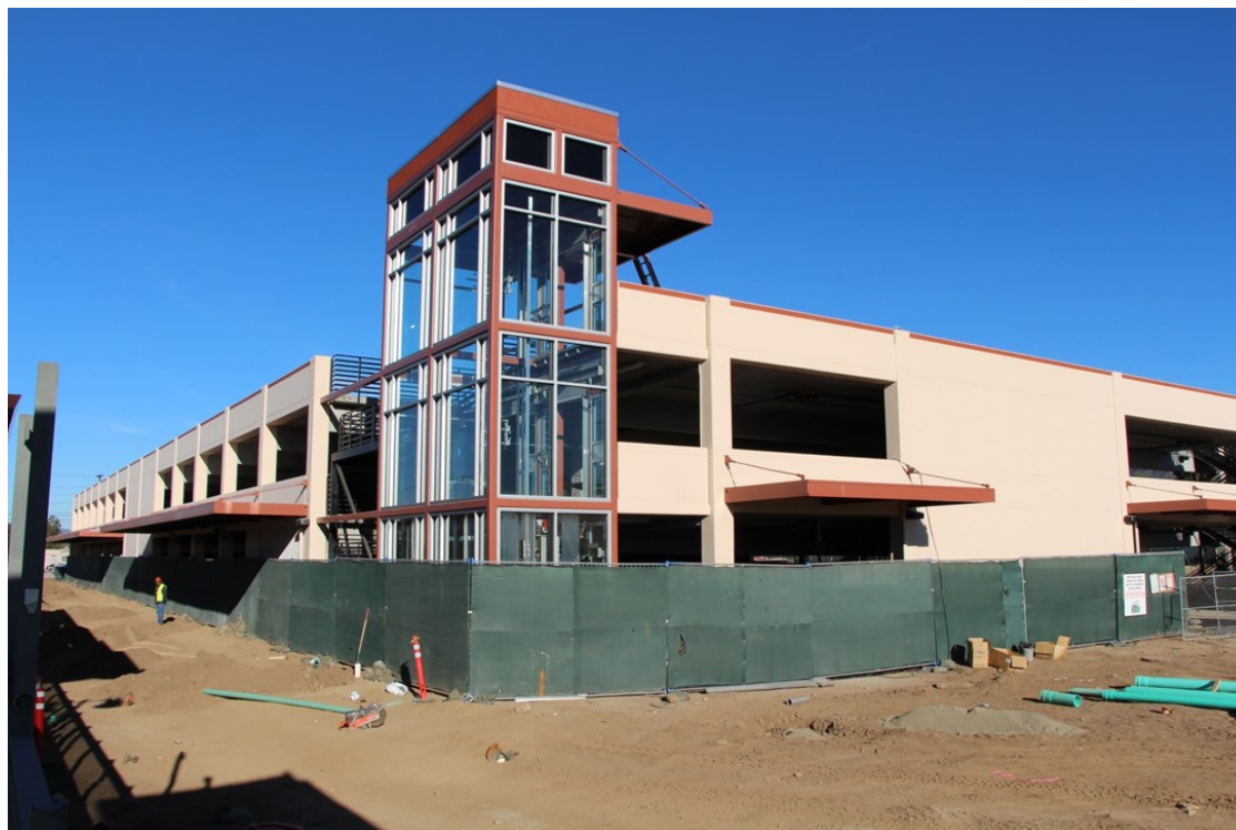
Monrovia Parking Structure Site Overview
