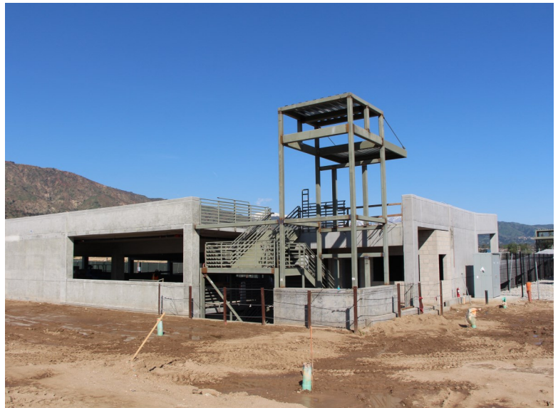
Azusa-Citrus Parking Structure Site Overview
