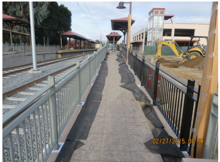
Segment 3: Monrovia Station - Guardrail Painting
