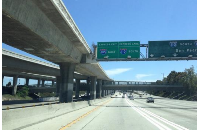
Figure 13: Photo of Existing I-110/I-105 HOV/HOT Direct Connectors
