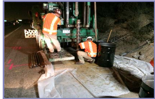
Drilling for a Soil Boring
