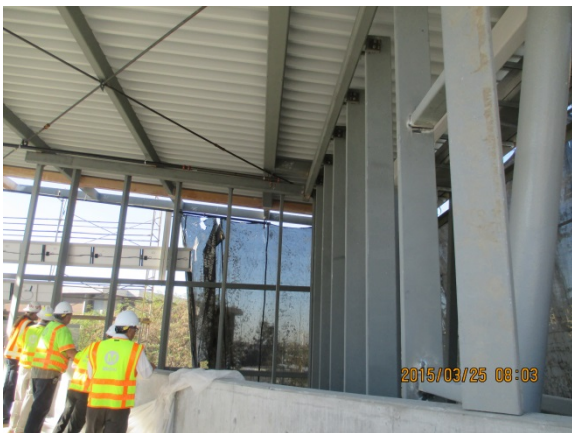
PV panels, Elevated Deck & Steel Artwork installed SW Corner.
