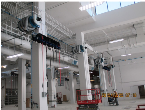
Painting application at Maintenance Building completed.
