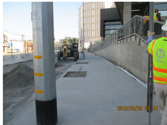
Ramp and Wire Mesh Fence installed at Transportation Building.
