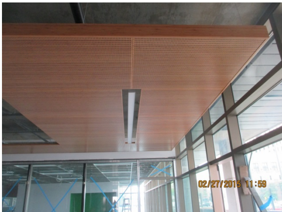
Installation of Bamboo Ceiling Finish Bldg. A Level 1.
