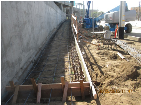
Reinforced framed for Ramp and earthwork along Vignes St.
