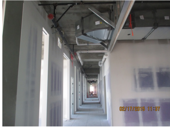
Walls finishing process at Bldg. A Level 2.
