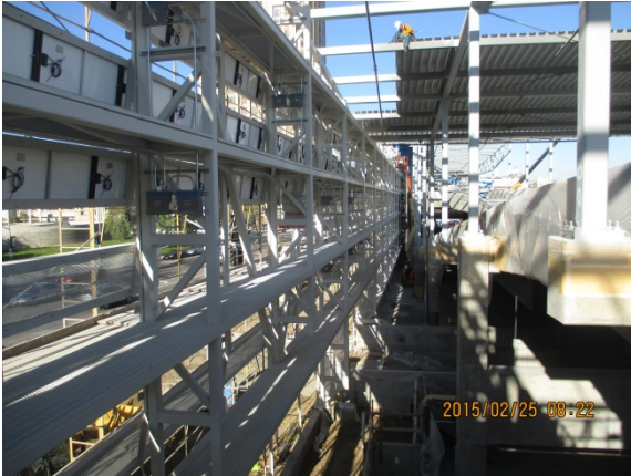
PV Panels Installation at Parking Garage Structure.
