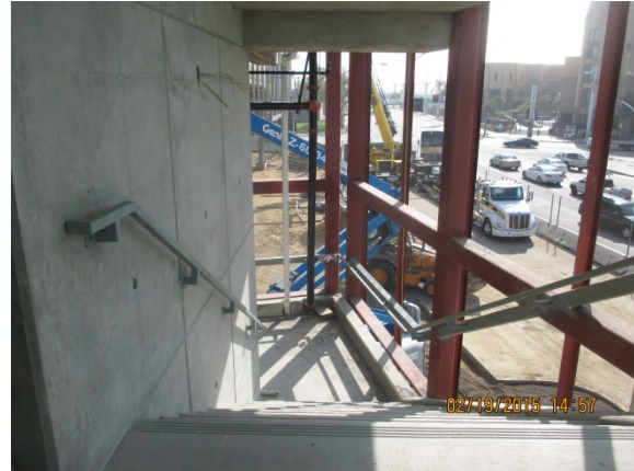
Handrails installed; welding on Red Steel members at Bldg. A.
