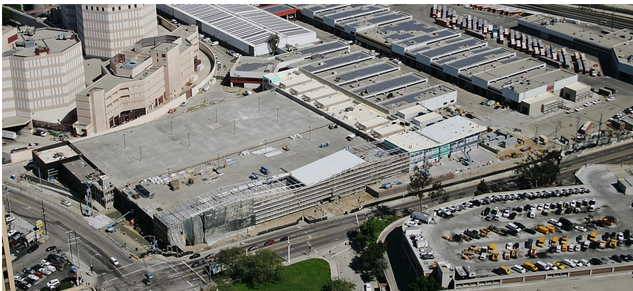
Transportation Building, Parking Garage and Maintenance Building in construction; at the bottom side Cesar Chavez Avenue and at the left side Vignes Street.
