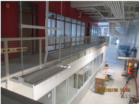
Welded wire mesh fence complete at Maint. Building Level 2.
