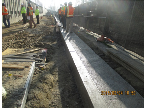
Curb Gutter Completed along Cesar Chavez Ave.
