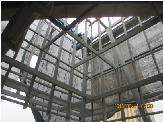
Structural Steel Frame for Artwork Completed at SW corner.
