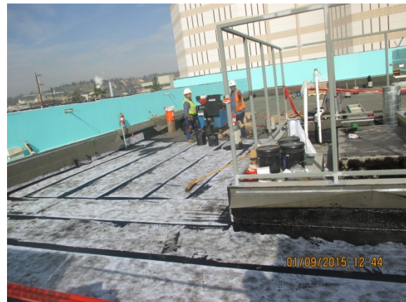
Membrane roof installation at the Transportation Bldg.
