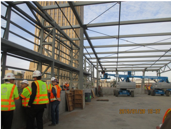
Installation of steel roof ribbon in progress at Parking Garage.
