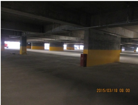
Paint application completed at Parking Garage Lower Level.
