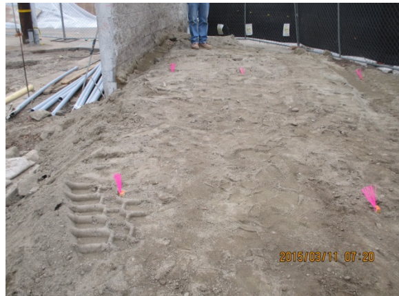
Elevation and Earthwork for Ramp access at Utility Yard.
