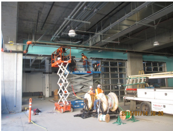
Pulling electrical feeders at the electrical panels in Parking.
