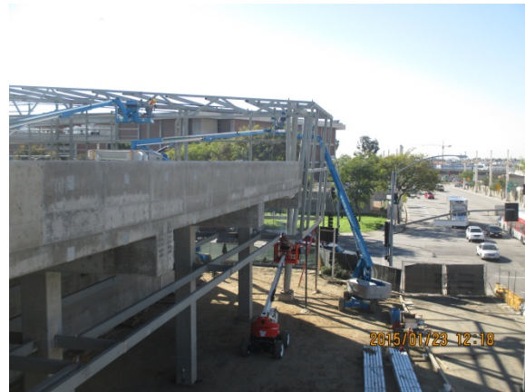
Installation of horizontal beams at the roof deck in progress.
