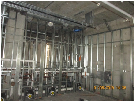
Interior metal stud framing at restroom in Transp. Bldg. 1 Level.
