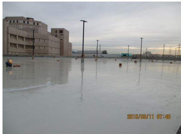
Polycoat Catalyst application at Parking Garage Upper Level.
