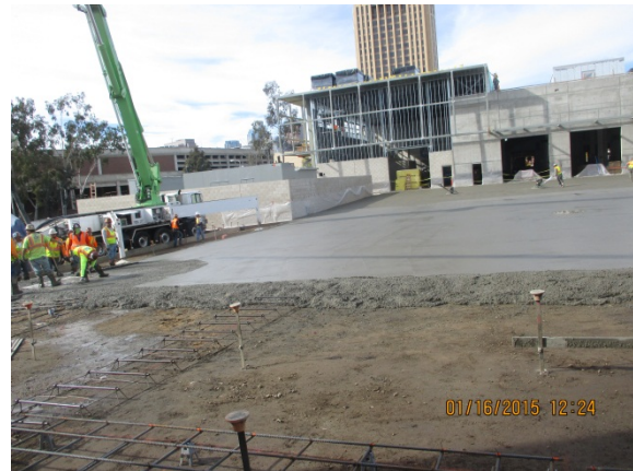
Concrete pouring in progress at East side of Utility Yard.
