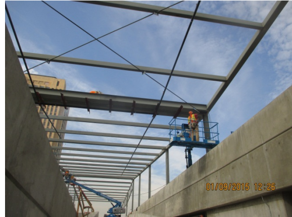
Installation of metal roof panels at the Roof Ribbon Parking.
