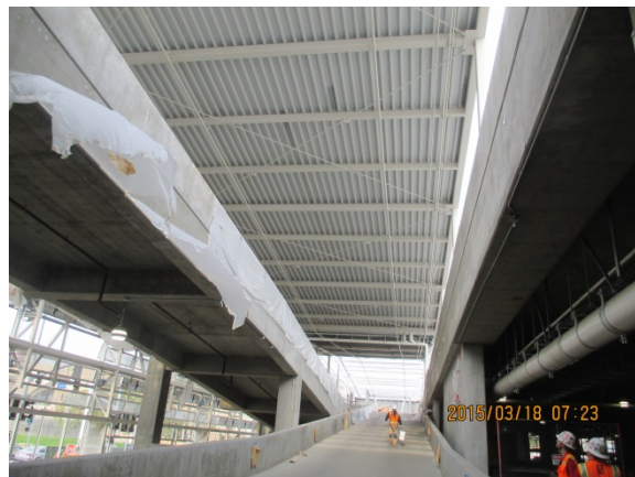
Elevated Roof Deck installed at Parking Garage Upper Level.
