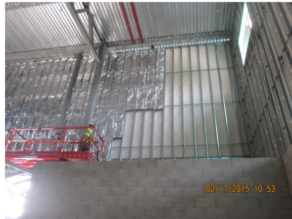
Insolation Installation at Maintenance Bldg.
