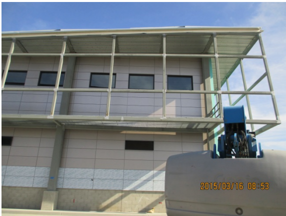
Architectural panels completely installed at Maintenance Bldg.
