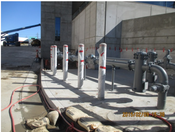
Bollards installation at Metro Driveway/ Vignes St Curb.
