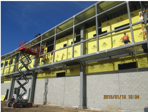
Installation of sheet rock at the exterior walls of Bldg. C.
