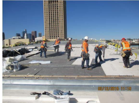
Insolation Installation at Roof of Maintenance Bldg.
