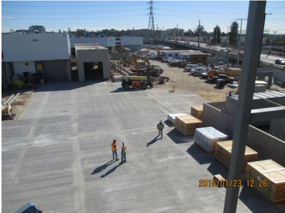
View of finished concrete at the CFM and Maintenance Bldg.
