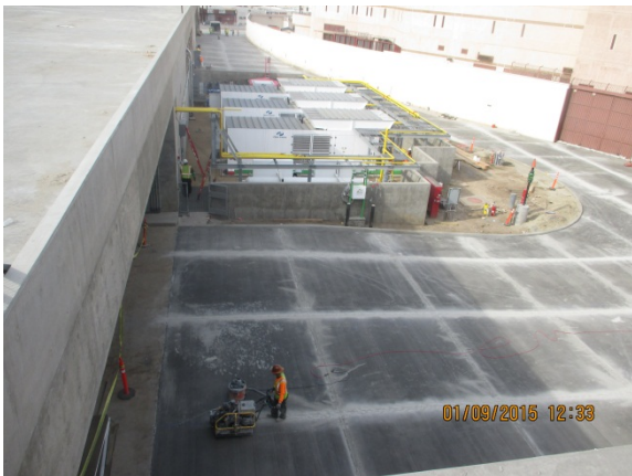
Saw cutting new concrete joints at Metro Drive Way.
