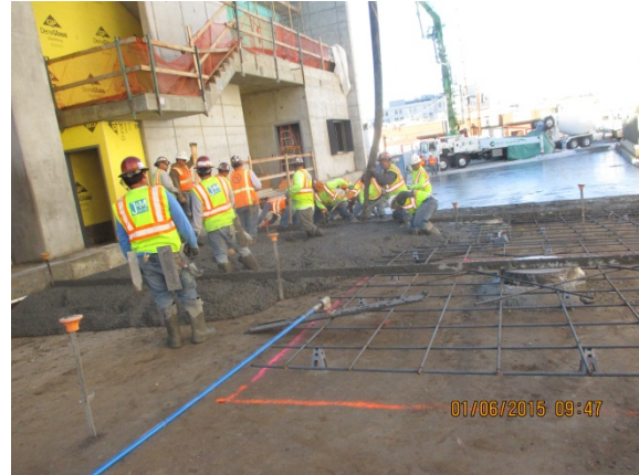
Placement of concrete along Metro Drive Way.
