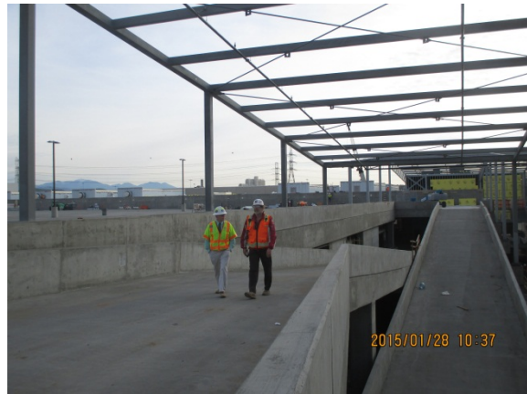
View of roof ribbon system at the roof deck Parking Garage.
