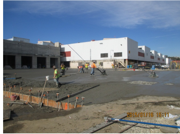
Concrete finishing at the West side of C Building.
