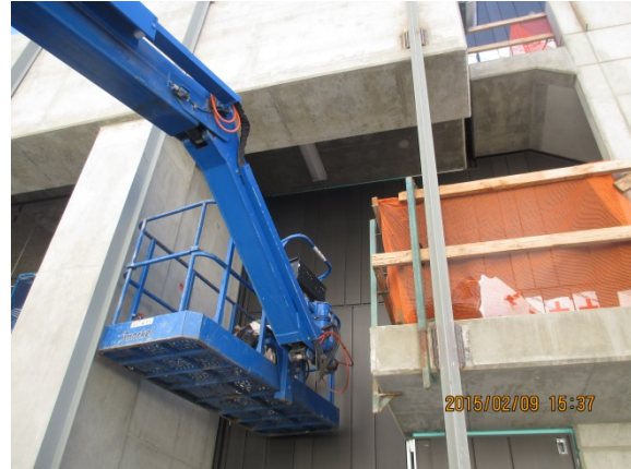
Zinc Interlock wall panel system installation. North of Bldg. A . .
