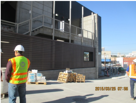
Perforated Zinc Wall installed at Transportation Bldg. Level 1.
