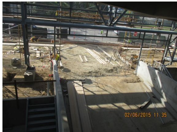
Curb & Sidewalk wood framing at Lyon St Garage entrance.
