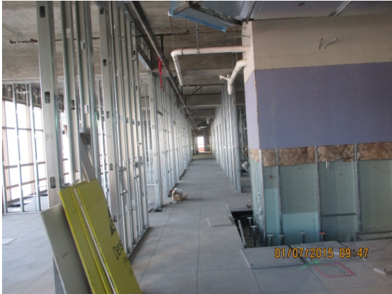
Interior metal framing at Transportation Bldg. Level 1.
