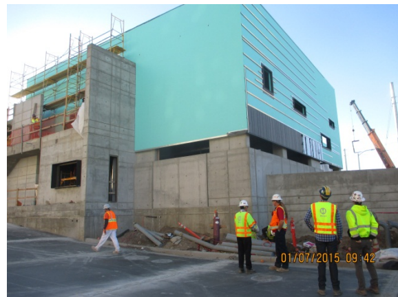
Installation of zinc panels at exterior of Transp. Bldg.
