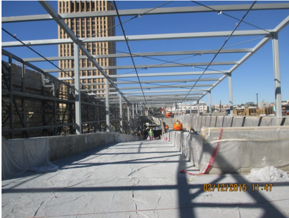
Painting Frame phase. Parking Garage Roof Framing.
