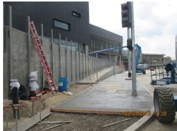
Ramps finished & cement curing on sidewalk along Vignes St.
