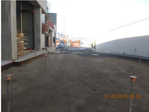
Placement of steel reinforcement along Metro Drive Way.
