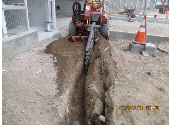
Opening Trench for sidewalk concrete pouring Lyon St entrance.
