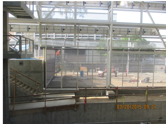
Horizontal Steel members and perforated wall installed Parking Building.
