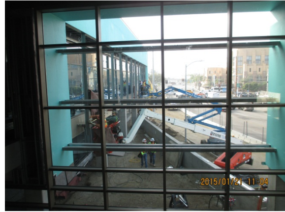
Installation of curtain wall glazing in progress at Building A.
