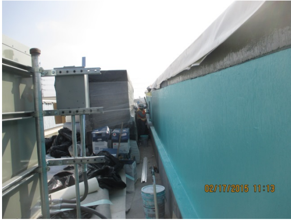
Water protection application at Roof of Maintenance Bldg.
