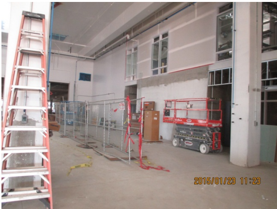
Interior painting in progress at Maintenance Building.
