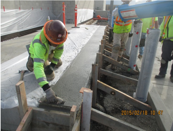
Concrete Pouring at Above Ground Fuel Slab.
