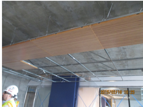
Installation of Bamboo ceiling in Bldg. A Level 1.
