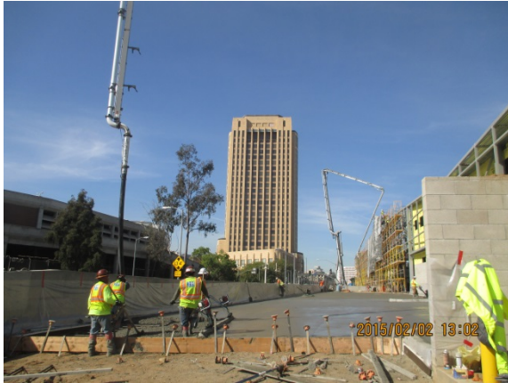
Placement of concrete along Parking Walkway.
