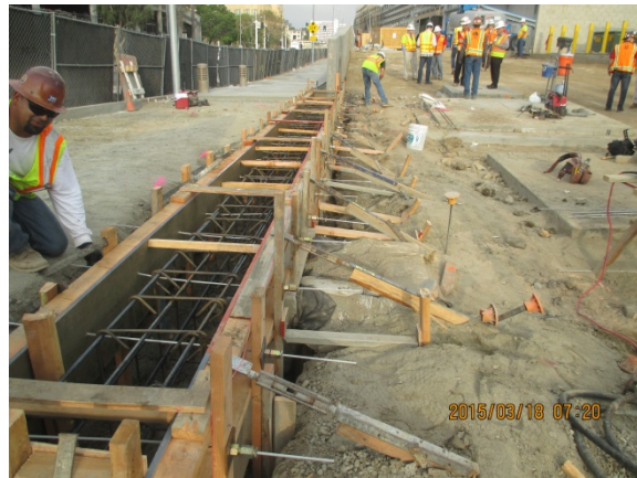
Prep and forming CMU Wall for Utility Yard Area.
