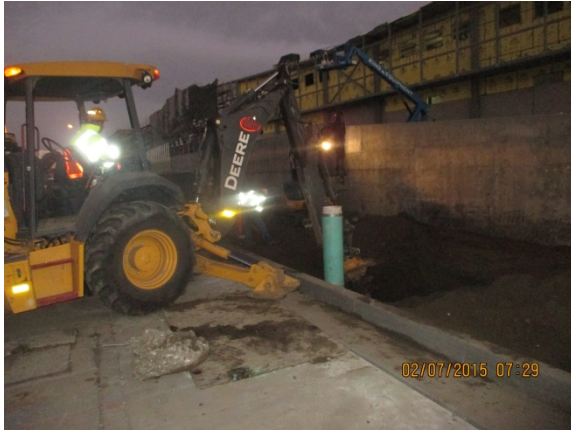
Relocating vent of electrical vaults at Cesar Chavez Ave.
