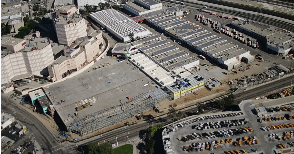
Transportation Building, Parking Garage and Maintenance Building in construction; at the bottom side Cesar Chavez Avenue and at the left side Vignes Street.
