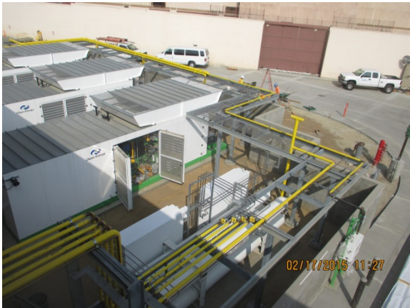
CNG Yard completed pipe installation.
