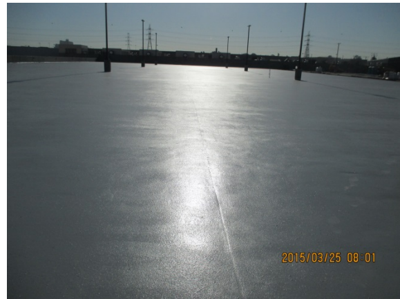
Parking Garg Upper Level, 3 weeks after application of Polycoat.
