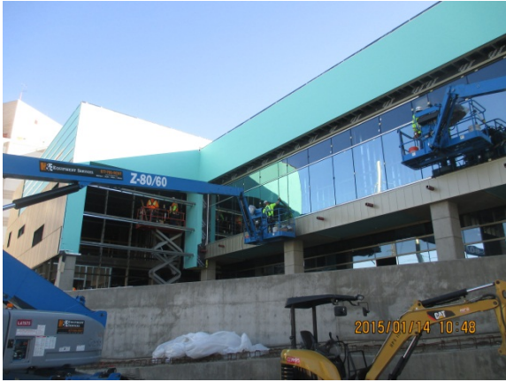
View of the exterior curtain wall at the Transportation Bldg.
