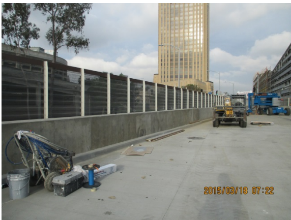
Perforated Zinc Screen Wall installed at Div. 13 South Elevation.
