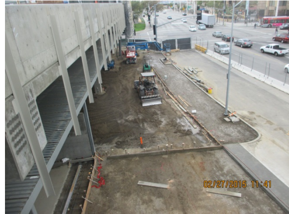
Pour of concrete in progress on front of Vignes St.
