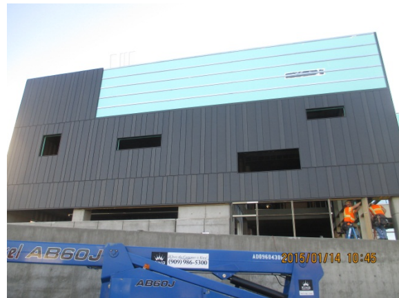
Installation of zinc panels at exterior of Transportation Bldg.
