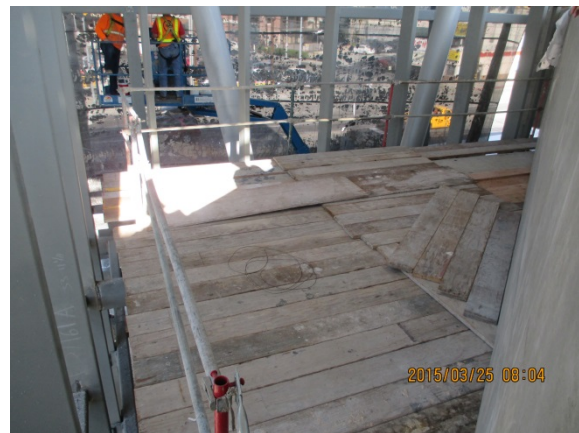
Dancefloor scaffolding ready for installation of Artwork Panels & bird deterrents.
