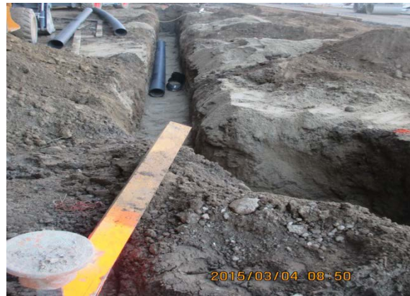
Open trench for piping at Vignes St. entrance.
