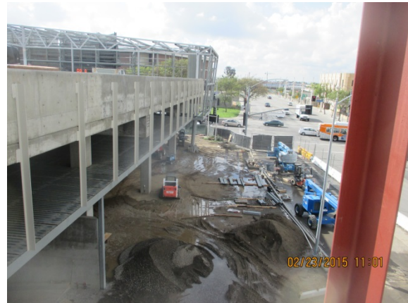
Vertical Steel members installed & earthwork at Garage Prkg.
