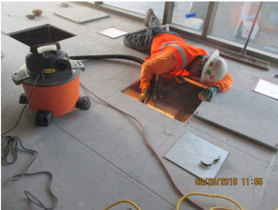
Under floor work under progress at Level 1 of Bldg. A.
