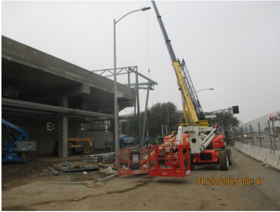
Installation of steel column members for the roof progress.
