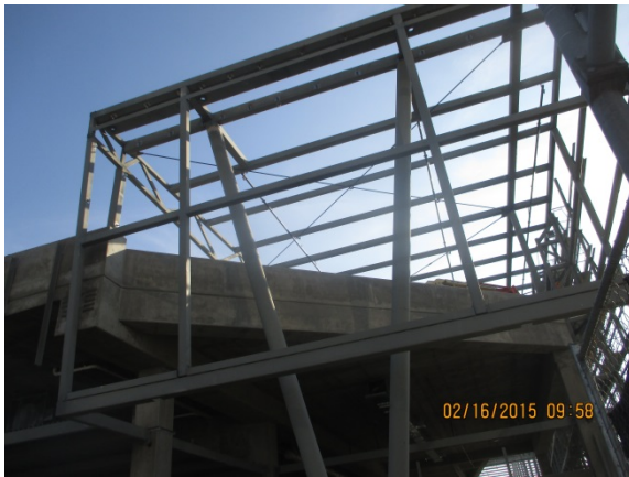
Installation of steel membranes of Roof Deck in progress.
