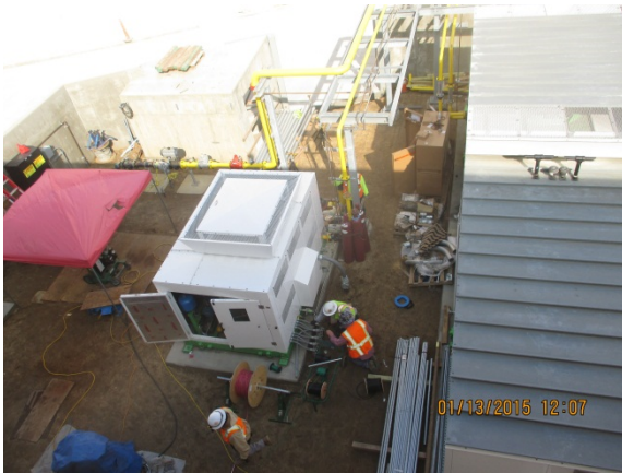
Wiring pulling at the CNG Yard equipment service.
