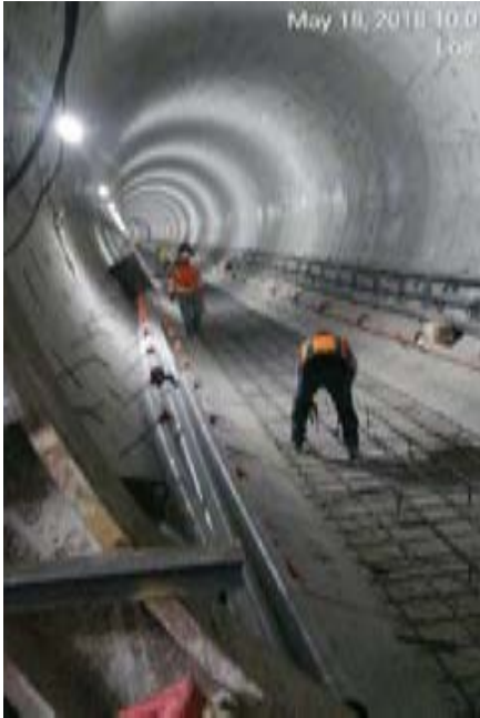
Invert rebar mat, in right tunnel from Central to Broadway
