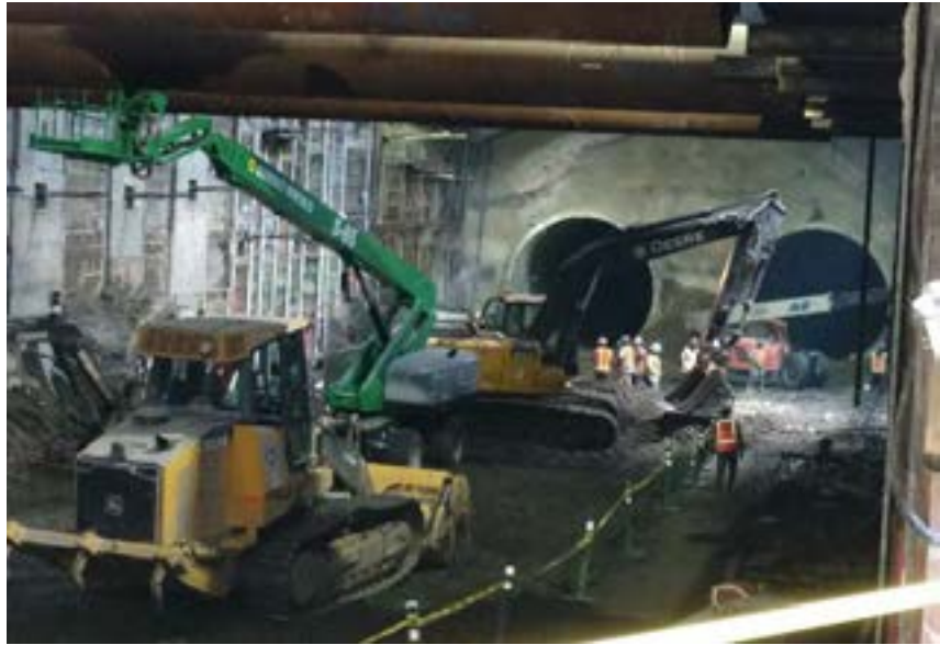
Sequential Excavation Method (SEM) underway at Historic Broadway Station
