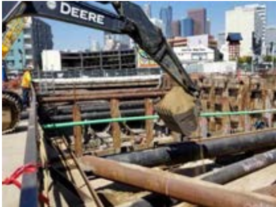
Station excavation resumed at 1st/Central
