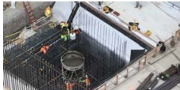
Invert pour in east sump in Grand Av Arts/Bunker Hill Station
