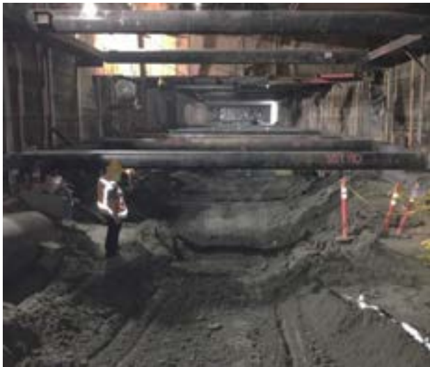
North access shaft excavation and mucking operations at Flower
