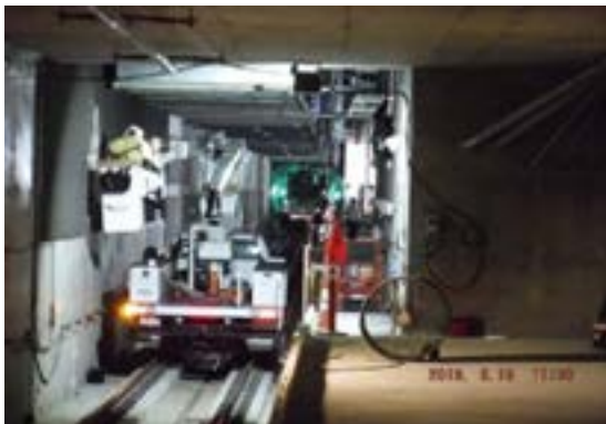
UG4 – Systems installation work looking north toward Leimert Park Station.
