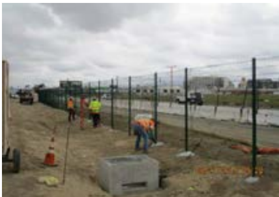
GUIDEWAY BETWEEN UG1 AND 104 TH ST. – Installing wire fence.
