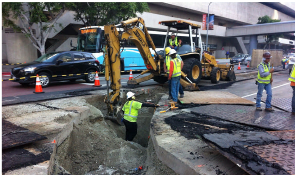
DWP Power trench excavation at the intersection of Flower Street and 5 th
