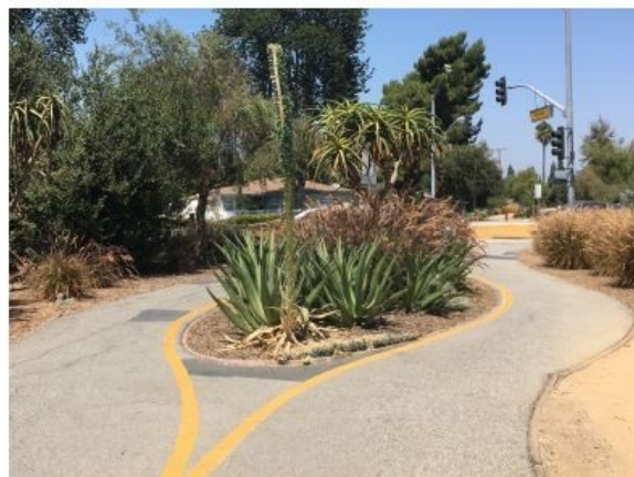
Example of diverter island that alert cyclists to upcoming intersection (Whittier Greenway Trail)
