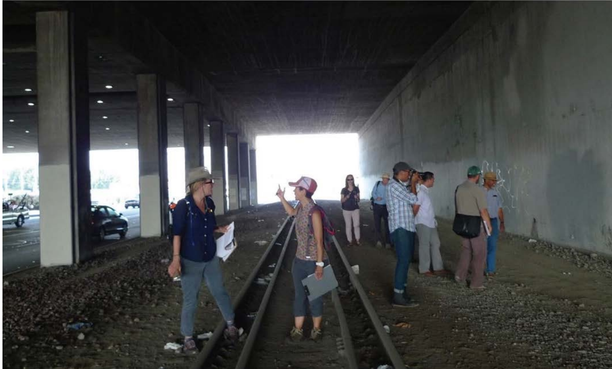
Before photo of Metro ROW at 110 Freeway Underpass looking West
