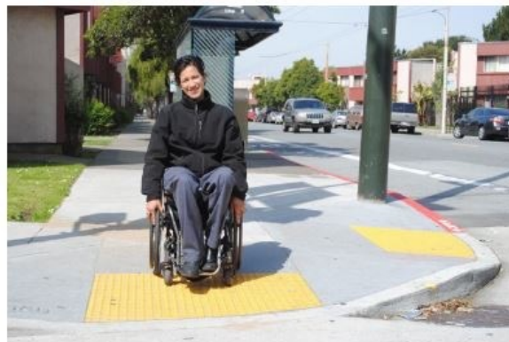
Directional curb ramps with tactile warning strips
