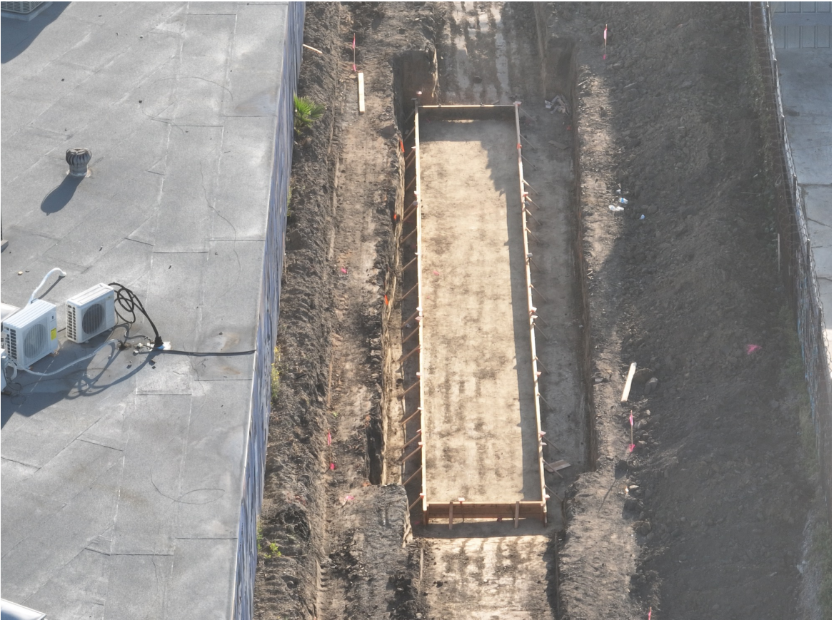
Construction of storm water management
