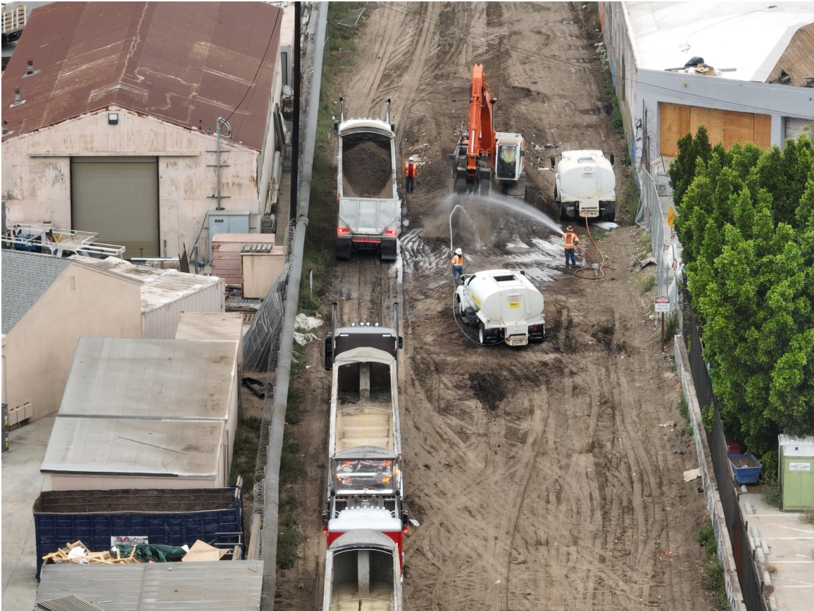
End of 10th Street, dust mitigation and material hauling
