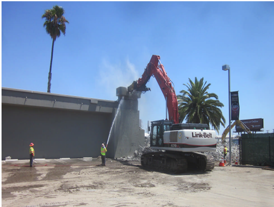
Century bridge north abutment demolition at 9 a.m. on July 26 th .
