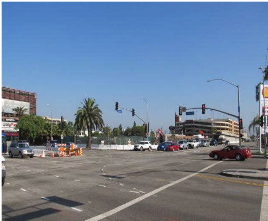
Century Blvd and Aviation after the bridge demolition.
