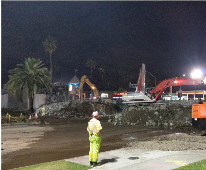
Century bridge demolition progress at 10 p.m. on July 26 th .
