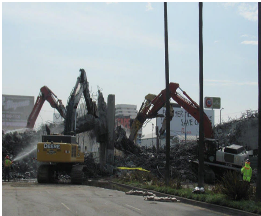
Century bridge demolition at 9 a.m. on July 26 th .
