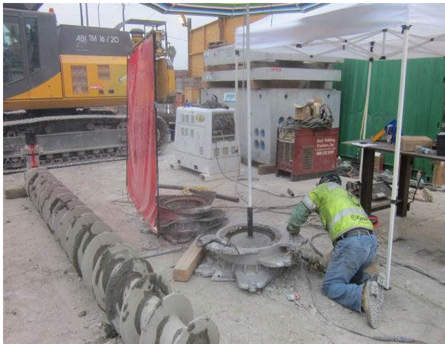
Cutter soil mixing wheels at the Exposition Station Yard.
