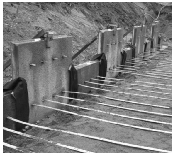
Figure 18. MSE Wall Construction (© Reinforced Earth)
