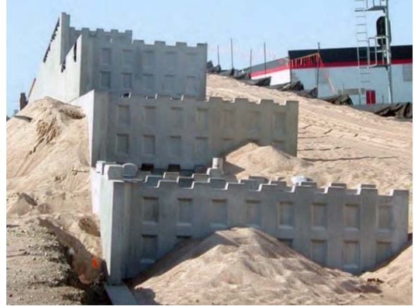
Figure 19. T-WALL® Construction (© Neel Company)
