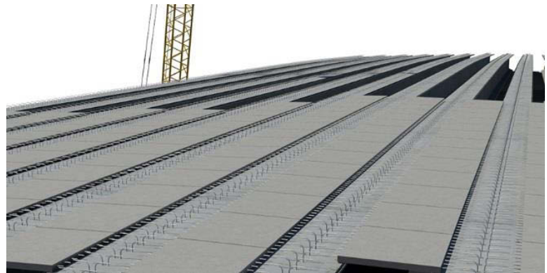
Figure 16. Precast Deck Panels
