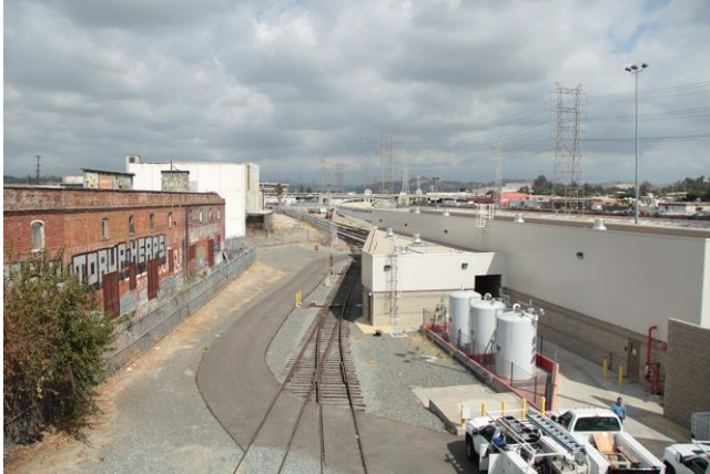
View of property, facing north from 1 st Street Bridge
