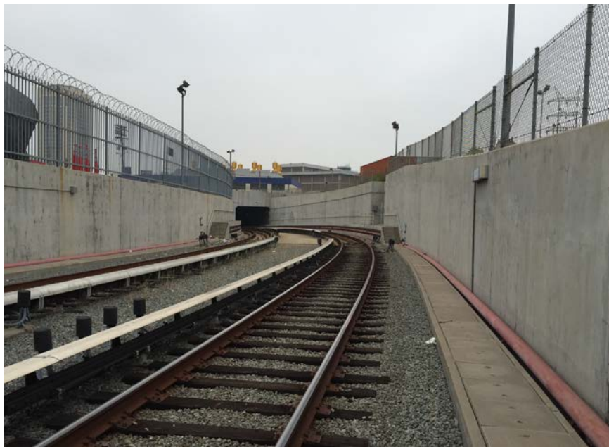
Existing heavy rail portal, south of U.S. Highway 101 freeway
