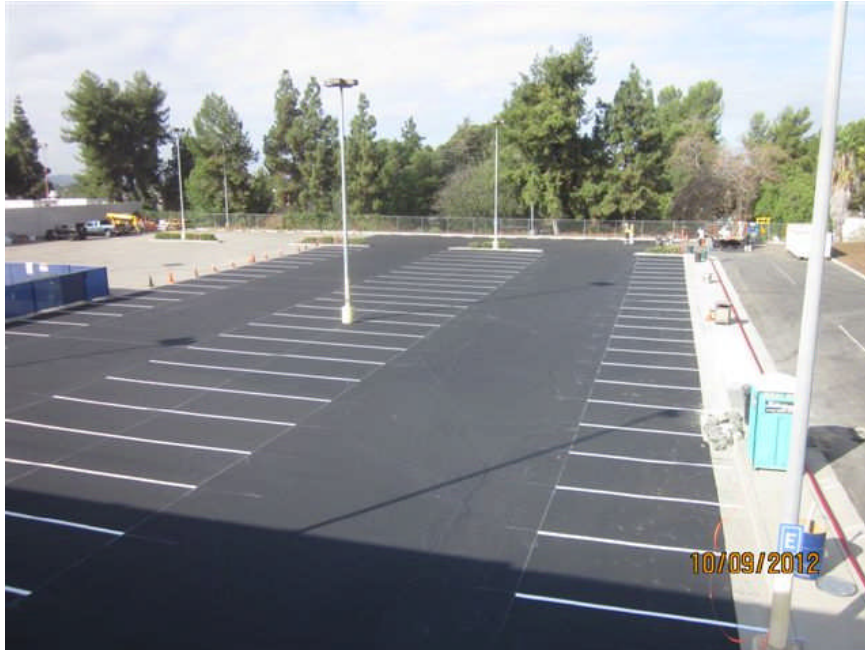
West parking lot striping.
