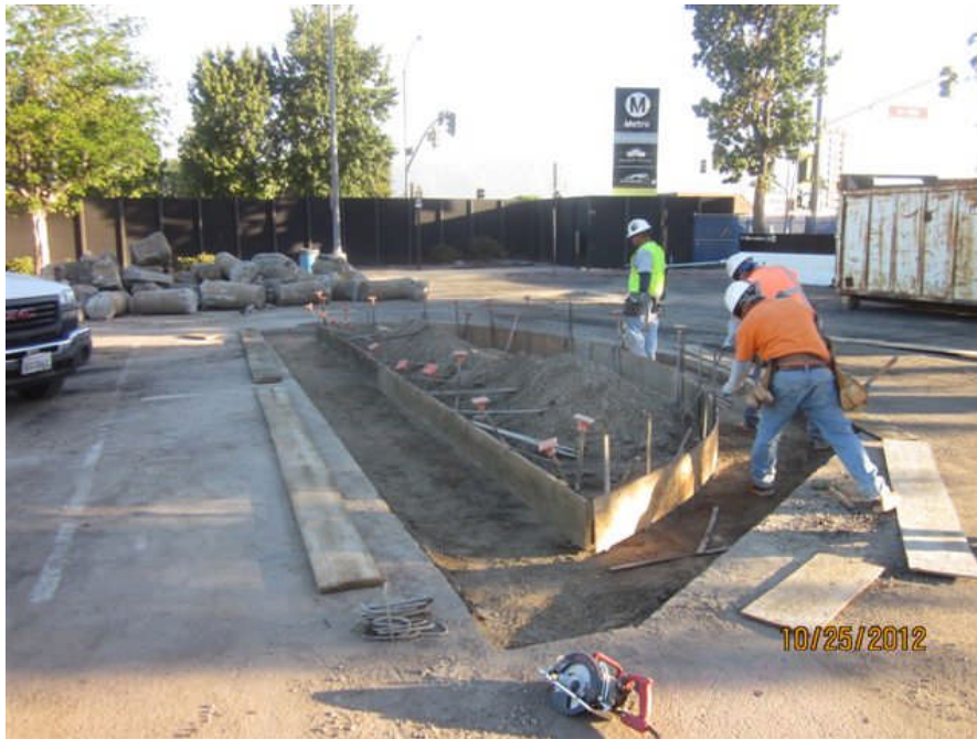
Forming islands in temp terminal.
