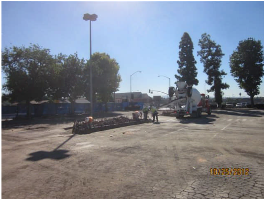
Placing concrete islands in the temp terminal.
