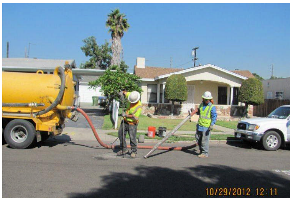
Crews locating utilities near 59 th Street.
