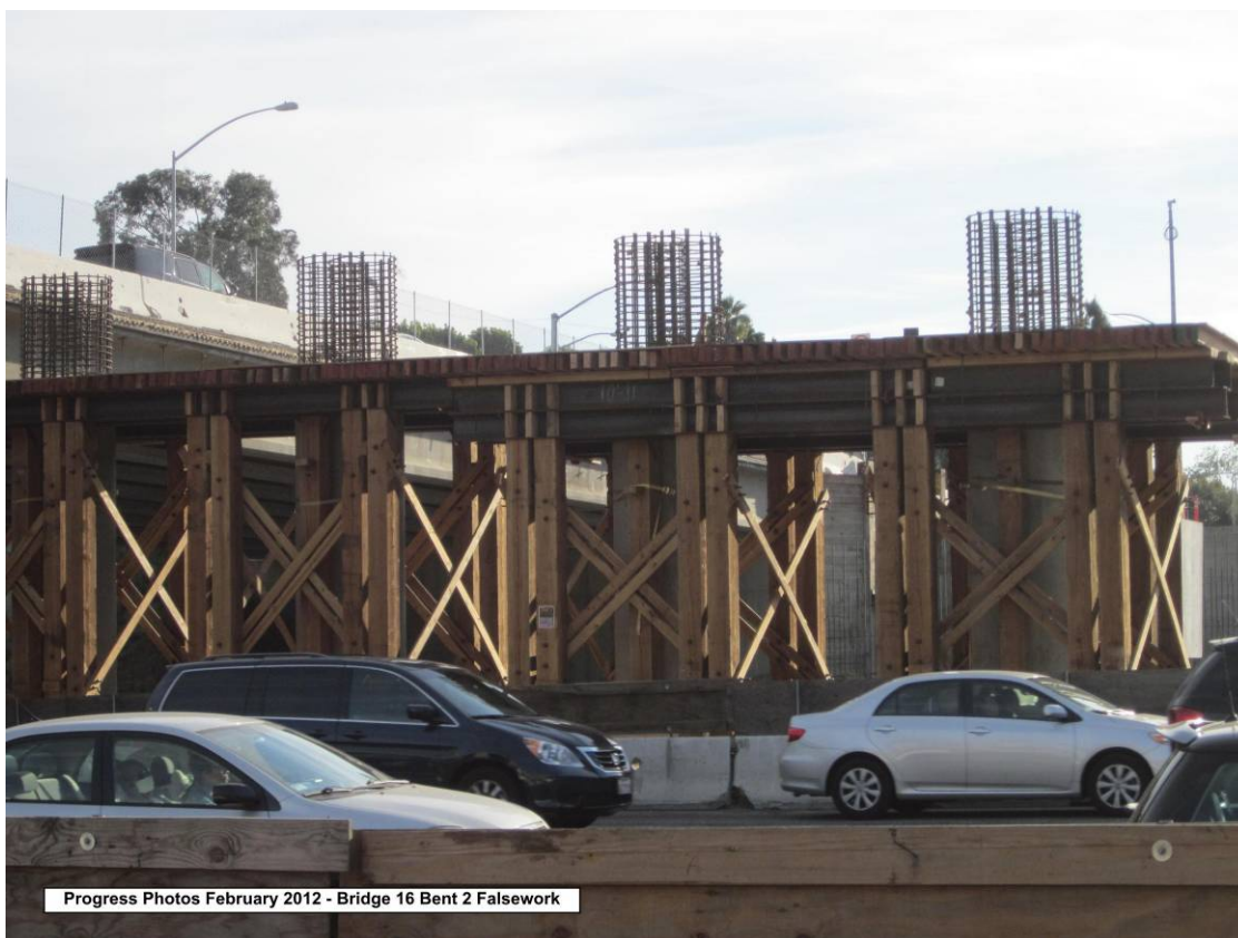
Bridge 16 Bent 2 Falsework.
