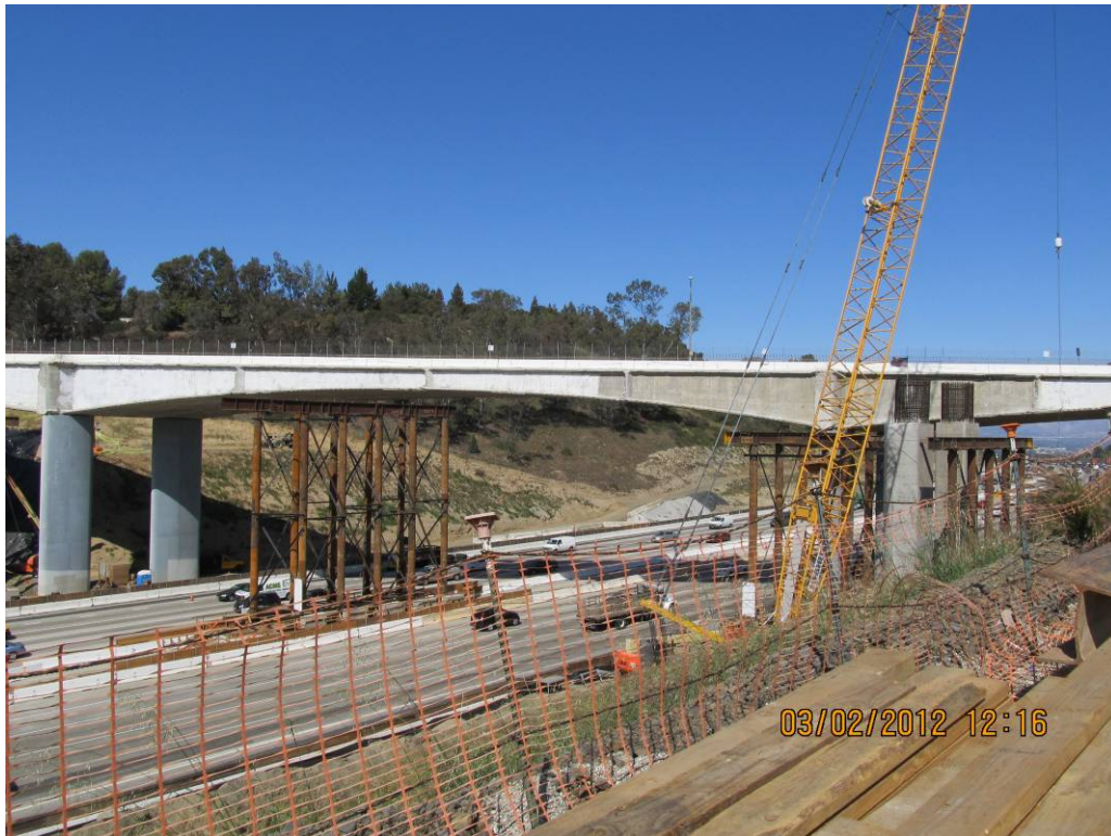
Mulholland Bridge falsework.
