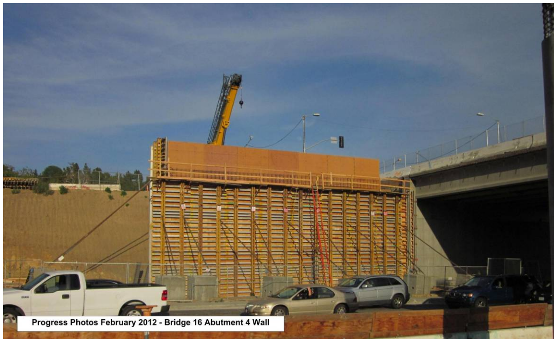
Bridge 16 Abutment 4 Wall.
