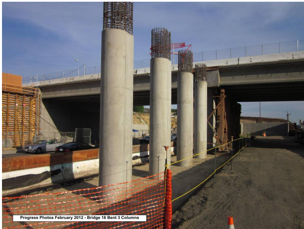
Bridge 16 Bent 3 columns.
