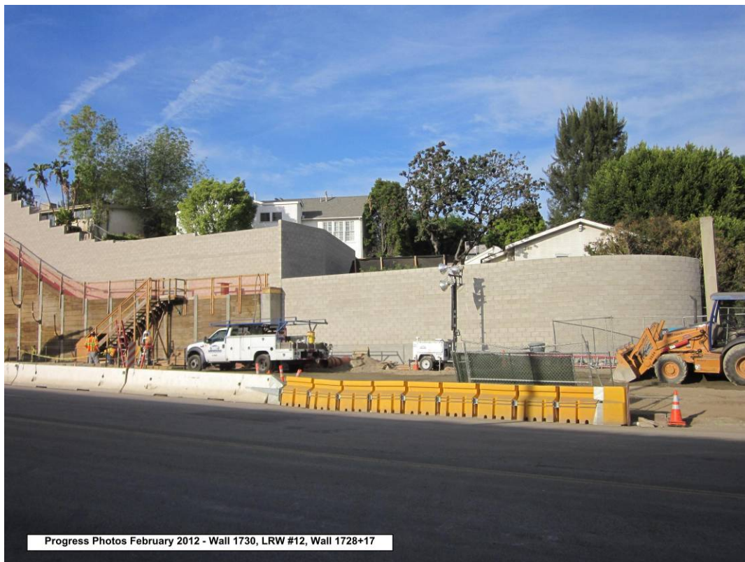
Wall 1730, LRW #12, Wall 1728+17.
