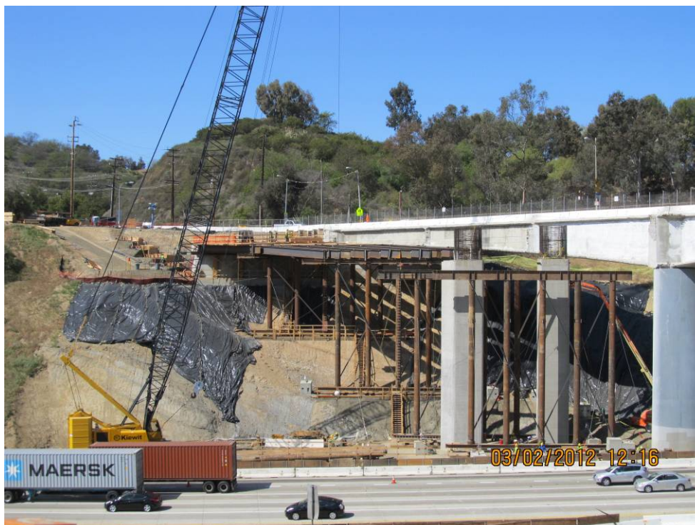
Mulholland Bridge falsework.
