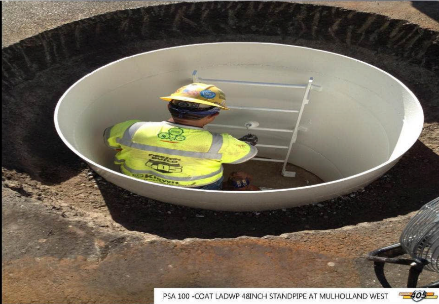
PSA 100 -COAT LADWP 48INCH STANDPIPE AT MULHOLLAND WEST
