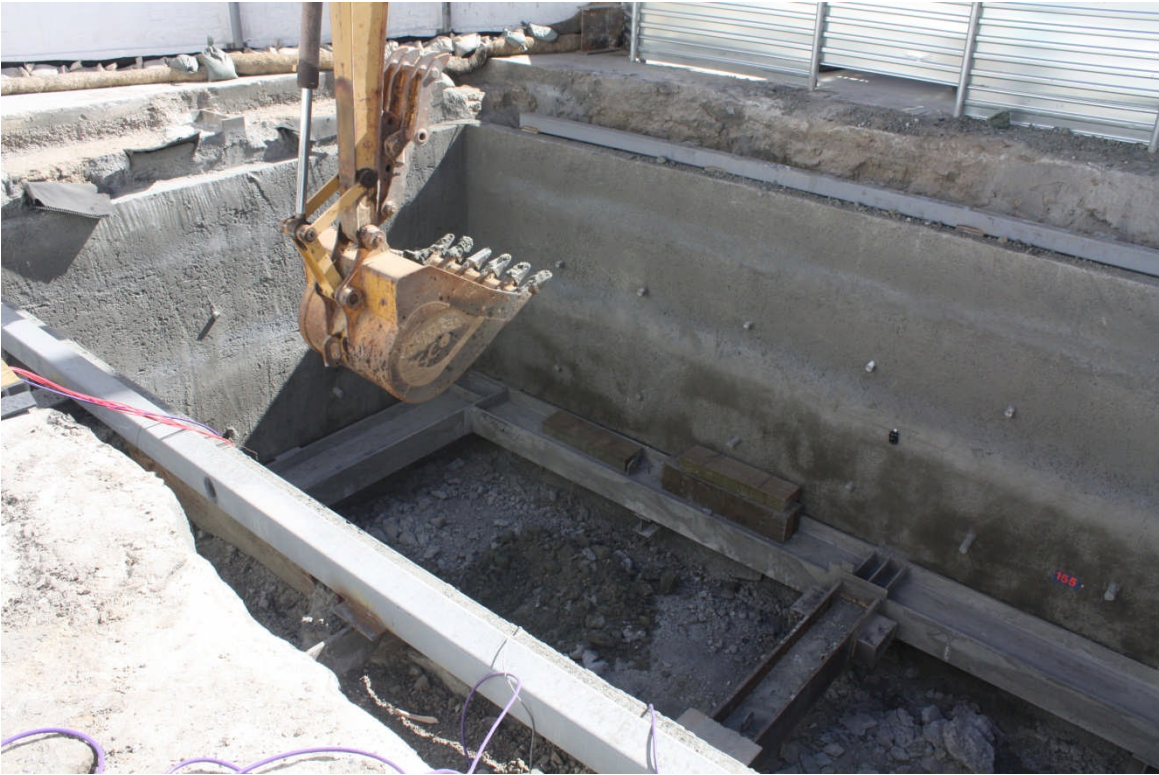
Excavation of the Exploratory Shaft
