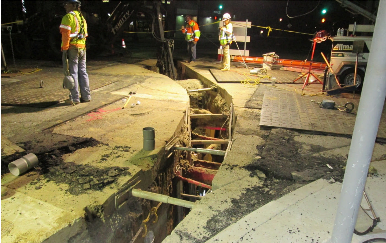
Placement of Utility Ducts by the C1048 (Wilshire/La Brea) Contractor
