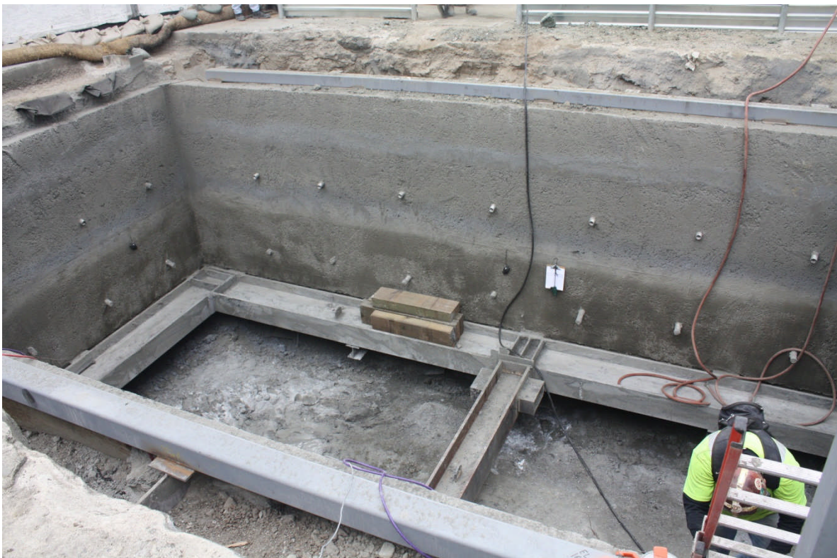
Exploratory Shaft East and South Walls with Shotcrete
