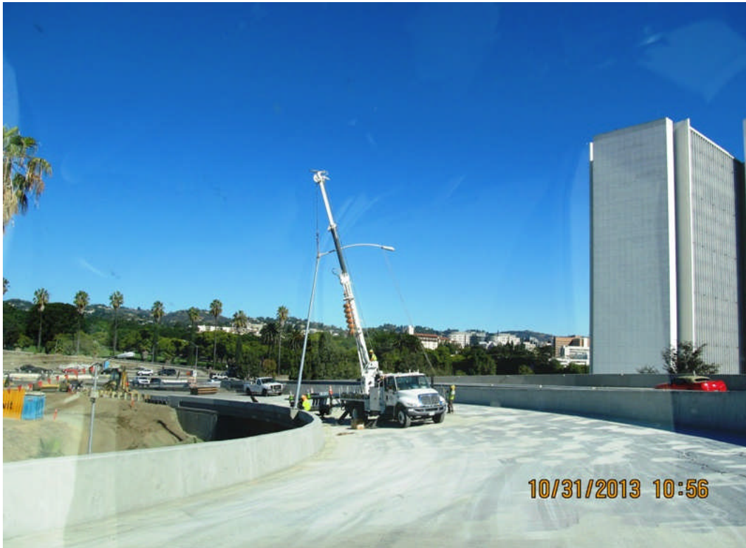
Bridge 8 - Top Deck and Barriers Poured; Light Installation.
