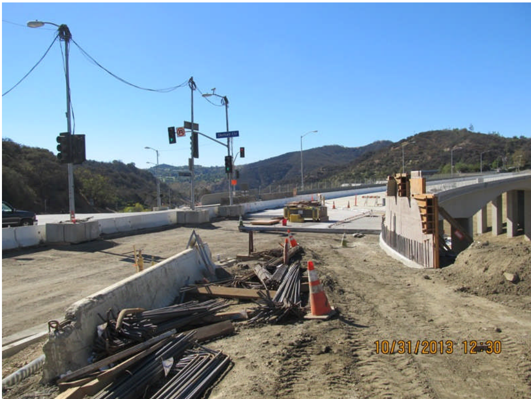
Bridge 22 Approach Slab Poured and Barrier Wing Wall Form Installation.
