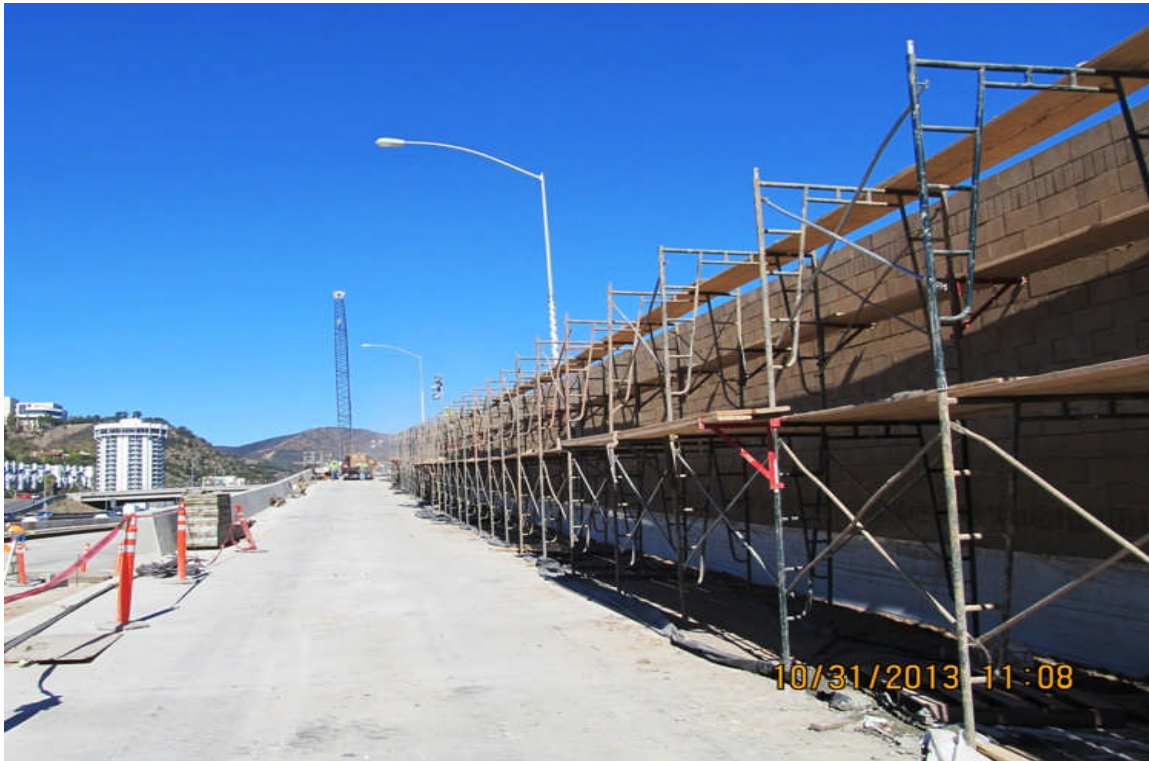
Wall 1718 Soundwall Construction.
