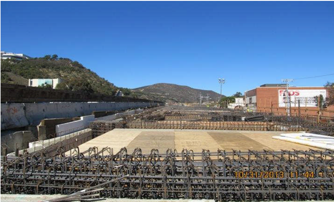
Bridge 17 Rebar Installation.
