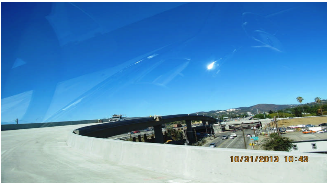
Bridge 8 Falsework Removed.
