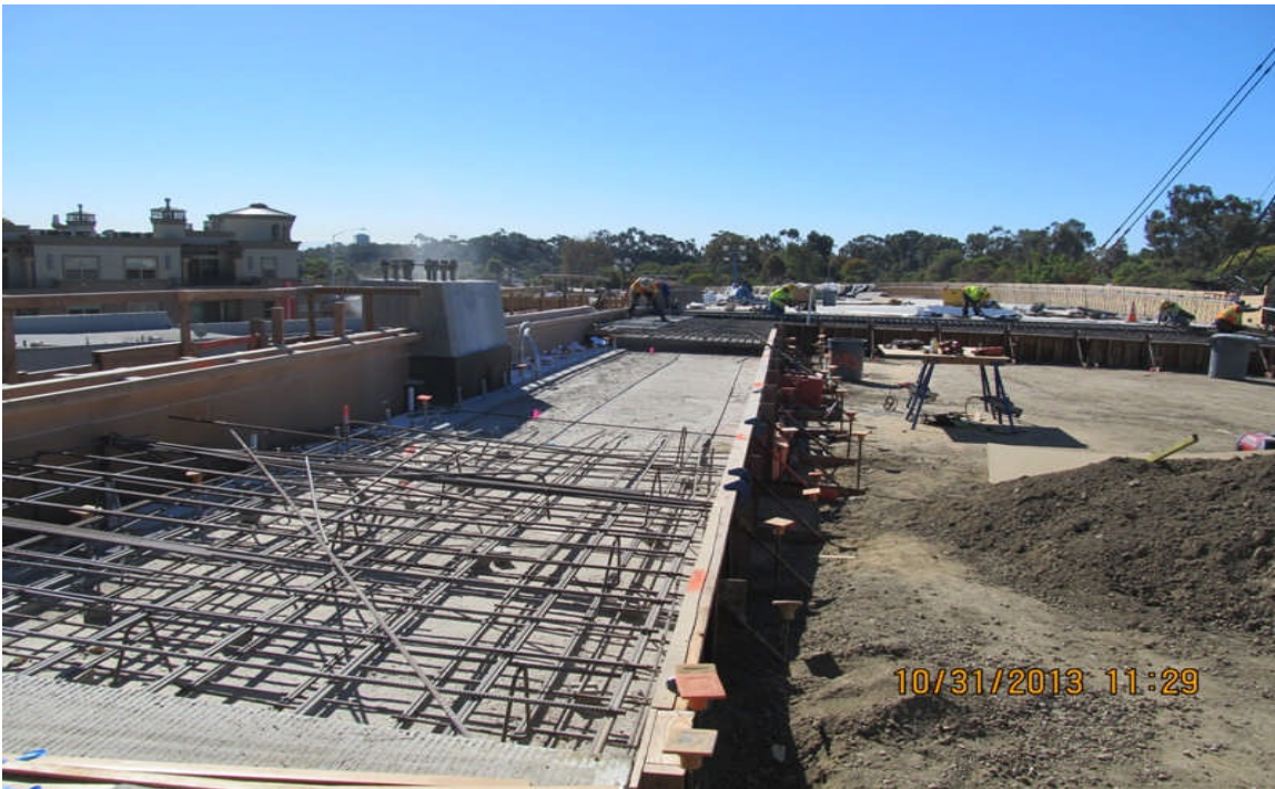
Bridge 14 Moment Slab Form and Rebar Installation.
