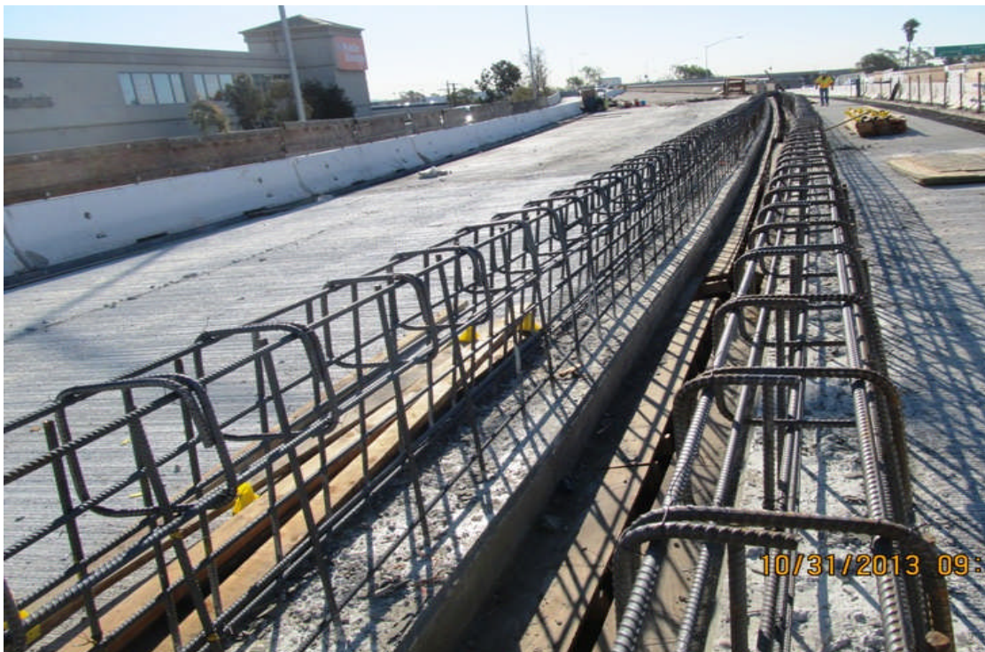
Bridge 2 Top Deck Poured and Barrier Rebar Installed.
