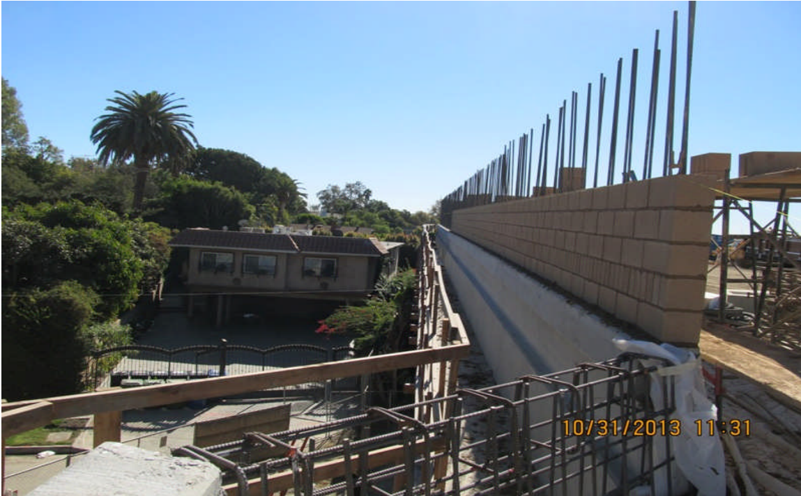
Wall 1738A Soundwall Construction.
