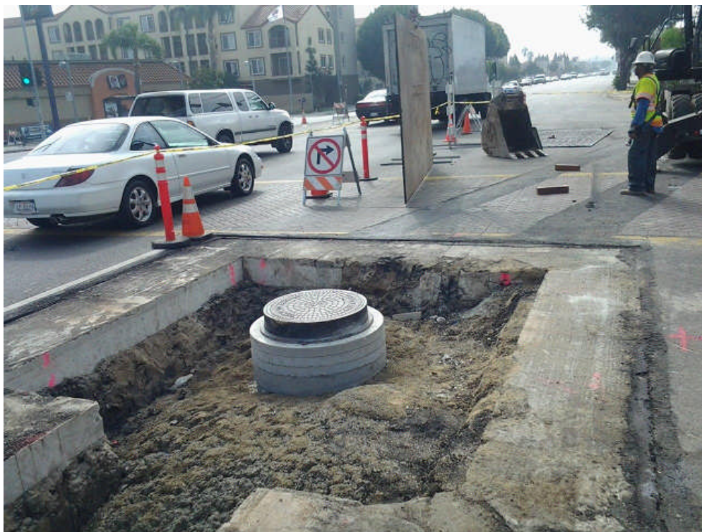
Slurry Backfill between 59 th and 60 th Street.
