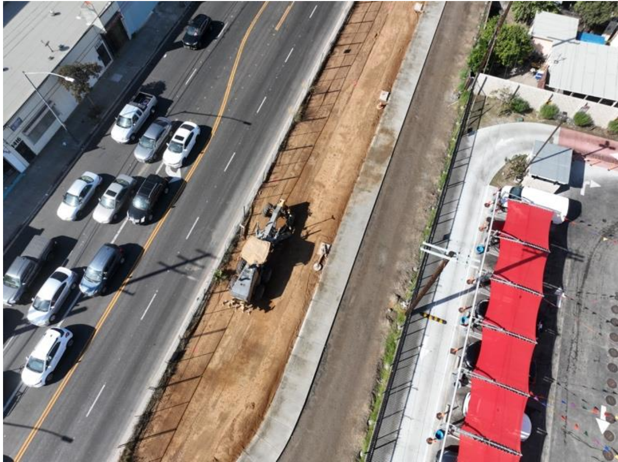
Motor grader being used to finish grade placed material southwest overview
