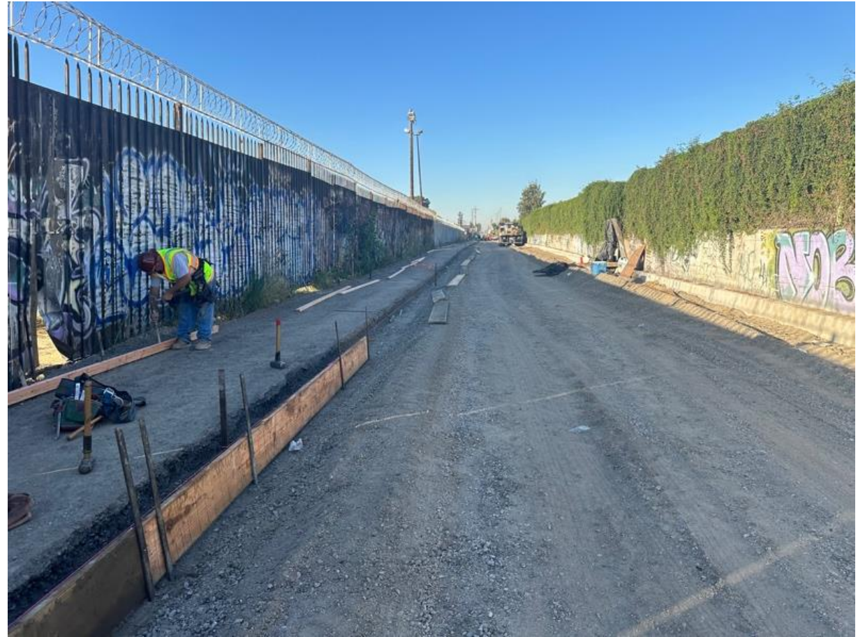
Form Placement for Pedestrian Path
