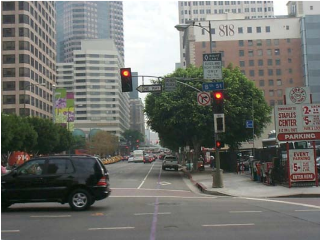
Off Peak Curb Lane Used for Parking
