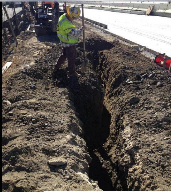
CT LIGHTING CONDUIT AT NB GETTY OFF RAMP
