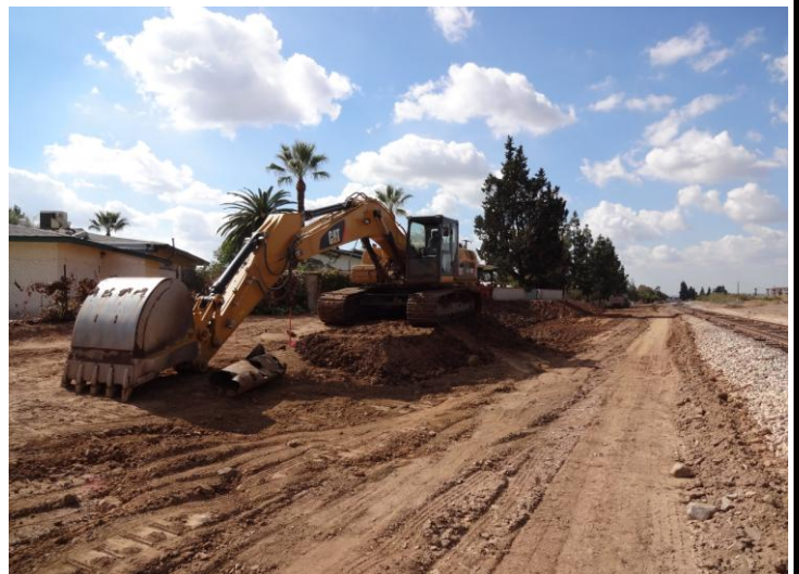
Grading work in Segment 4
