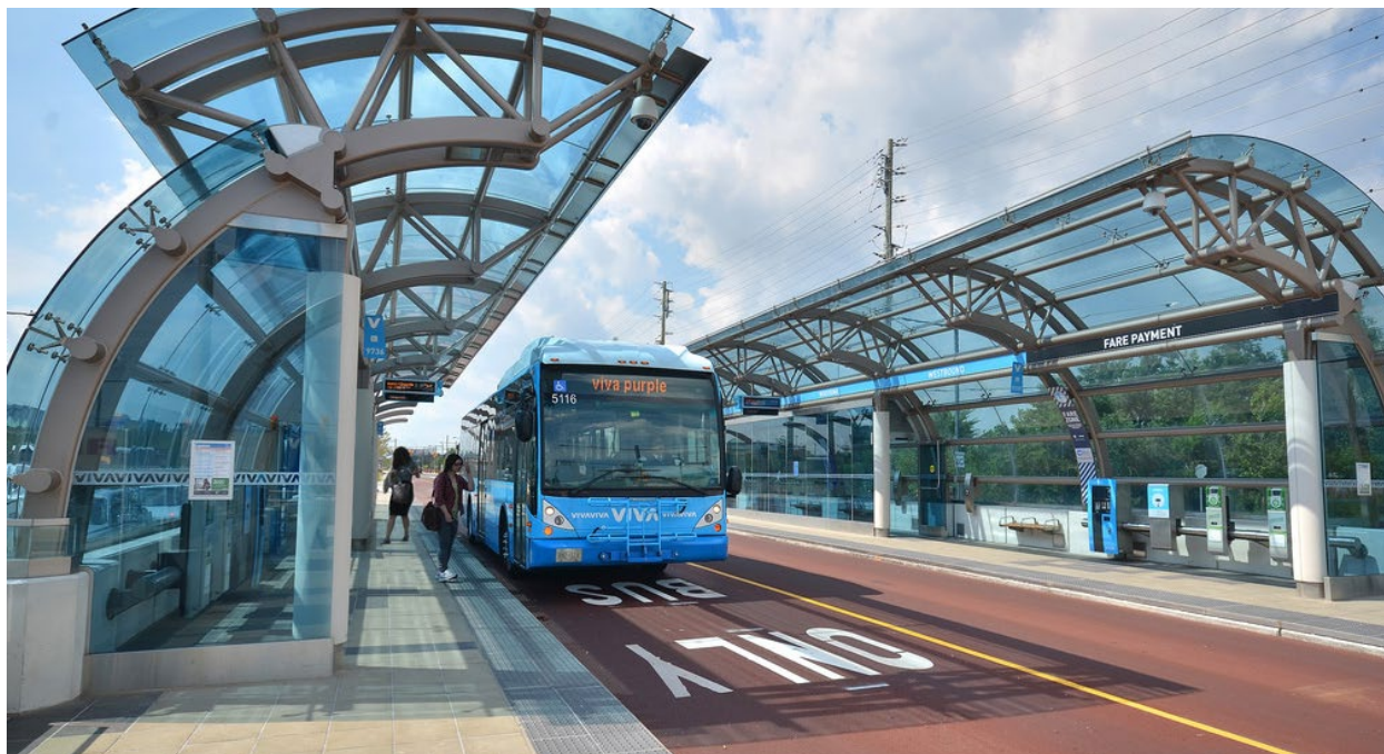
Access Control / Source: IBI Group
