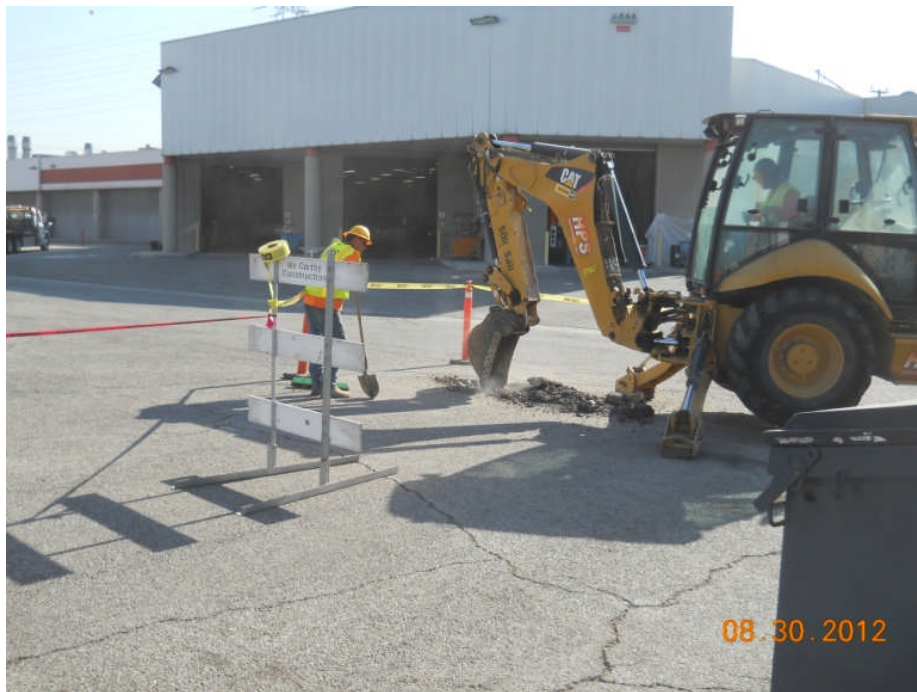
Temporary sewer facility connections.
