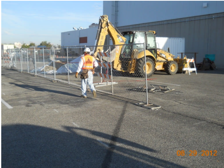
Temporary fencing being installed.
