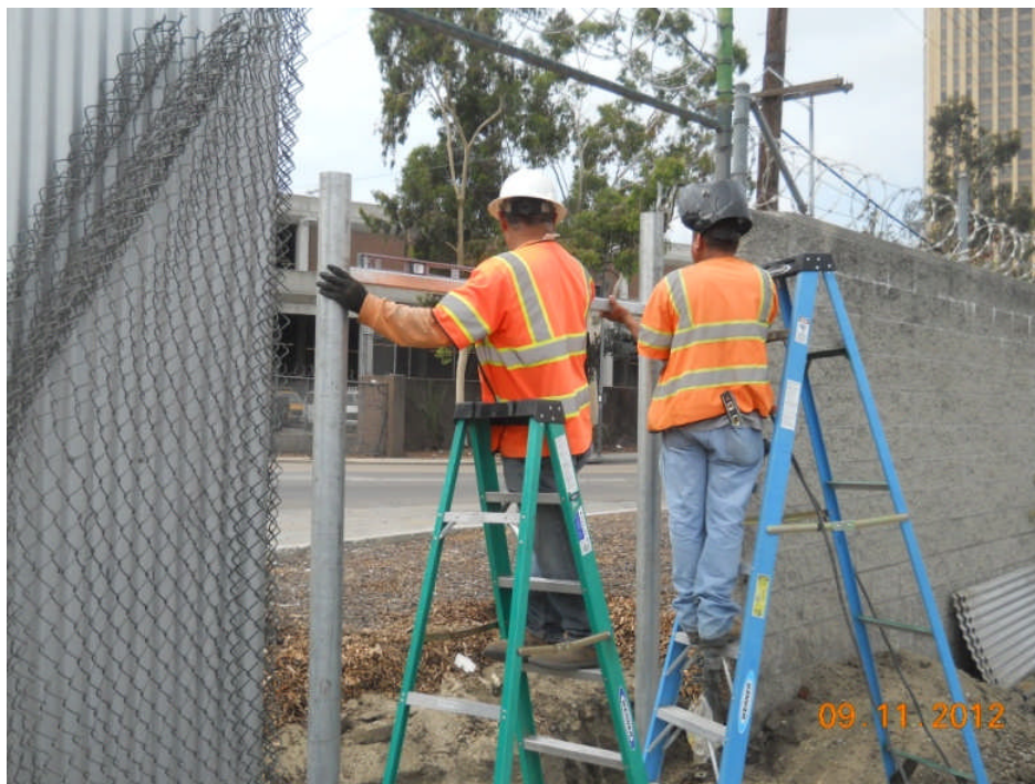
Temporary pedestrian access gate.
