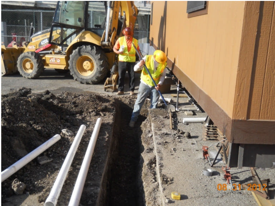
Temporary sewer facilities.
