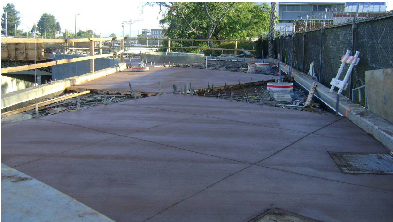
New colored concrete placed POC.
