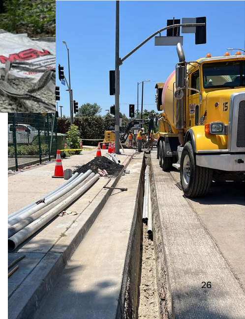
Utility Owner-Performed Advanced Utility Relocation
