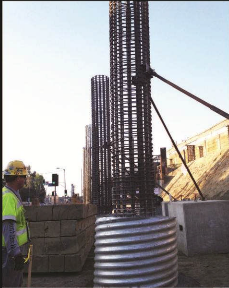
BRIDGE 17 FRAME 3 COLUMN BRACING
