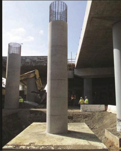
BRIDGE 2 STAGE B COLUMNS
