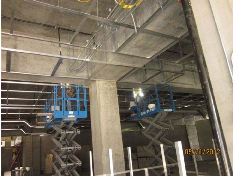
Installing metal ceiling frames.
