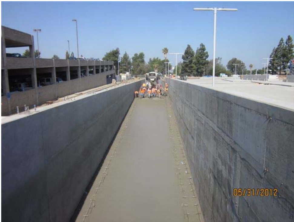
South bus ramp.
