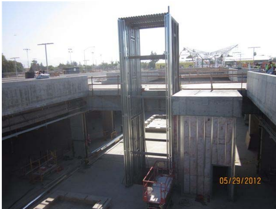
Metal framing on elevator shaft #3.
