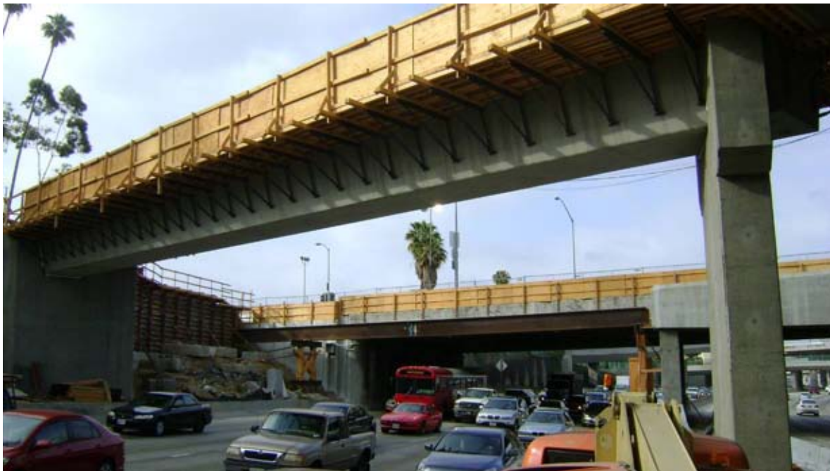
Area prepared for backfill behind POC wall.
