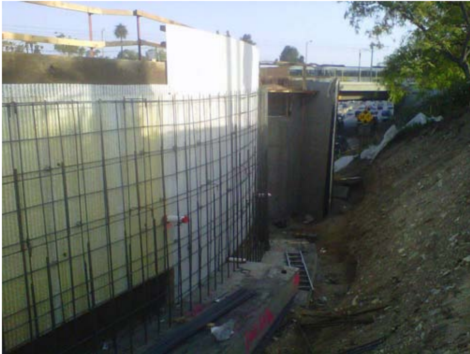
Area prepared for backfill behind POC wall.
