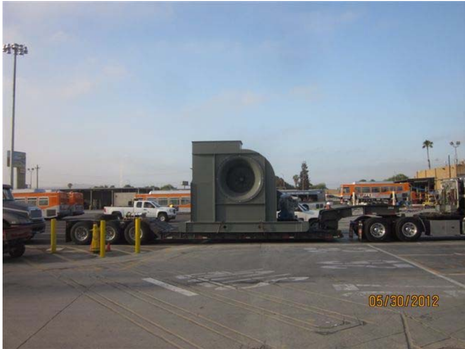
Main HVAC units on site.
