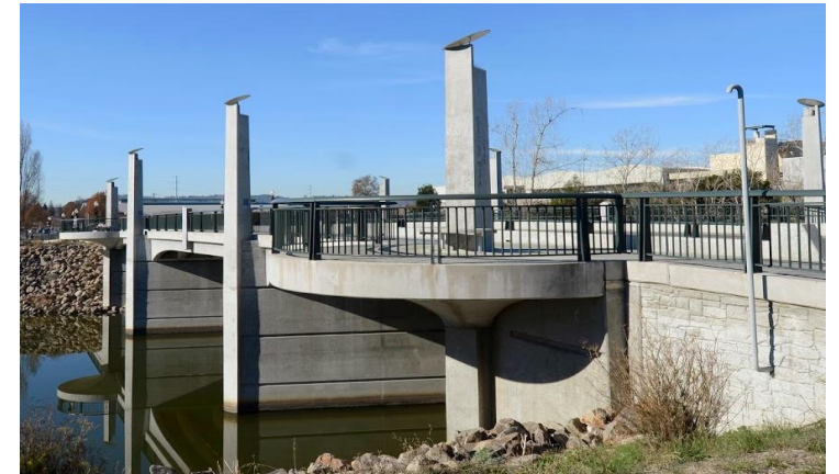
City of Napa First Street Bridge Replacement
