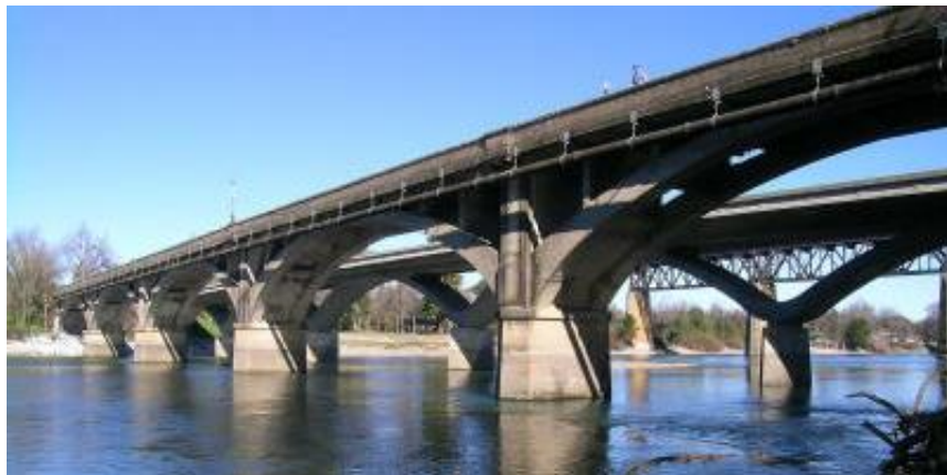
City of Redding historic Diestelhorst bridge replacement with Benton Drive (now is a pedestrian bridge)
