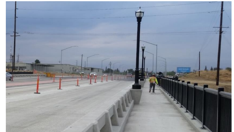
City of Reedley E. Manning Road Bridge Replacement - Fresno County
