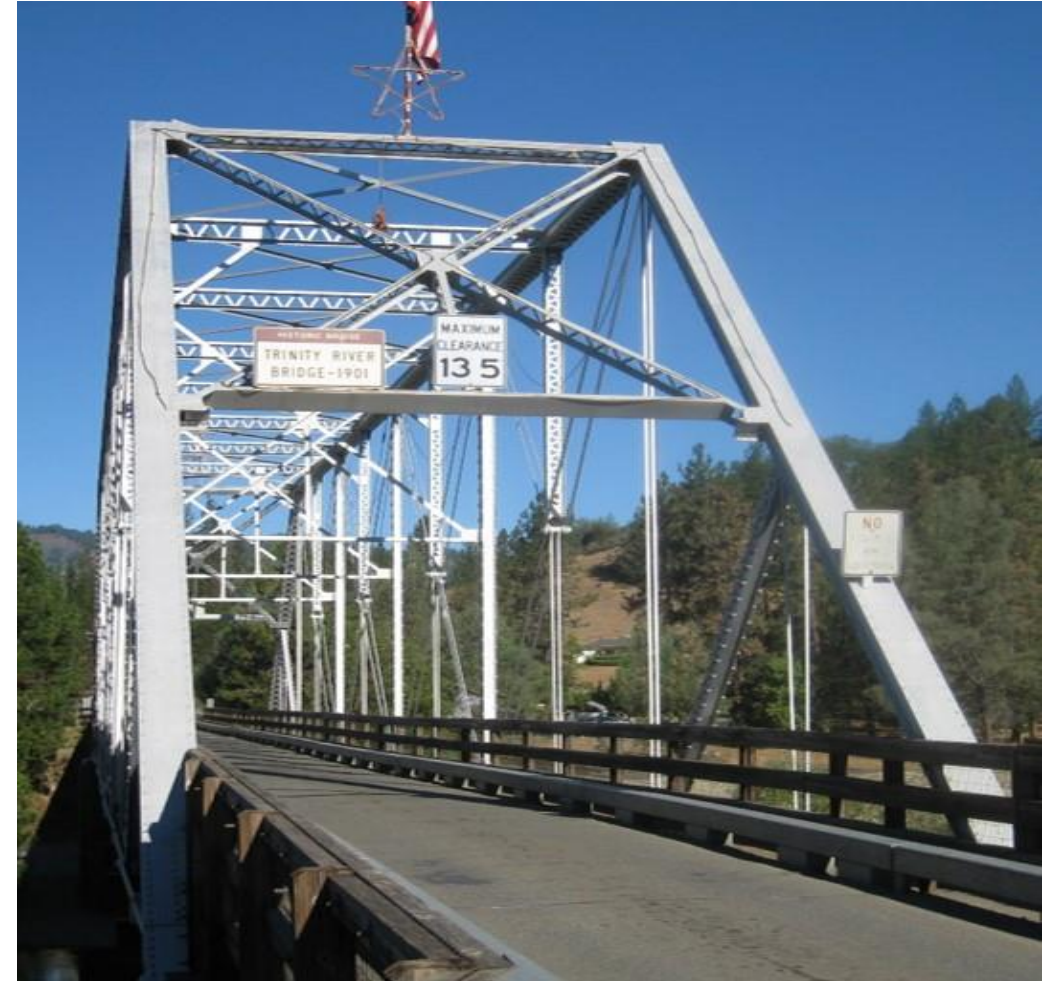
Trinity County Turnpike Road Bridge Painting
