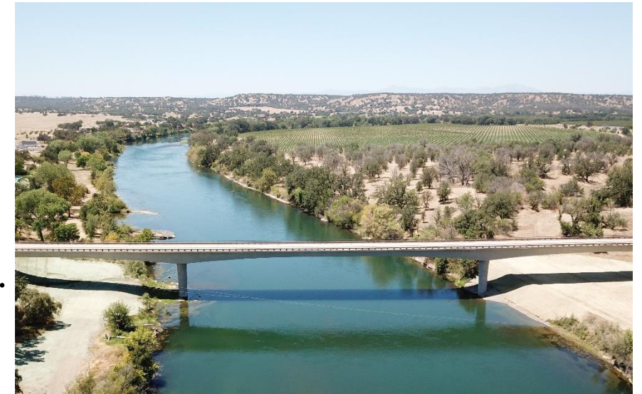
Tehama County Jellys Ferry Bridge Replacement
