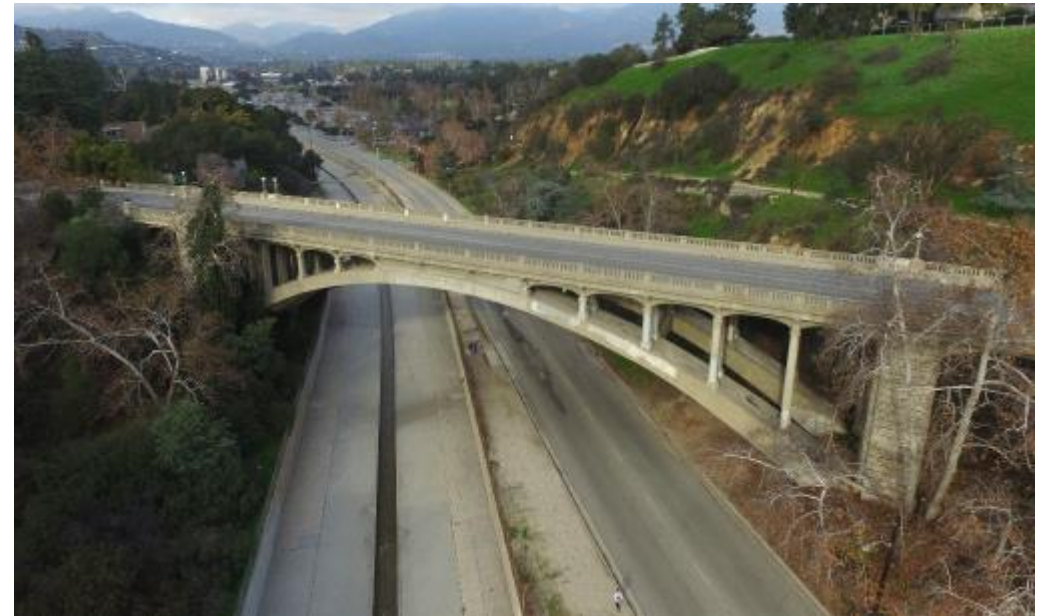
Holly Street Bridge 53C1041
