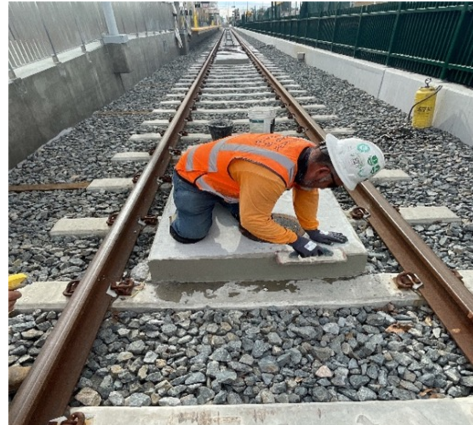
Sacking and patching rail vehicle pads along southbound track
