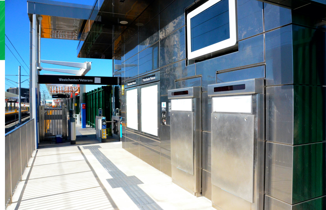
Platform entrance and Ticket Vending Machine
