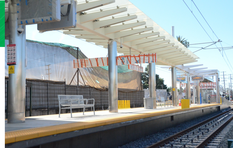
Station platform, benches, and bollards
