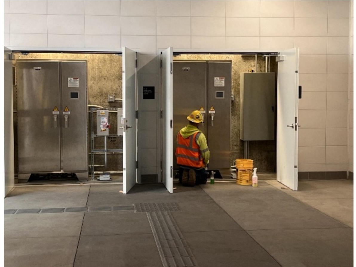
Cleaning escalator controller cabinets at the concourse level.
