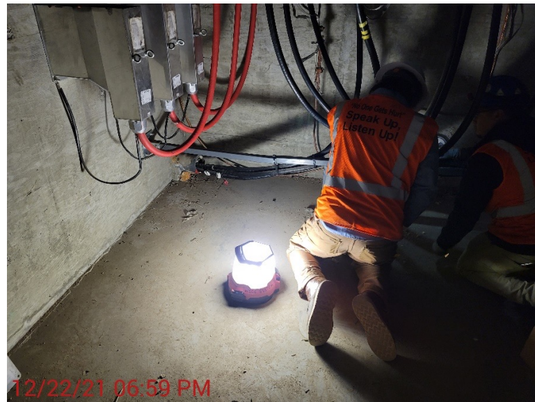
Remaining items Remedial work for TPSS #2 Vault
