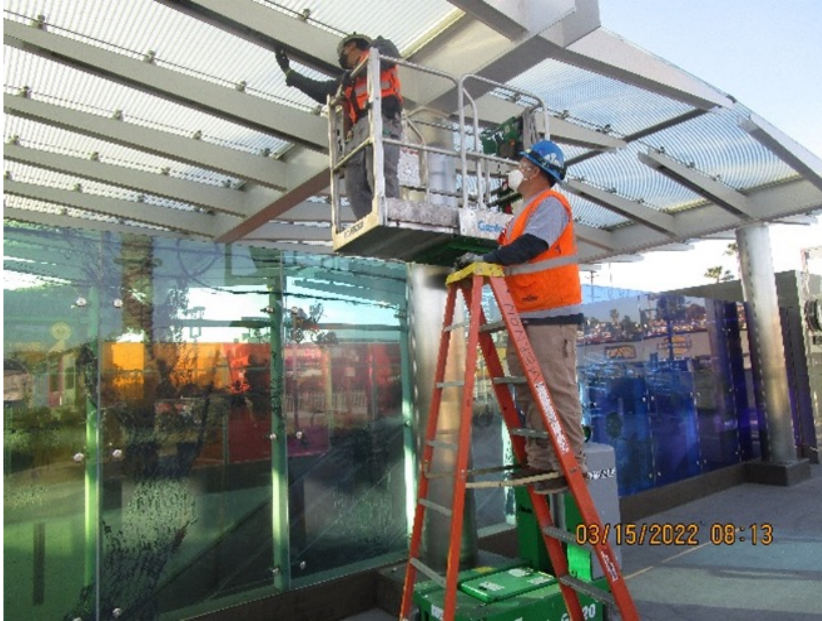
Adjustment of wires for lighting at the main entrance plaza canopy.
