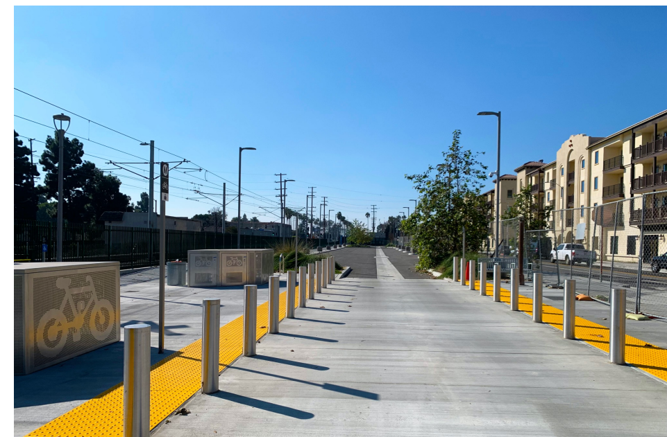
Station parking lot looking west
