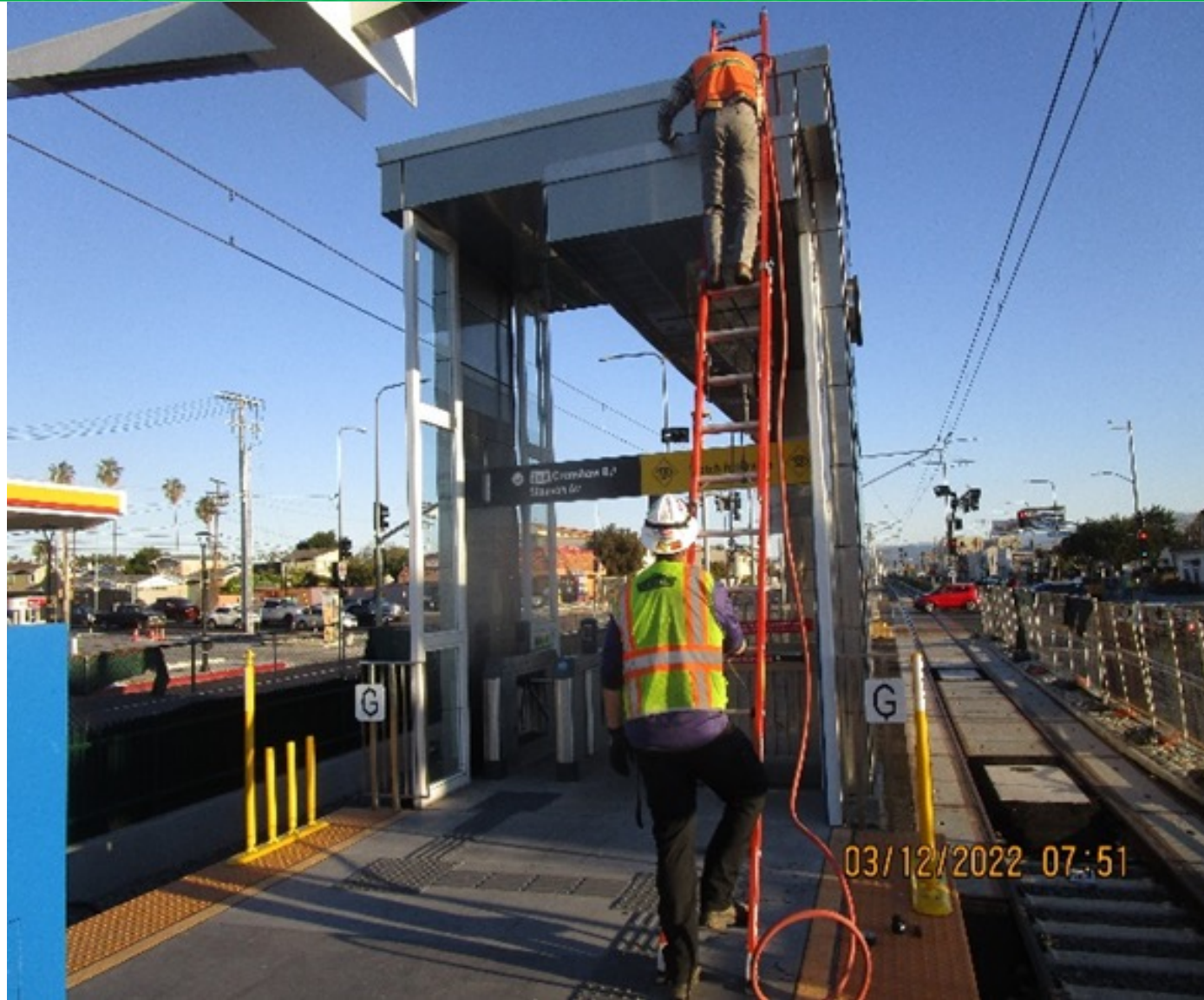
Water pressure testing for the roof drains at the south pavilion
