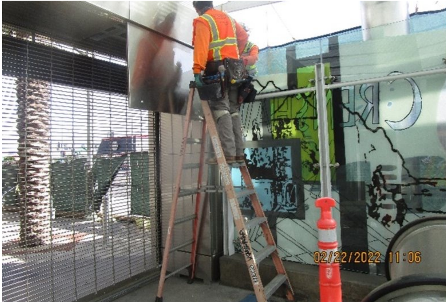
Adjusting stainless steel cladding panels at the main entrance plaza level.
