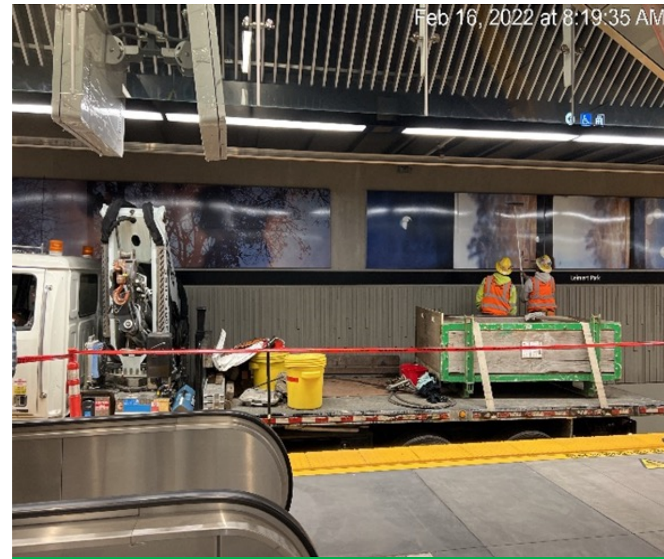
Cleaning of art panels along the Leimert Park Station platform.
