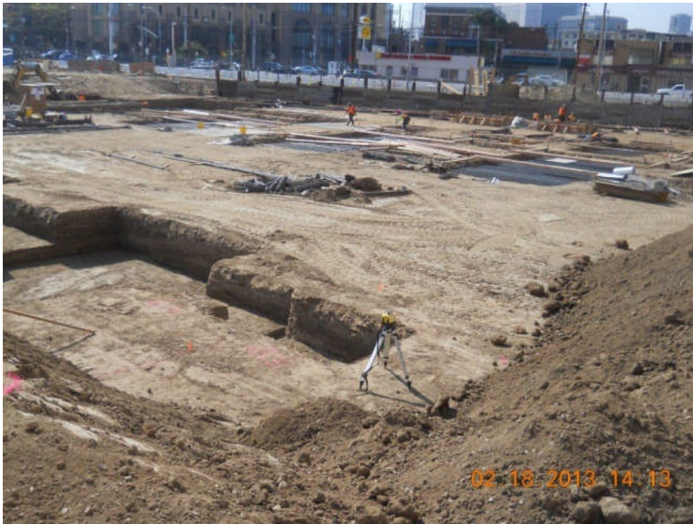
Foundations at Administration Building.
