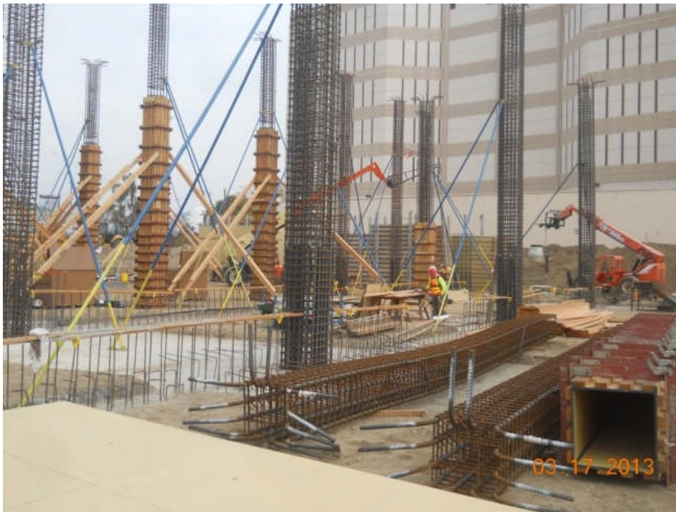
Column formwork at Parking Garage Building.
