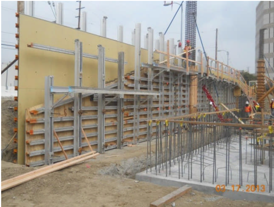
Wall formwork at Administration Building.
