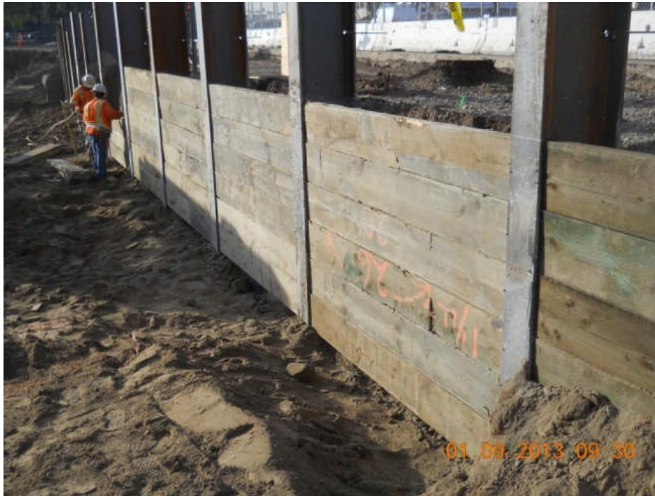
Shoring at Vignes Street.
