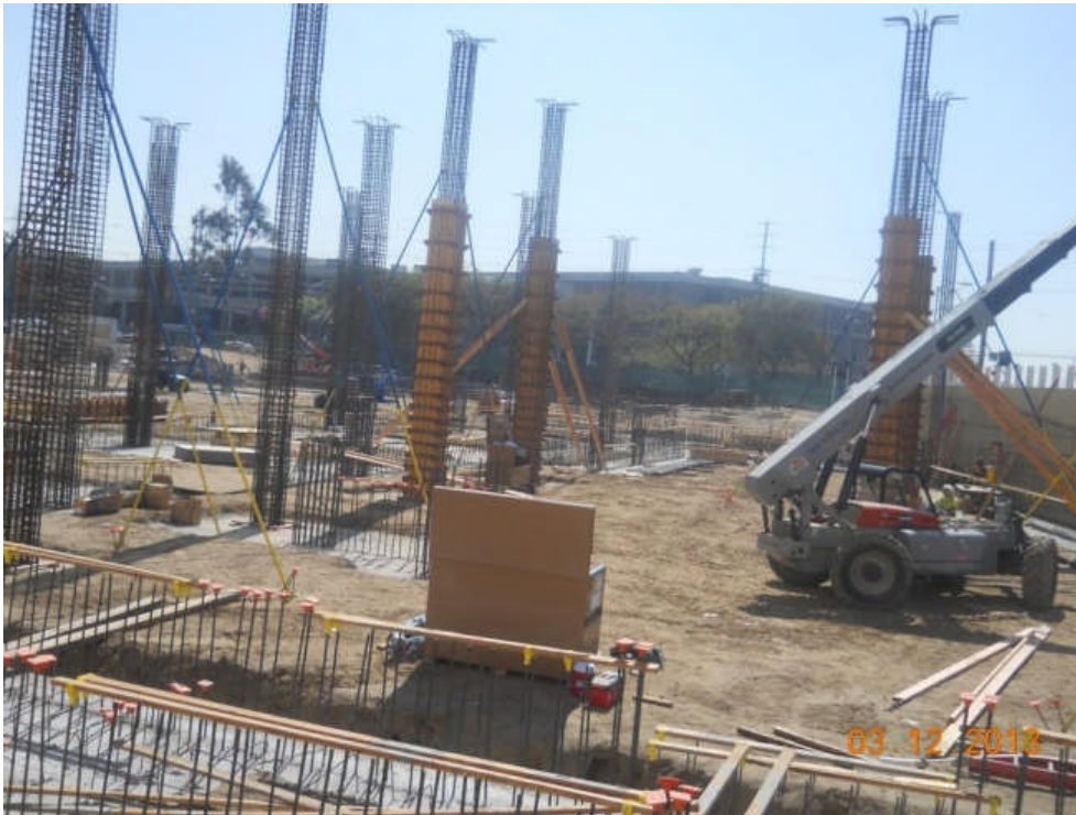
Concrete formwork at Parking Garage Building.
