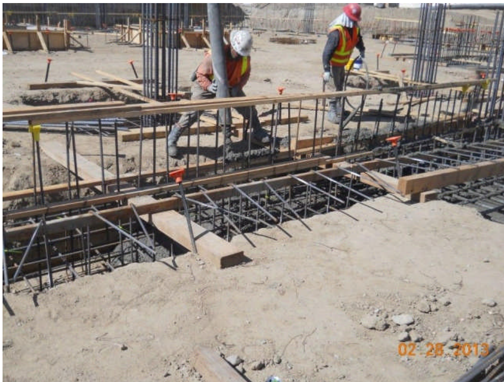
Concrete placement at Parking Garage Building.
