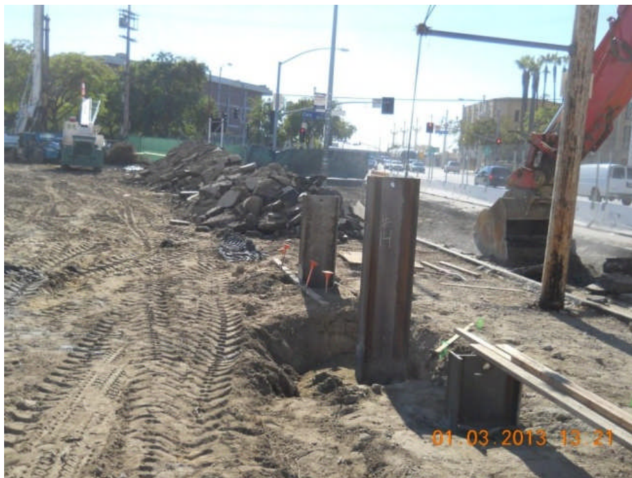
Shoring installation at Vignes Street.
