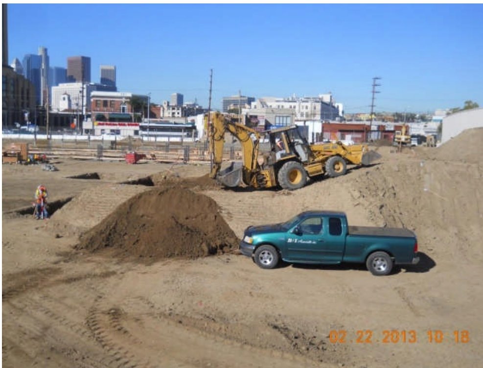
Foundation excavation at Parking Garage,
