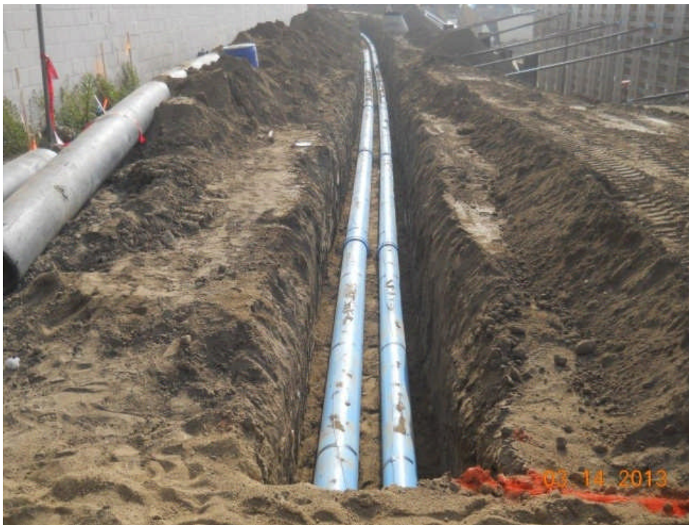
Underground utilities at Metro Drive.
