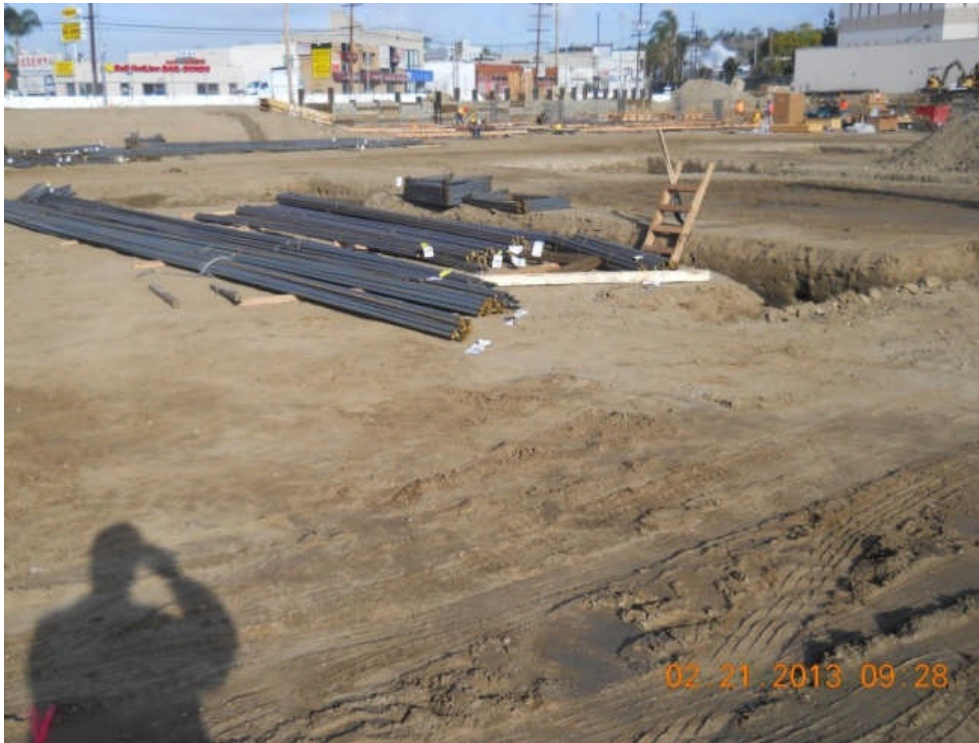
Concrete reinforcement at Parking Garage.
