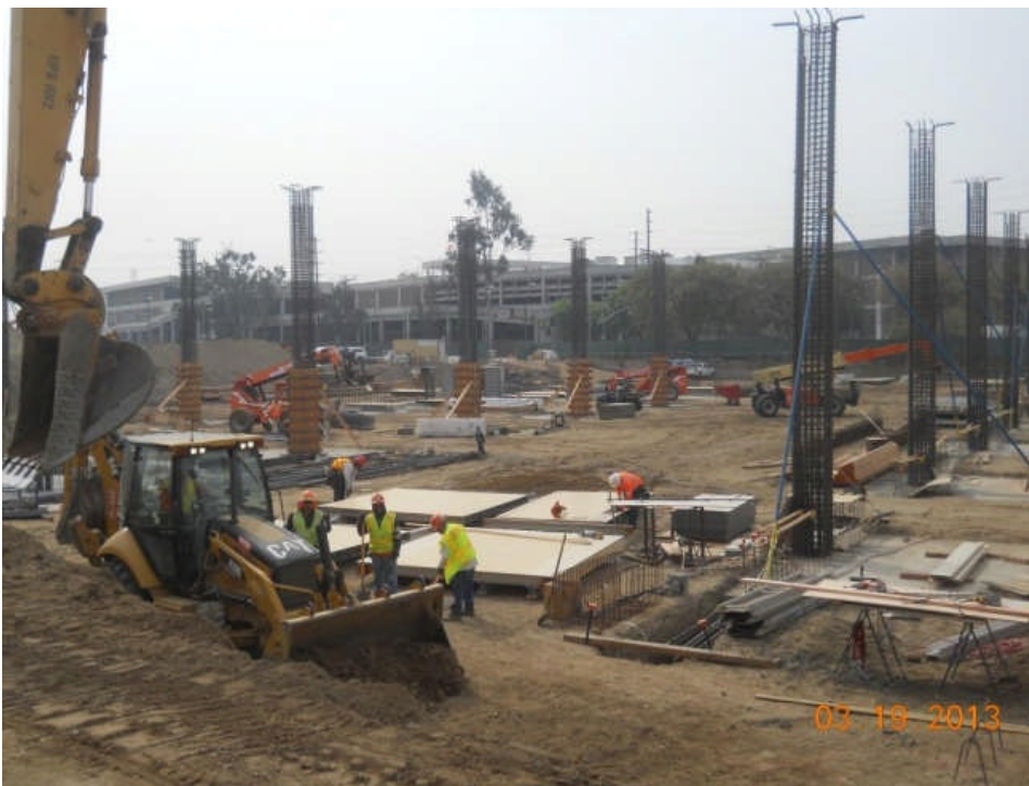
Column formwork at Parking Garage Building.
