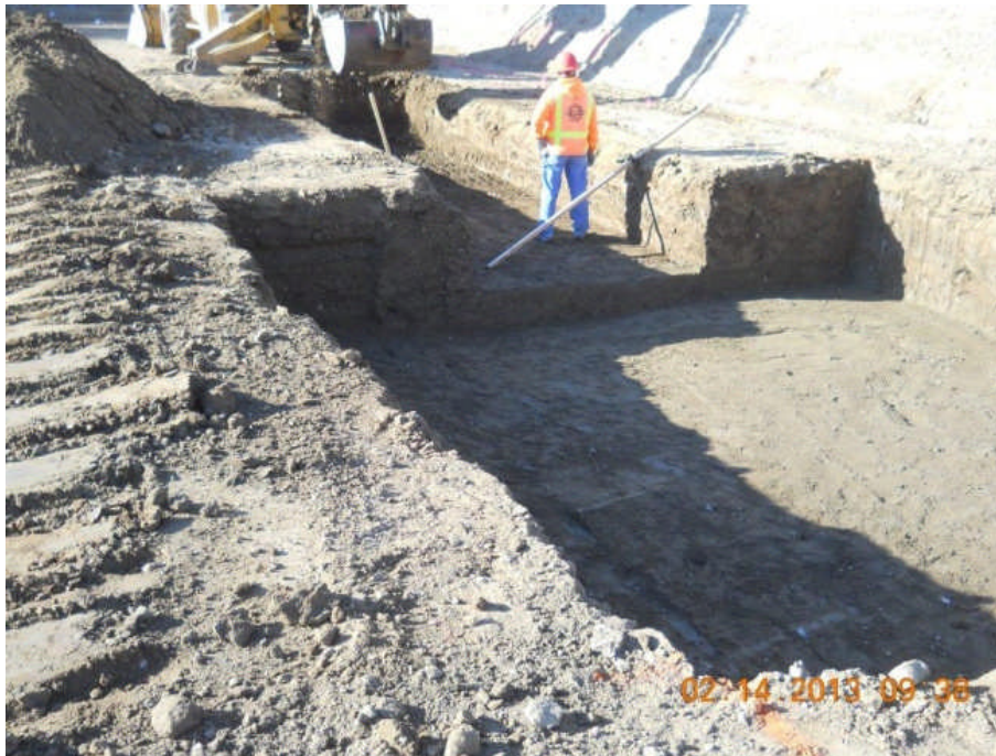
Footing excavation at Administration Building.
