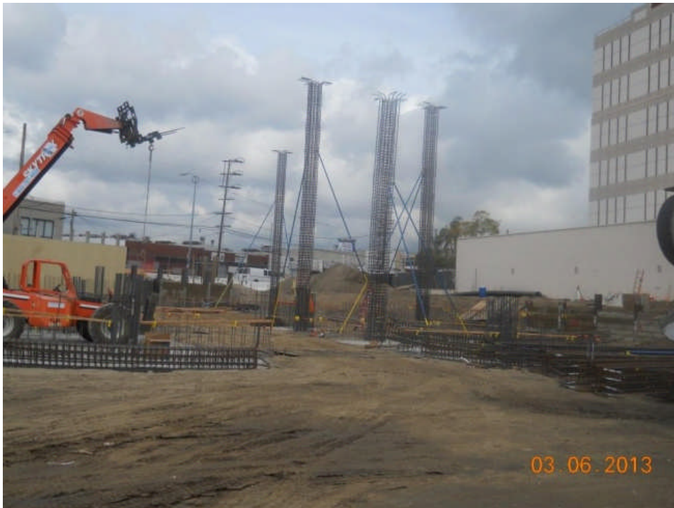
Concrete reinforcement of columns.
