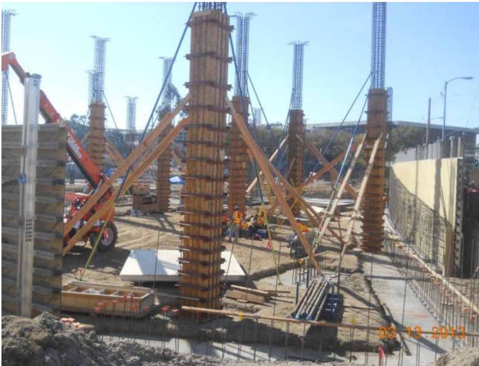
Concrete formwork at Administration Building.
