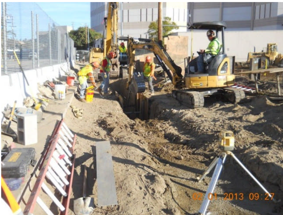
Utility trenching at Vignes Street.
