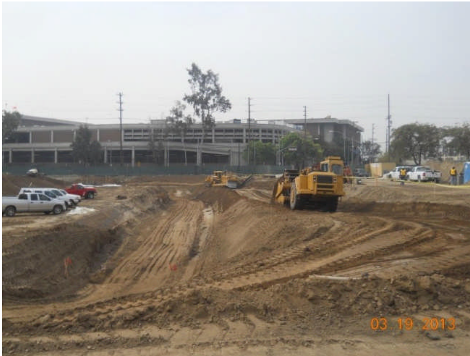
Mass grading at east Parking Garage Building.
