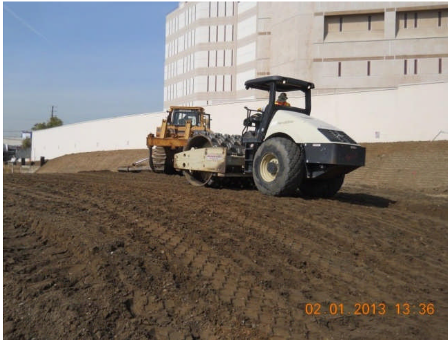
Grading and compaction on site.
