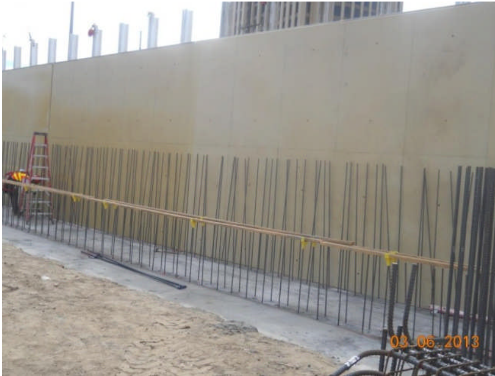
Formwork for cast-in-place concrete walls.
