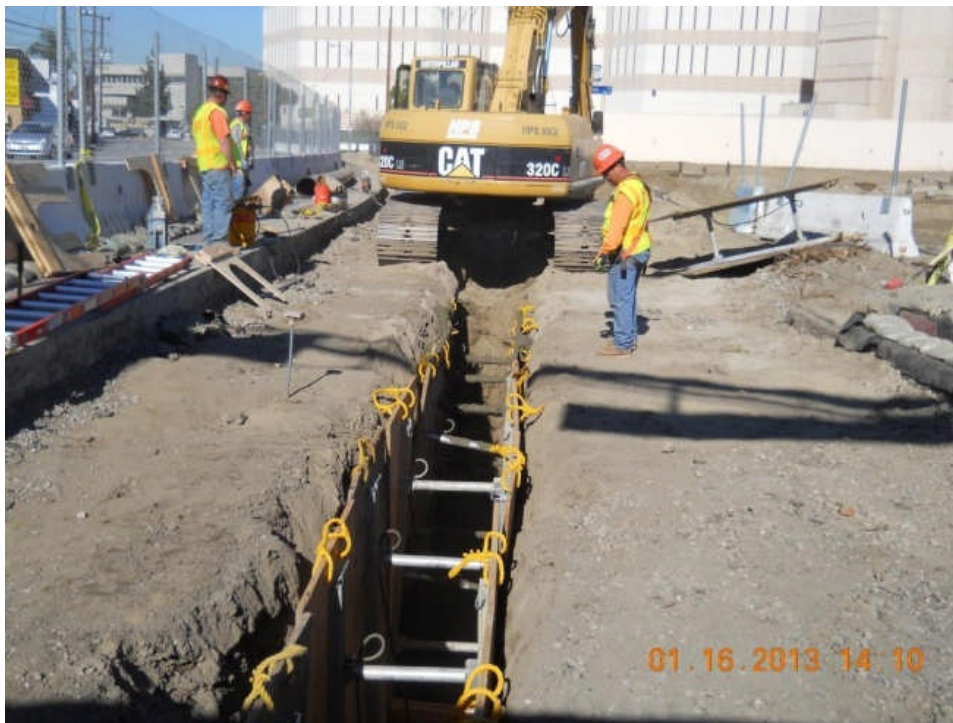
Utility excavation at Vignes Street.
