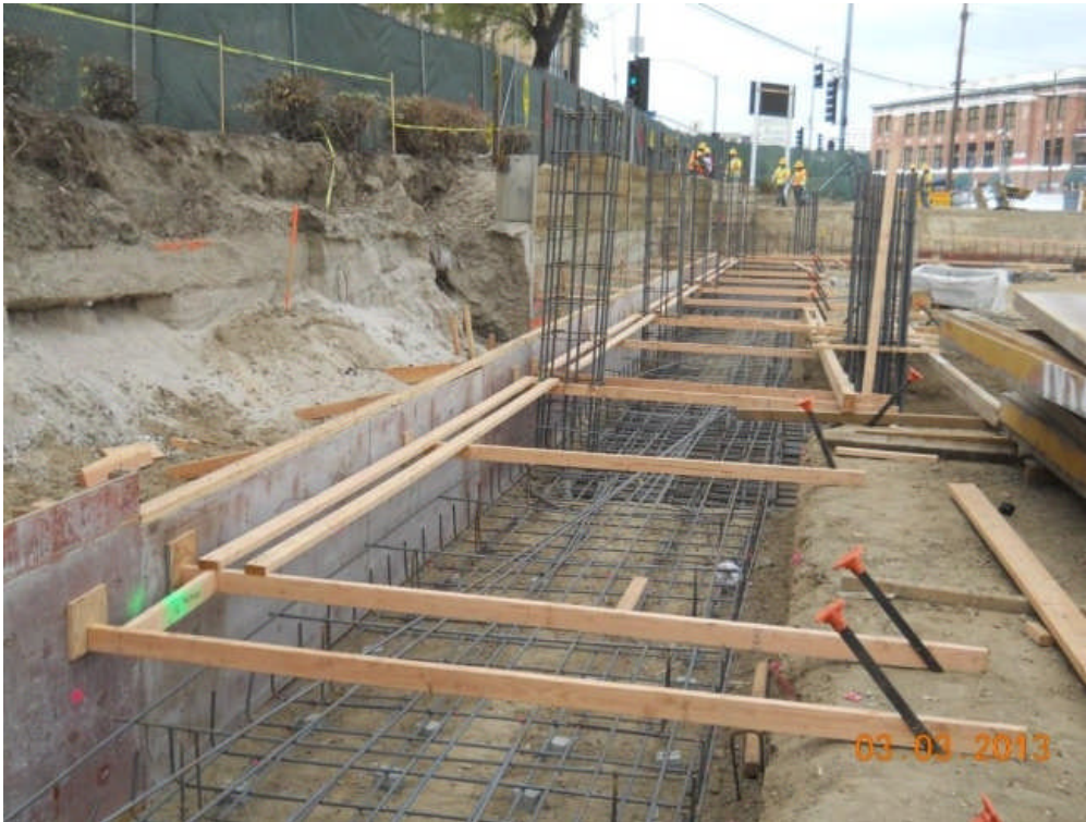
Foundation formwork at Parking Garage.
