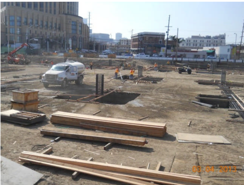
Foundation formwork at Parking Garage.
