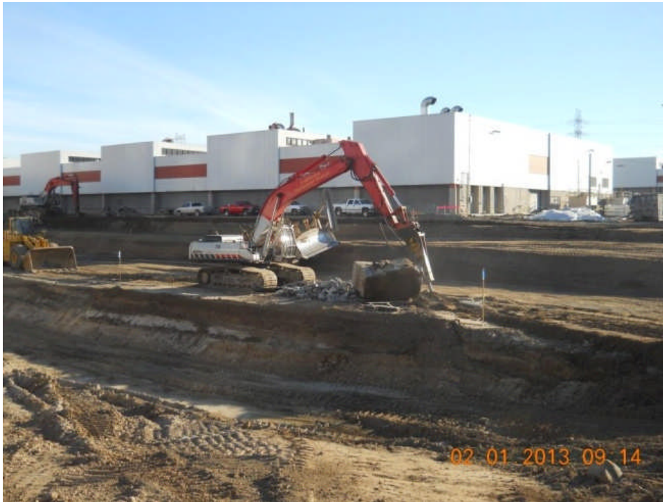
Earthwork and removal of obstructions.
