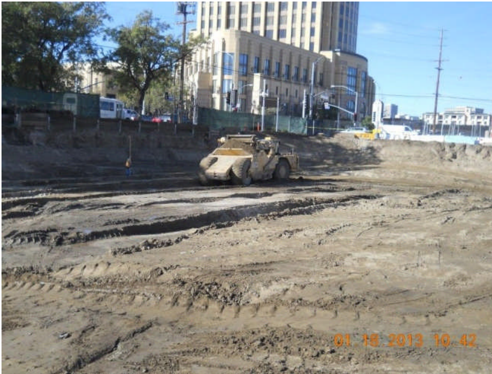
Mass grading at south Parking Garage Building.
