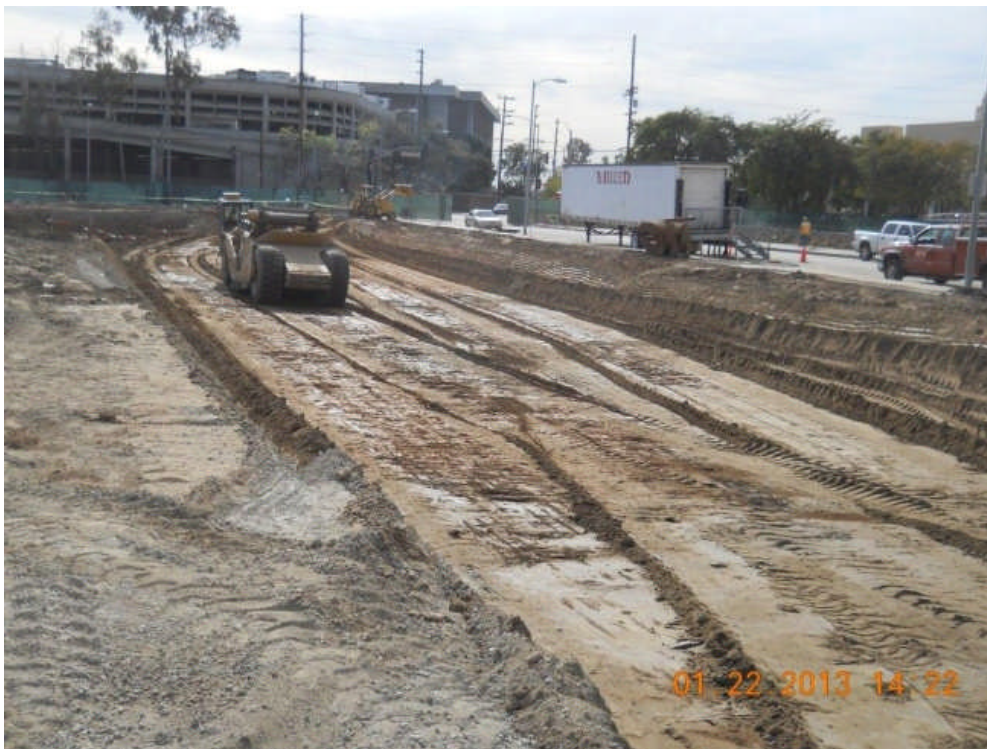
Mass grading at east Parking Garage Building.
