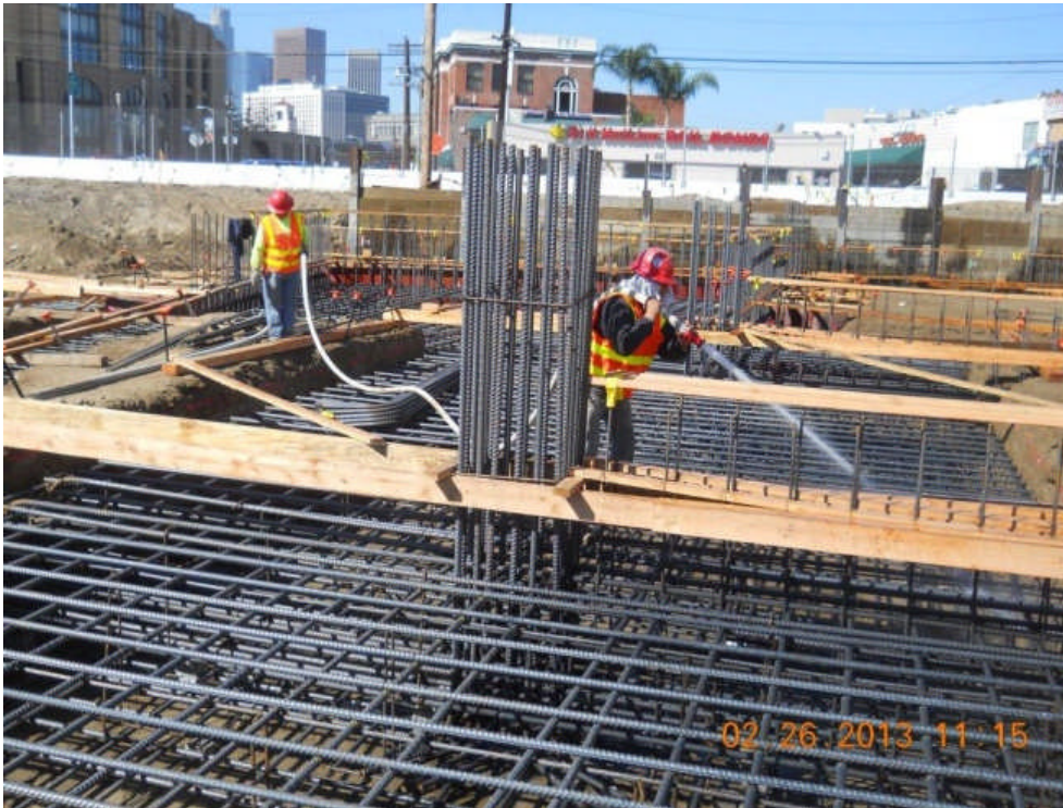
Foundation reinforcement at Administration Building.
