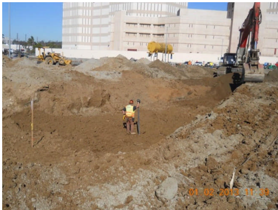
Earthwork at east side of Lyon Street.
