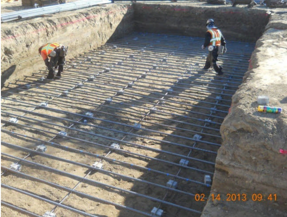
Foundation reinforcement at Administration Building.
