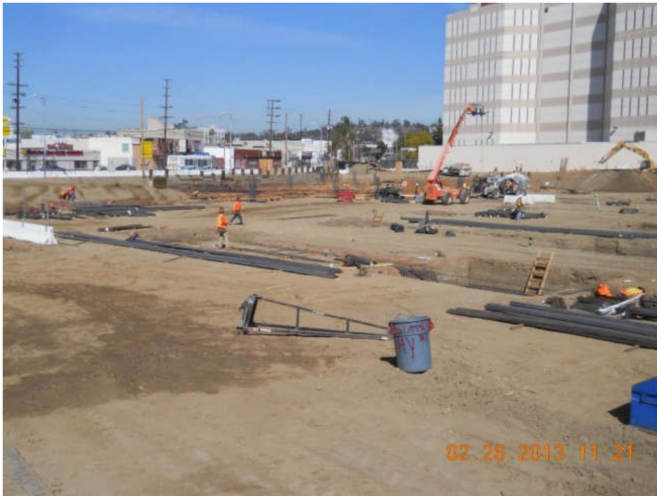
Foundation excavation at Parking Garage.
