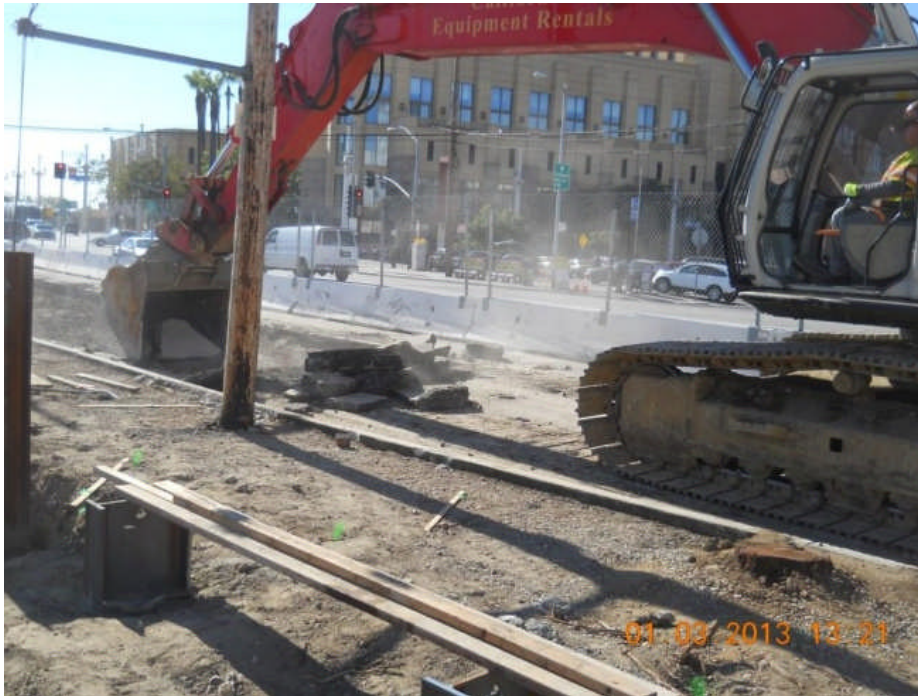
AC pavement demolition at Vignes Street.
