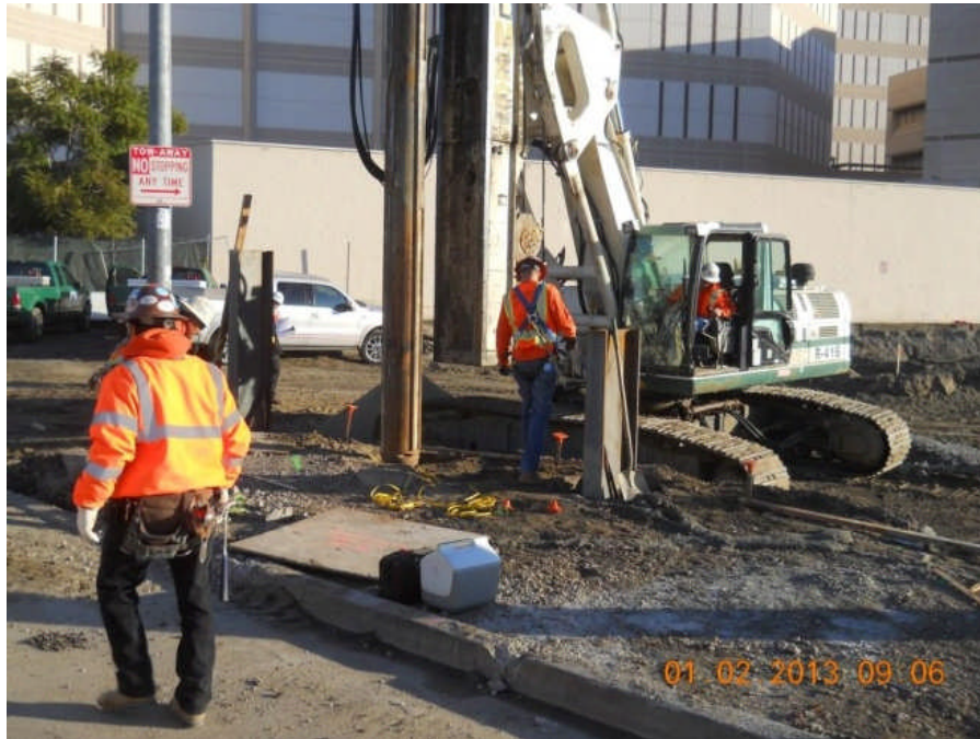
Shoring installation at Vignes Street.
