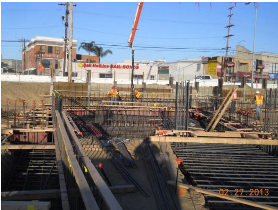
Foundations at Parking Garage Building.
