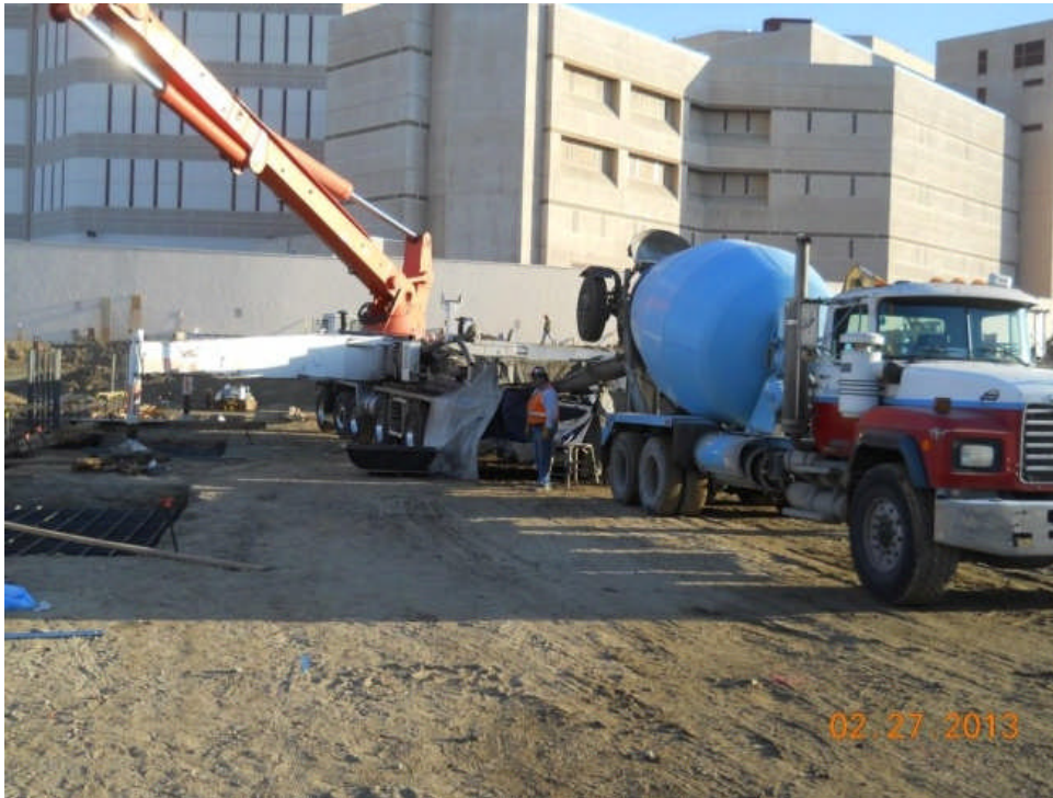
First concrete placement at Administration Building.
